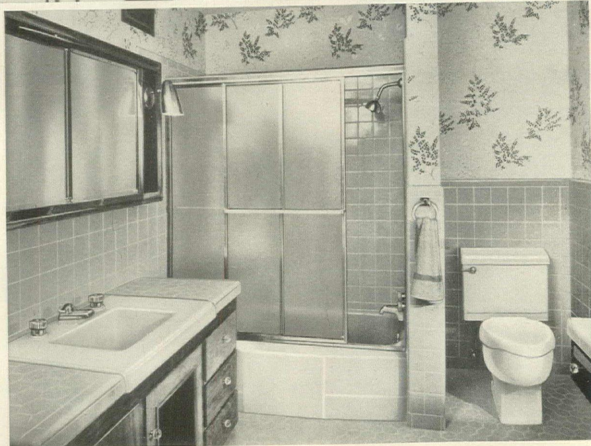
Crane Fixtures were used in exhibit homes at all price levels. This Crane Criterion bathroom ensemble was featured in one of the Wichita homes in the $14-20,000 class. It made a big hit.
