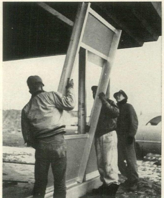
Two men position 85-lb. panel between top and bottom rails. Finished construction indicates variety of designs possible.
