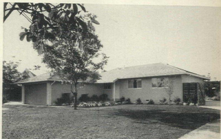
Two hip-roof houses, both based on plan at left, demonstrate choices offered. Cedar shakes are new lure.
