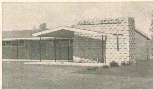
Concrete masonry constructed church school. Note the unusual effect created by alternately protruding block.
