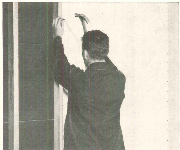
INSULATION BOARD PANELS ...NOW sell more fast, low-cost remodeling jobs with Gold Bond Insulation Panels. Flame-resistant Ivory coating saves painting. Fast handling; easy to cut. Bevel or cover joints with moulding.
