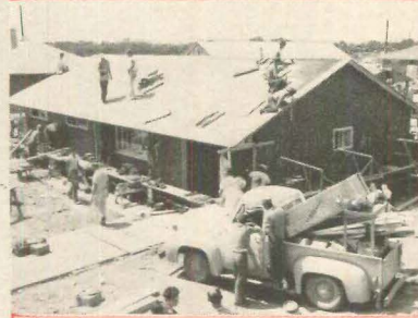
3:39 P.M. Roof nearly finished, bricklayers at work
