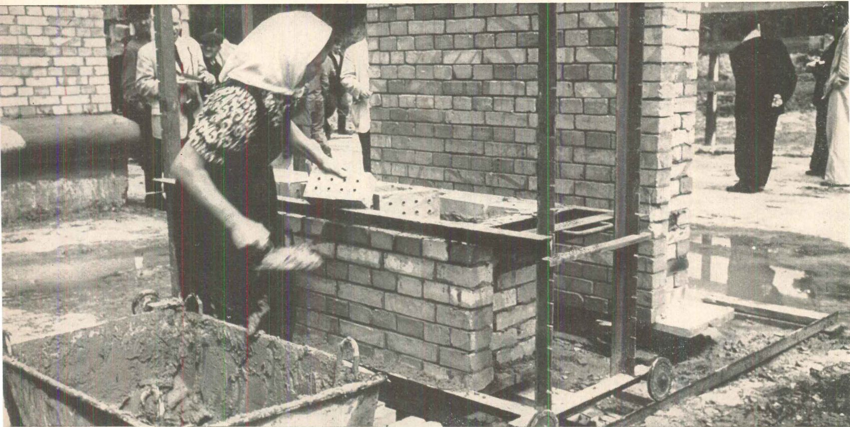
Women do most construction work. This one makes prefabricated apartment house walls (like one at rear). Relatively unskilled, her work is kept accurate by steel jig which rolls on track as sections are finished.
