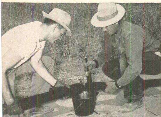
Connections for plastic pipe can be made simply with a solvent "weld". No threading vise or dies are needed.
