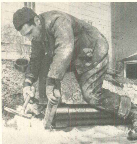
Joints are quickly and easily made by simply tapping together—no cement, no calking.
