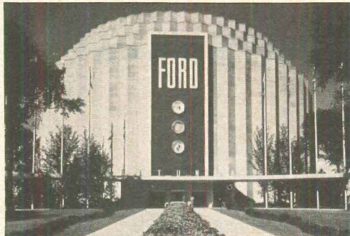
Lightweight block were selected in the construction of the beautiful Ford Rotunda at Dearborn, Michigan.
