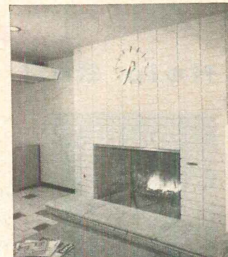
(left) Exposed concrete block in stacked bond adds charm to this residential fireplace.
