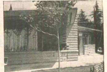
(right) Frank Lloyd Wright designed this beautiful concrete masonry home, using standard 4" high block.
