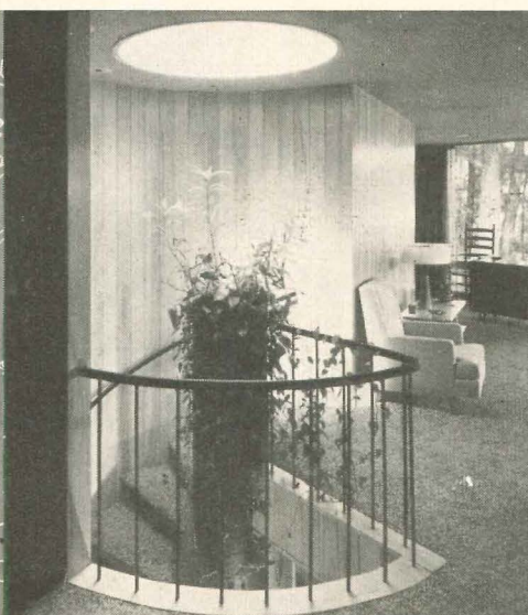
Circular staircase is at center of house, lighted from above by a (5' dia.) plastic dome. Pinpoint spots ring the dome for night lighting.
