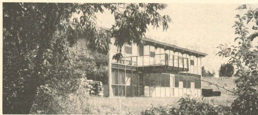
Cantilevered balcony gives upper level of hillside house a 100 sq. ft. deck outdoors. This glassy facade faces south, works well even during harsh Vermont winters.
