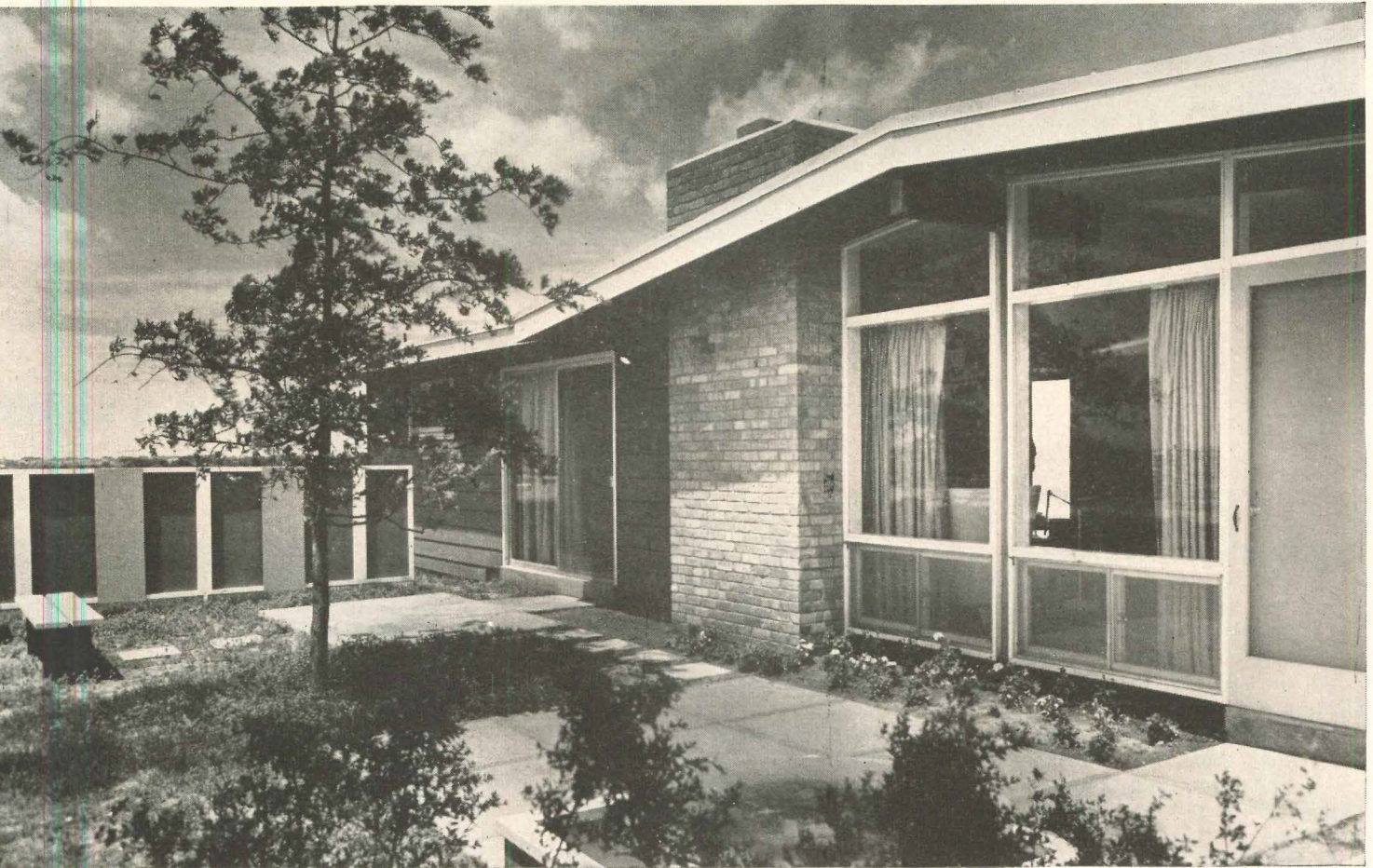
Big terrace behind house is Kemp extra. Others are floor to ceiling windows, post-and-beam construction, privacy fences.
