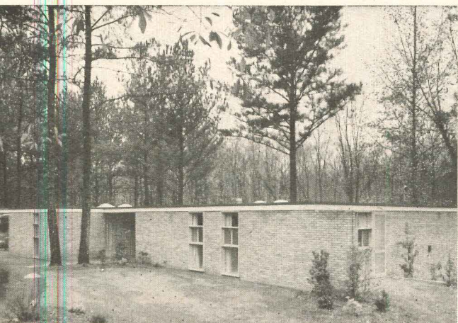
Street side house preserves its privacy, gives little indication of its openness. White domes on roof are plastic skylights.
