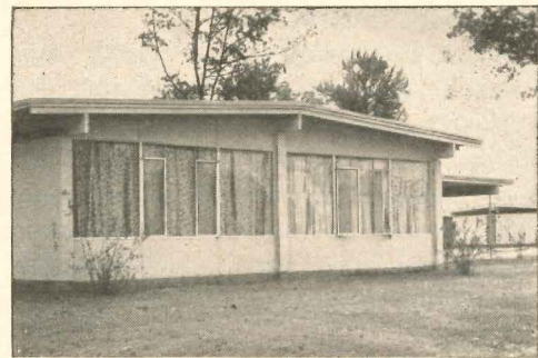
Entire rear wall is filled with windows prefabricated in six floor-to-sloping roof sections. Cemesto replaces glass at bottom.
