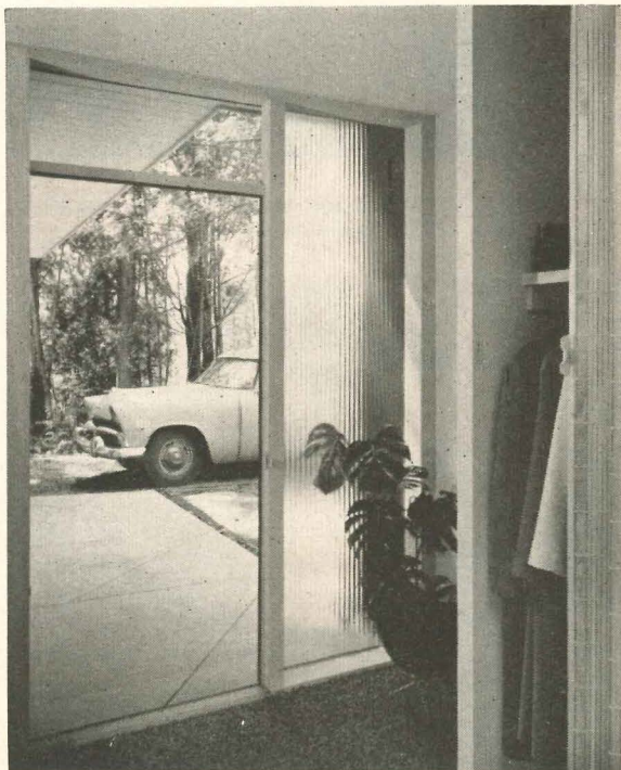
Front entrance is shielded against rain outside, has obscure glass around it for light with privacy. Coat closet is behind accordion door at right.
