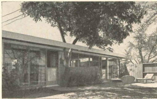
Rear patio serves as play yard. Kitchen has "Dutch" door made by cutting stock door in half.
