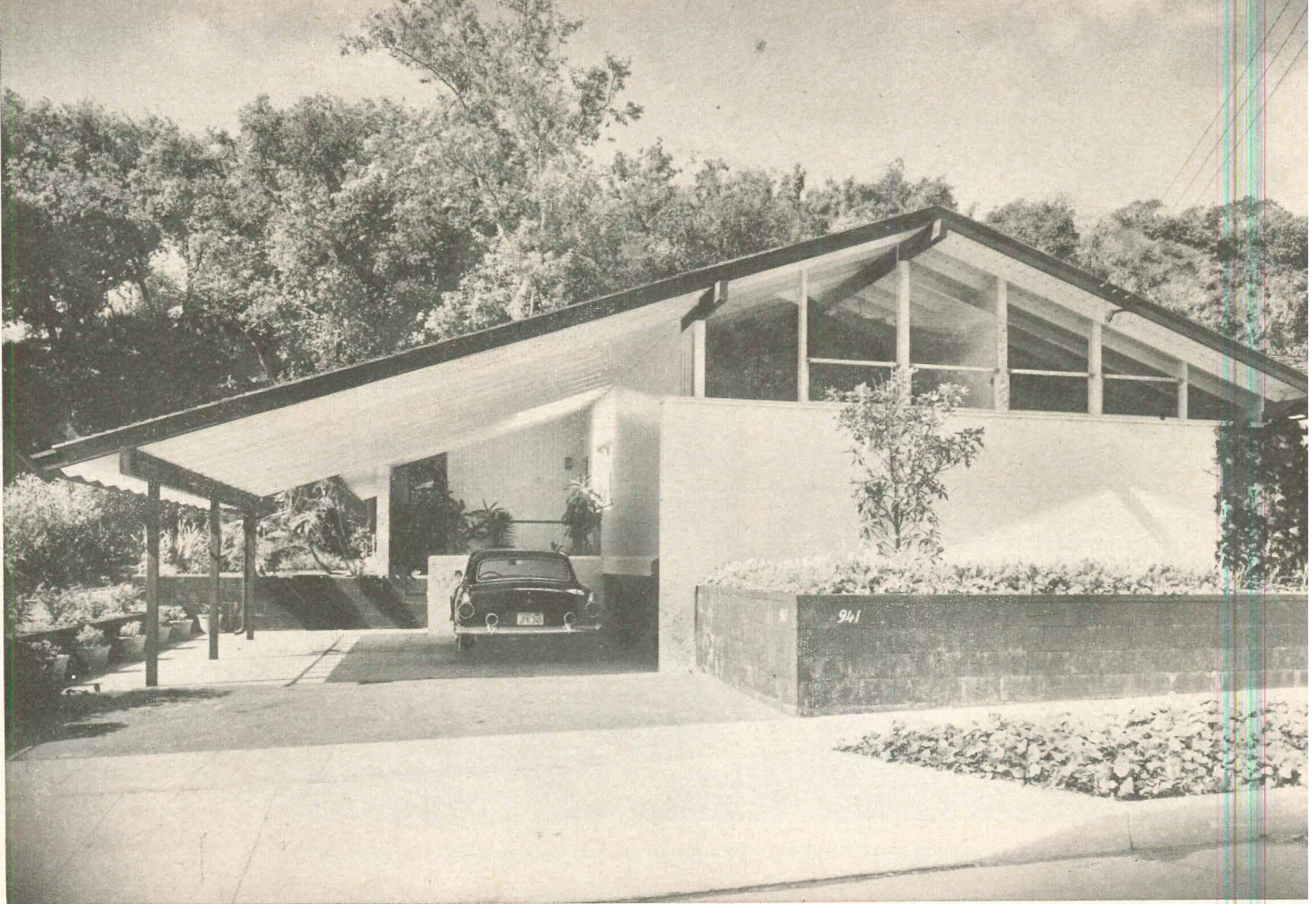
From the street, the wide pitched roof ties the carport in with the rest of the house. Carports are 2'-3' below floor level of house.
