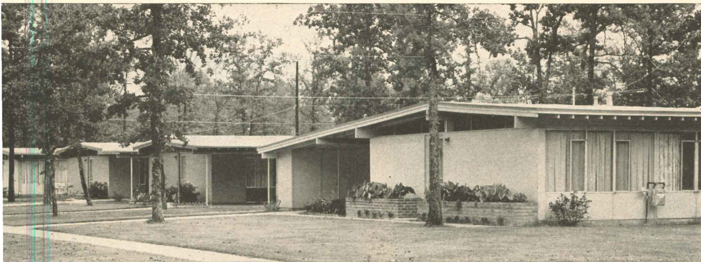
Entire rear wall is filled with windows prefabricated in six floor-to-sloping roof sections. Cemesto replaces glass at bottom.
