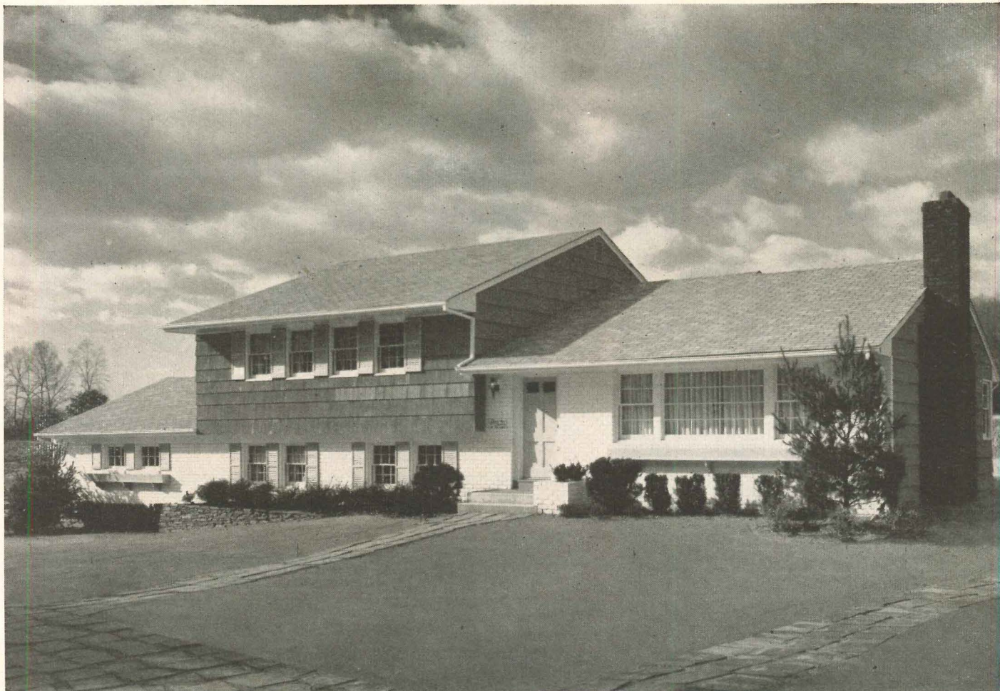
Front of house shows pleasant blend of white brick, shingles, and gaily painted shutters. Sloping site lent itself to good split level construction; the front door is on grade, while the lower living area is fully exposed to sunlight.
