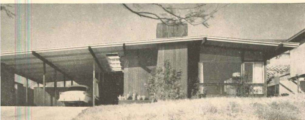
1,650 sq. ft. house sold for $24,500. Builder plans to put up more. Fireplace and patent flue are housed in redwood-covered stack at center of facade.
