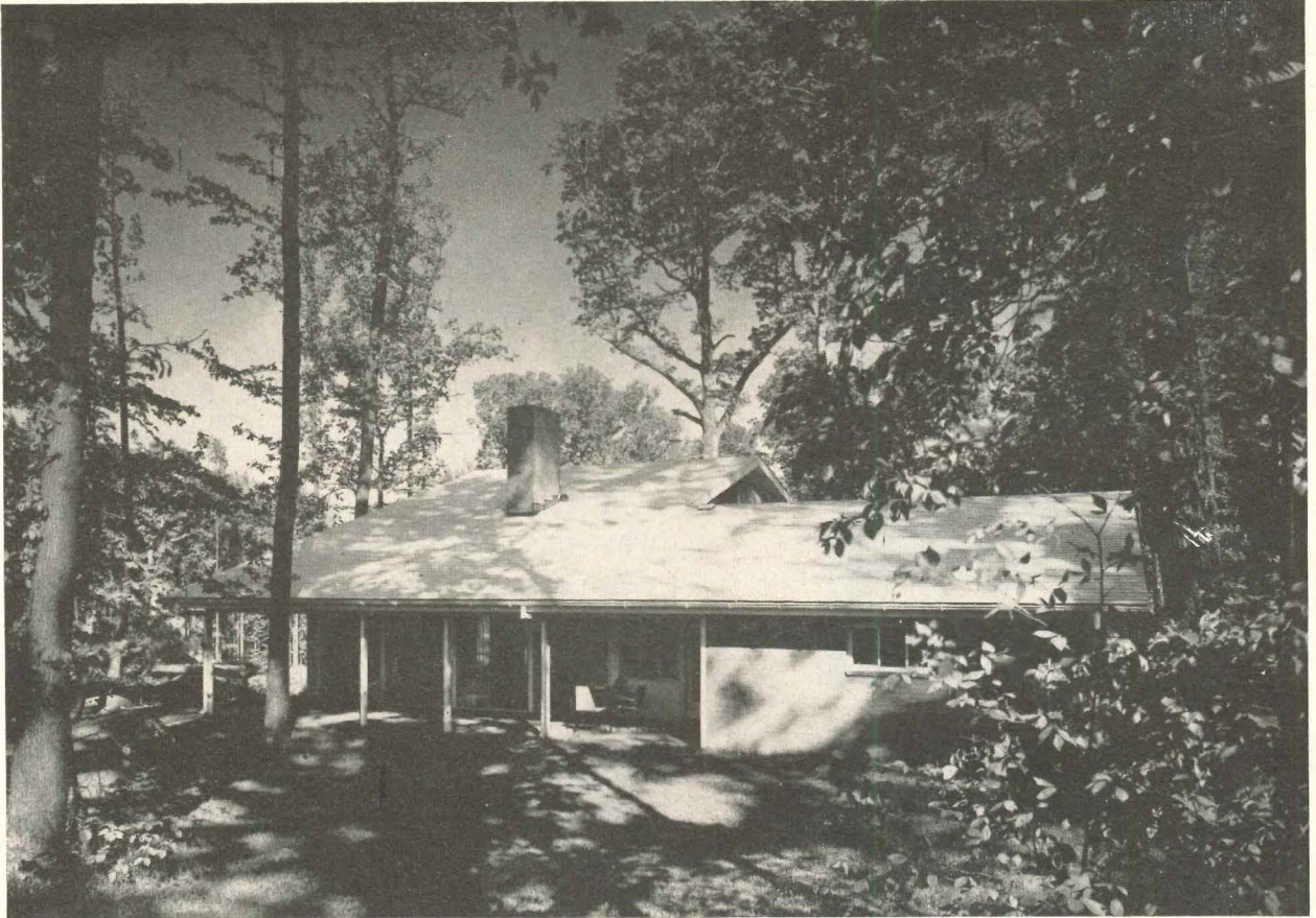
One-story side looks low because big roof slopes out over terrace, with roof line at window height. Terrace can be screened.
