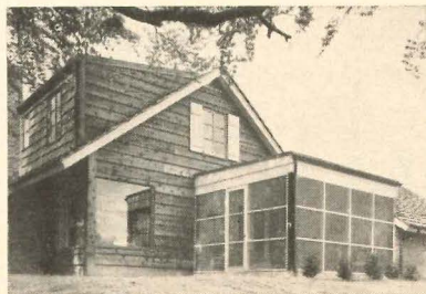
Dormer windows and screened-in porch, seen from the side and rear, make the house look much larger. Dormer gives extra light and air to upstairs bath and bedrooms. Screened-in porch opens off the dining area.
