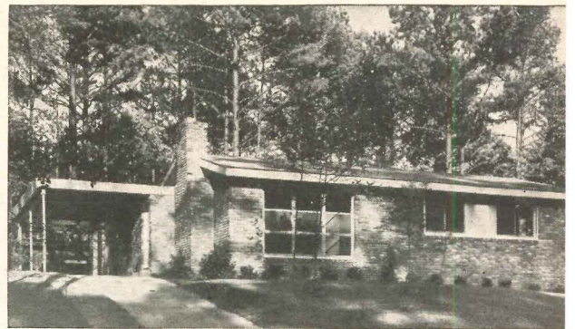
Front of house shows how well trees shade glass. Brick walls are insulated.
