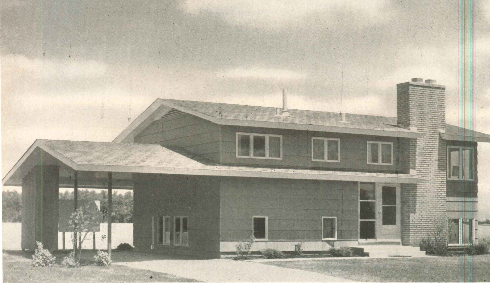
Elevation seen from street shows strong resemblance between this version of two-story house and today's popular split level design
