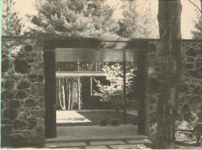
Entrance to house is through one of two gates that lead into walled garden. Sliding doors can close off gates, keep out storms.
