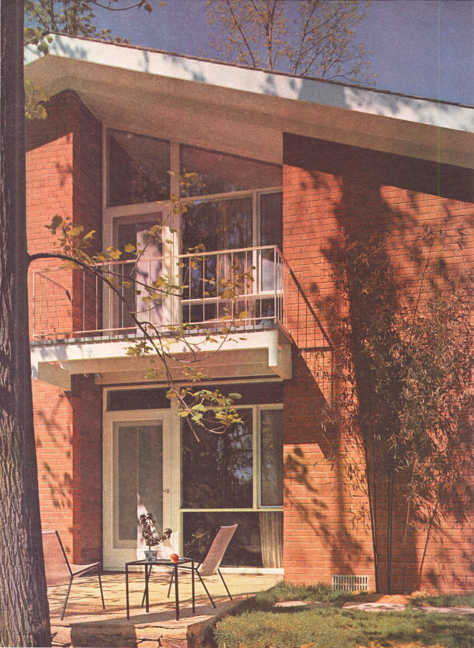
Balcony is an extension of an inside balcony. With their traditional exterior materials, the balcony and terrace show how good designers can learn from forms of the past and still achieve a contemporary building. Grilles at ground line provide ventilation for crawl space area.
