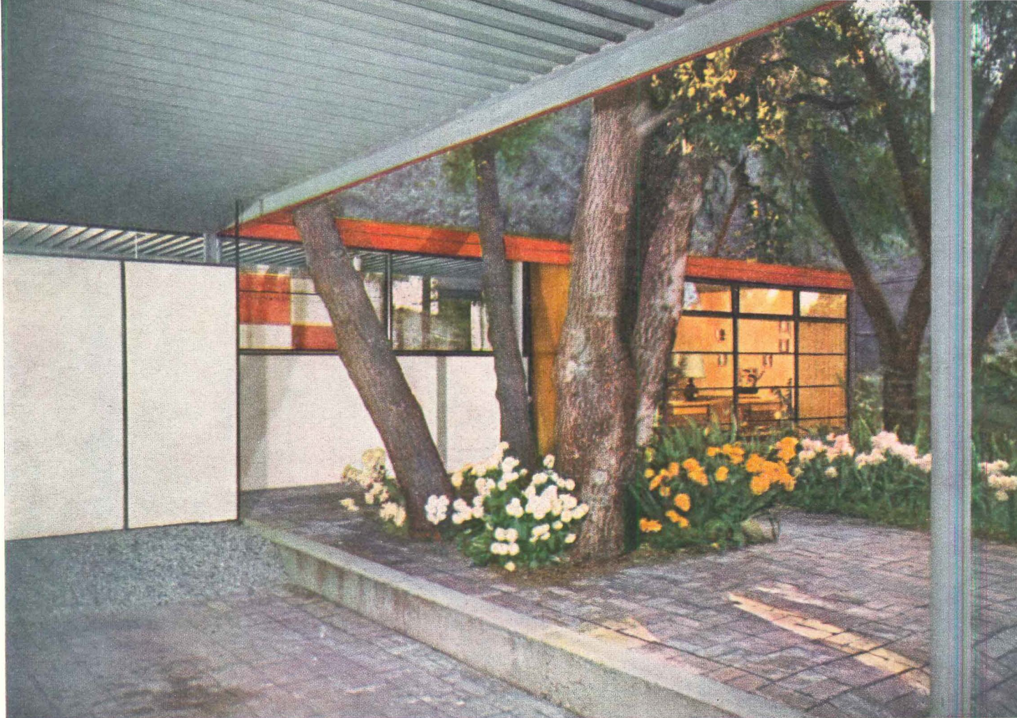
Walls of steel-framed house are finished with painted plywood. Windows at far right are steel factory sash, those at left slide.
