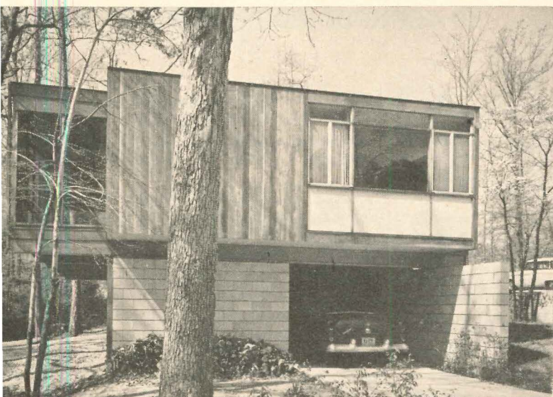
...e view shows carport in lower level. Upstairs, a 40' long, 6' p screened porch faces downhill. Vertical siding is redwood.
