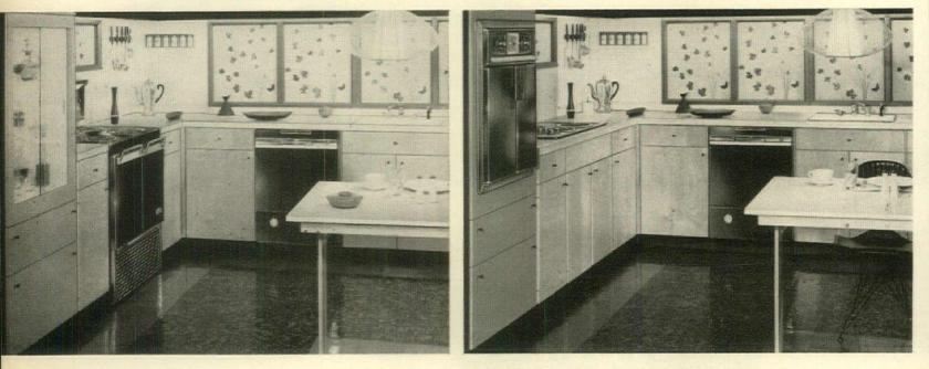
FLEXIBILITY of modular design is shown at its money-saving best in the Oriental Magic Idea Kitchen with Cabinets by Bilt-Well. At the left, the 30-inch RI-39-58 Range blends into a compact cooking center. At the right, in the same cabinets, the RBW-101 Built-In Cooking Top drops into position; RBW-90 Wall Oven slips into the glass cabinet space. Either way, Frigidaire makes it easy to satisfy every home-buyer!
