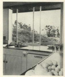
**Sliding aluminum window** will be marketed nationally in 1958. Window has automatic latching, double weatherseals, fin for nail-on installation.
