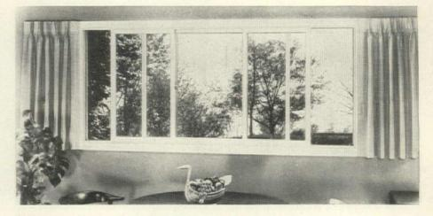
**Sliding wood window units** are removable for cleaning, painting. Called Style-Trend, they are available as sliding units, or as combined sliding and picture units. Available optionals: drip cap, inside trim, storm sash, aluminum screens, and self-storing storm sash and screen units.
