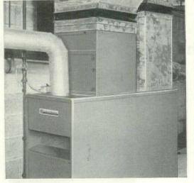
4 SHOW YOUR HOUSE "READY FOR AIR CONDITIONING." Where the plenum would ordinarily rest on the furnace, install the jacket for an American-Standard summer air conditioning evaporator unit. Apply a sticker reminding the buyer how easily he can add whole-house cooling and enjoy complete, year 'round comfort.
