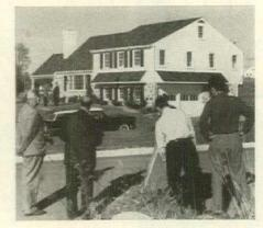
borough, and Max Fink show how they each have used the "new look" in asbestoscement siding, and why. They detail how —with a full undercoursing of fibreboard to "kickout" the shingle and reinforce it —the flat look that used to be asbestos' giveaway has been eliminated. They point out the savings they have enjoyed in using asbestos shingles, the simple installation, the wide variety of colors and easy mainte-
