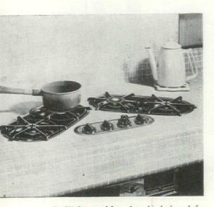
**Built-in cooking top** is designed for installation with ceramic tile. Burner pans fit level with counter top and small lip on pan allows a tile setter normal leeway in fitting tiles around pan area. No cut-out in the cabinet front is needed since controls are included on the cooking panel.
