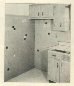
**Plastic wall tiles** in  $4\frac{1}{2}''$  squares are now molded to give appearance of four small squares. But it has 50% more water seal contact with the wall, goes up faster than small tiles. Costs and application methods are the same as regular  $4\frac{1}{2}''$  tile. Known as Modern Mosaic, the new tile is available in 15 colors, may be combined with individual quarter tiles as shown above. Artcrest Plastics Co., Chicago.
