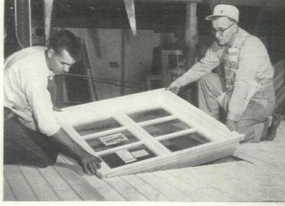
Window installation is easy (calls for no wedging) because opening has been framed and trimmed accurately. Casement and double-hung units are already glazed, hung and primecoated when Auburn buys them, get final paint coat at site.
