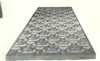
AMERICAN HOUSES' TEST FLOOR, 1956: 4" thick phenolic-and-paper floor panel doubles as warm air plenum, can span 8' under normal residential loads.
