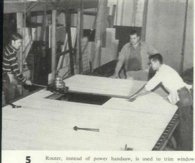
Router, instead of power handsaw, is used to trim window openings. Reason: it's faster, more accurate. To adapt router for this awkward job, Auburn attached two pipe handles and steel finger that guides router along rough frame opening.
