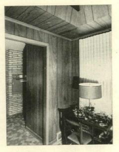
**Prefinished plywood paneling** in ten finishes is now available with complete paneling package. Known as PlyWelsh, the products include the paneling, color blended putty sticks to fill nail holes, and stains to match surrounding builtins, doors, etc.
