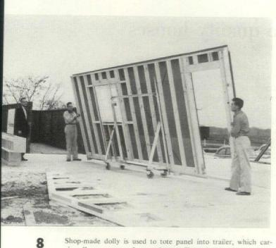
Shop-made dolly is used to tote panel into trailer, which carries all components for one house. Two chunks of scrap lumber, nailed to bottom plate, serve as bumpers to protect panels. They will be knocked off before panel is erected.
