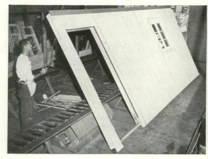
Finished panel is lifted off assembly conveyor and set on dolly (photo 8) by two electric hoists. Smart idea: to keep door frames from buckling, bottom plate has been extended under opening—will become stool when panel is erected.
