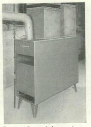
Utility furnace in basement. Cumbersome return air duct is visually displeasing—a sales *disadvantage*.
