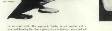
assembly. Engineers found that individual panels in the plane's body
