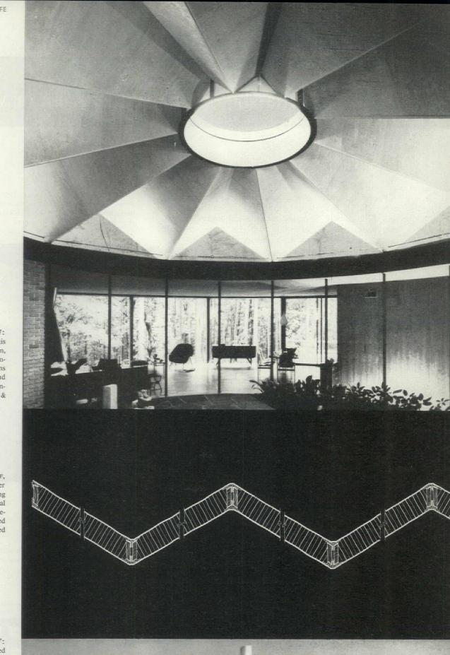
FOLDED ROOF, Atlanta, Ga. 1957: Circular patio in center of this house is covered by stressed skin, wooden folded roof. Steel compression ring in center contains skylight. Tension cable around periphery keeps roof from flattening out. Architects: Alexander & Rothschild.
