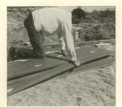
**Black Styrofoam** is now scored so it can be broken to different widths right on the job. Grooves at 3", 12" and 20" marks across the 24" width of each board make on-the-job selection of sizes quick and easy, give a choice of size to fit most foundation and cavity walls. Called Scorboard, boards are 1" thick, 8' long.
