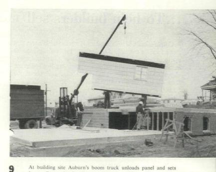
At building site Auburn's boom truck unloads panel and sets it up. Crane also handles trusses and partitions. Five working days after components are delivered to site (shop-to-field move costs \$40) house is completely closed in./END.
