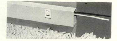
NATIONAL HOMES' SHEET ALUMINUM RACEWAY, 1957: Raceway wiring system developed by this prefabber may cut costs in half. Baseboard radiation pipe and cover fit under raceway.
