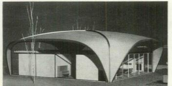
ALCOA'S "CAREFREE HOUSE" for 1958: Panelized roof, with outside and inside skins of anodized aluminum, core of foamed styrene. The panels will span clear from ridge-beam to loadbearing exterior walls, form an overhang. Early study by Architect Charles M. Goodman.
