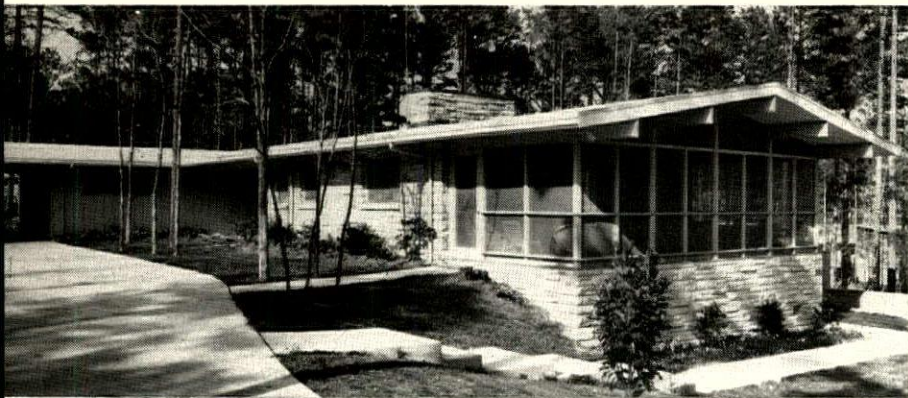
Big overhang partially shades even low sun. Overhang at the gable end makes screened porch fit into house like another room. Architect: Owen F. Smith; Builder: Inland Construction Co.; Raleigh, N.C.
