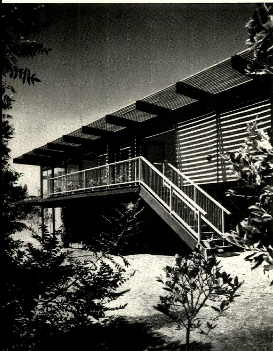
Striking patterns are created by this latticed overhang. Open overhangs can control sun, add more architectural interest. Architects: Winslow & Waltz; Builder: E. W. Leishman; Brentwood, Calif.
