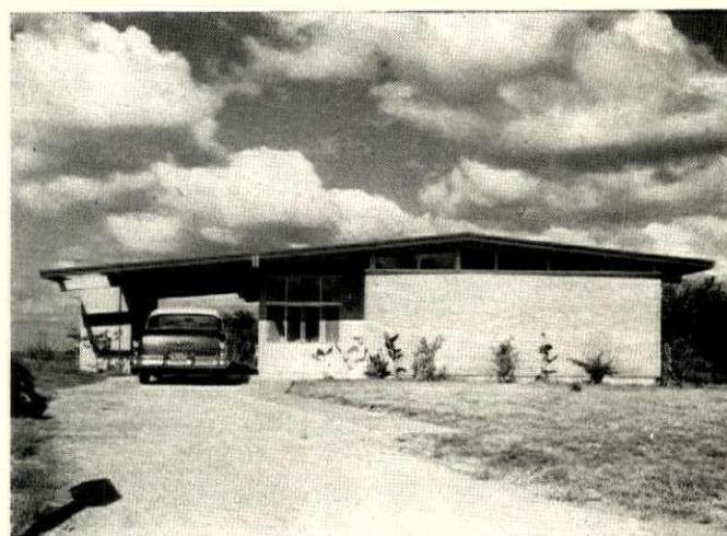
Small house looks bigger because overhang becomes the carport roof. Large windows are set back to widen overhang. Architect: John A. York; Builder: Arroyo Estates; Harlingen, Tex.
