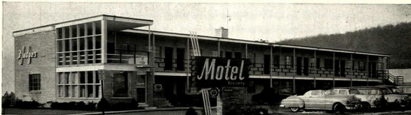
The new 24-unit, 2-story "3 Judges" Motel, just off the famous Wilbur Cross Parkway, at New Haven, Conn. Architect, Caproni Associates, New Haven; consulting engineer, R. S. Leigh, Woodbury; plumbing contractor, J. V. Ursini Co., New Haven.
