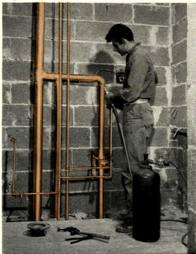
Copper tube and solder-joint fittings make a compact, space-saving installation. A 3" copper tube with fittings can be installed within a standard 4"-wide partition.
