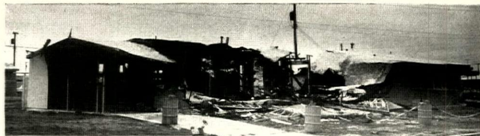
AFTER: Occupants call it "Malfunction Junction." Escaping gas blew up this duplex.
