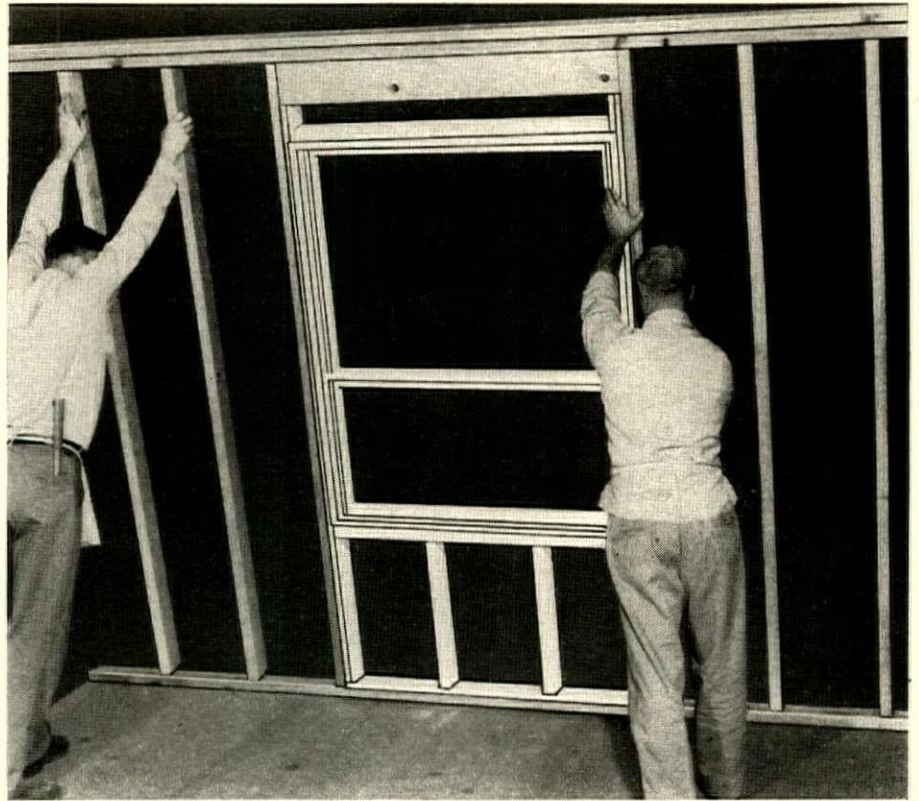
NEW STRUCTURAL WINDOW is assembly of cripples, nailers, frame and sash. Upper cripples are cut off with discontinuous headers.
