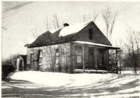
RUN-DOWN HOUSE symbolizes move Oskaloosans made from older neighborhoods. Forty such houses have already been torn down and 135 others are slated for demolition.
