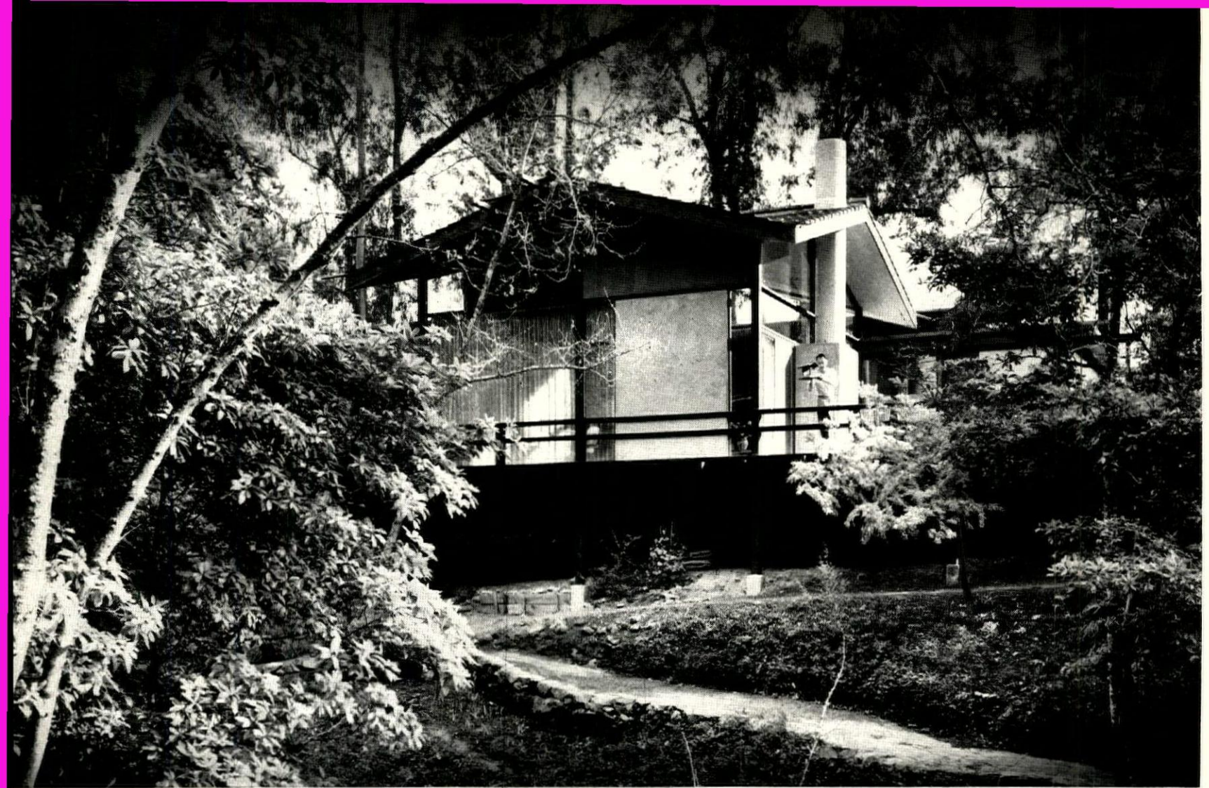
HOUSE is raised off ground level by posts supporting deck. This, with paneled exterior and four-gabled roof, add to Japanese effect.
