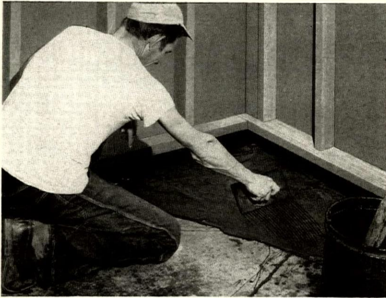
① Spread mastic over waterproofed slab.
