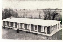
Crystalite aggregate is a white marble roofing material that is 80% to 85% reflective. The material will not fade, discolor, crumble, or deteriorate, but by reflecting heat should reduce air conditioning costs. Stone weighs 90 lb per cu ft, is used at 350 to 400 lb per sq rate on 4½-in-12 pitch roofs. Crystalite is shipped in bulk or in 100-lb multiwall bags. In cost Crystalite competes with the cheapest aggregates.
