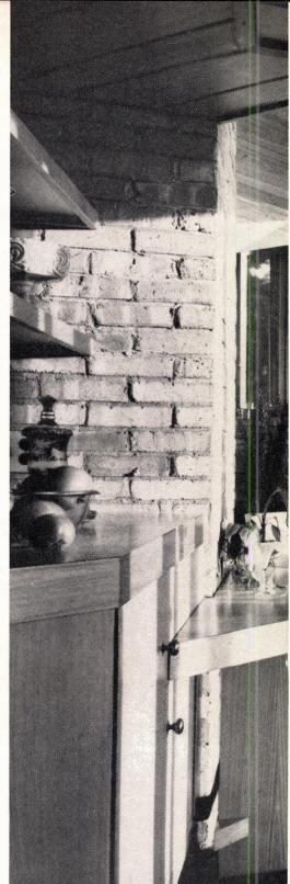
Strong horizontal lines in the living room (above) are enhanced by the contrasting vertical window mullions. Mr Wright rarely uses mullions at corners; instead he miters the glass as shown here. Furniture was designed by the architect.
