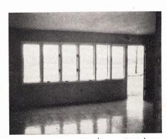
REAR WINDOW WALL in one-story house combines fixed glass with wood casement windows. Dado-high glass wall ends at door, which opens onto back yard.
