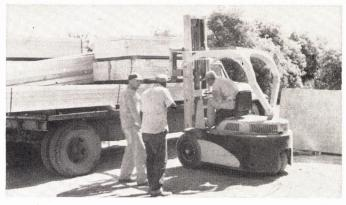
**FOAMED CONCRETE SLABS** called Siporex come strapped on pallet. Fork lift is used for rapid unloading. Slabs are 8' long, 3 and 4" thick.
