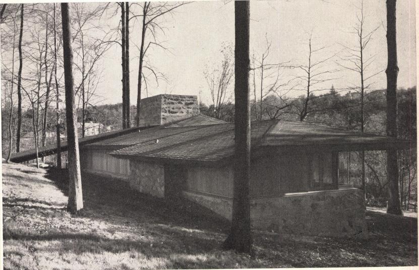
Rear elevation is as carefully articulated as the others. The masonry base (here 2'-6" above the bedroom floor) becomes a retaining wall. The roof repeats the gentle undulations of the site. Note how over-
