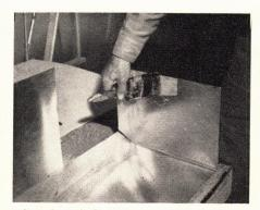
when shape is formed, coat with adhesive ...
