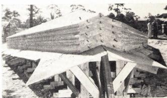
ROOF SECTIONS are cast one on top of another, 3 and 5 in a stack.
