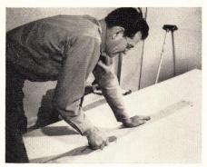
You can cut Clad-Rex with linoleum knife . . .
