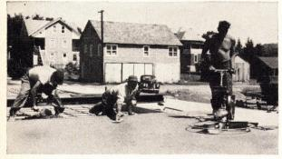
**FINISH FOR WALL PANELS** is very smooth to take paint inside and out. They are first wood floated and then steel troweled with the power float at right.
