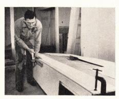
To bend it, score metal with glass cutter . . . and bend over table edge at score mark.
