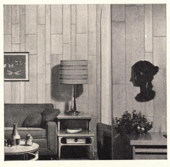
LOC-WALL: Idaho White Pine and Inland Red Cedar in Formal and Traditional styling; Larch in Formal styling. Plywood Panels look like individual boards of random lengths and widths, edge and end-Vee'd. Also produced with Gruve-Ply pattern. Interlocking furring strips are already attached.
