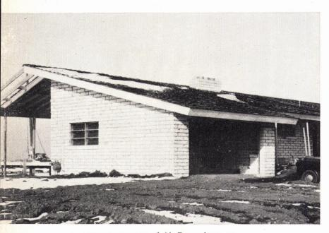
**EXTERIOR WALLS** of this Denver house are made of Durox block—a foamed concrete. A wall like this has a U factor of .11, works well in the north. Exterior gets silicone treatment.
