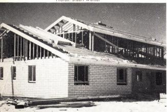
**BLOCK WALLS** of Durox for first floor of this Colorado house are combined with stud walls on upper half story. Sole plate for gable end is nailed right into block wall.
