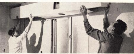
position form on adhesive-coated wall, roll in place to get sure contact.
