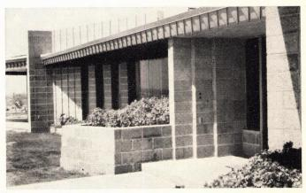
FOR PLANTERS that become part of the exterior, block is laid in common bond while walls are stack bond for greater emphasis.
