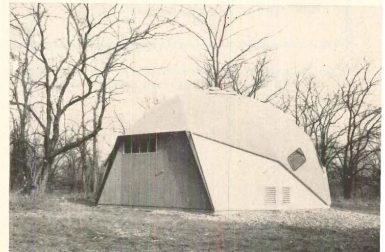
3 Adjacent panels are bolted together. Four pairs of base triangles, plus door assemblies, complete base of dome. Holes are for ventilators.
