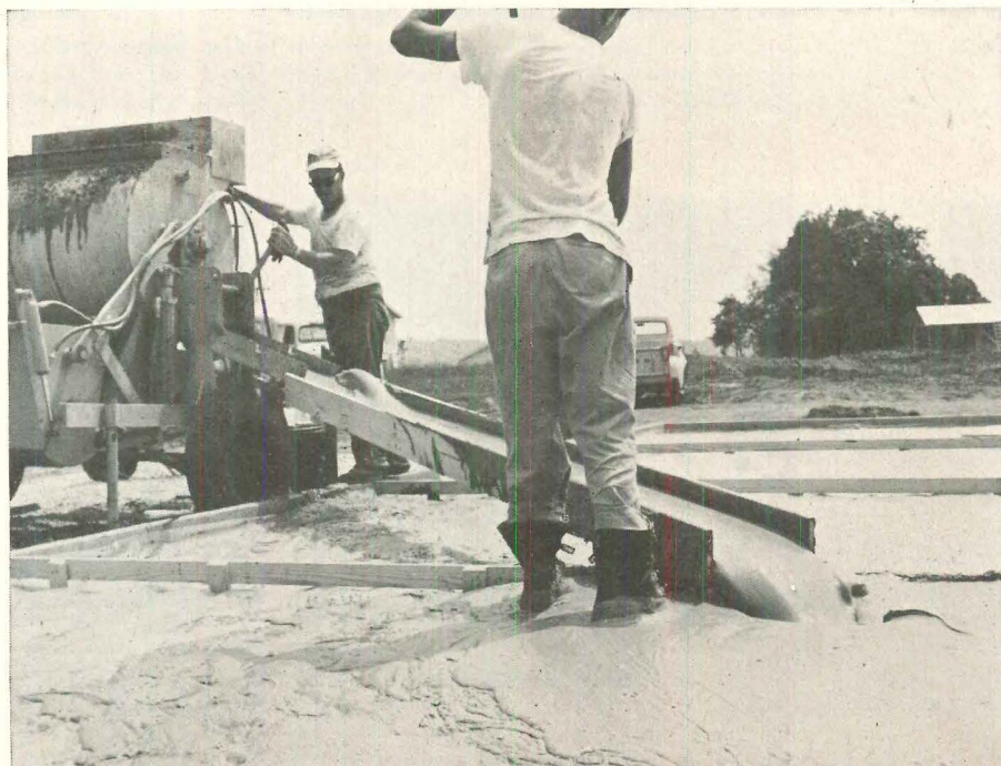
Insulating foam concrete has smooth consistency. Called Betocel (p 123) the mixture is sand, cement, water and a
