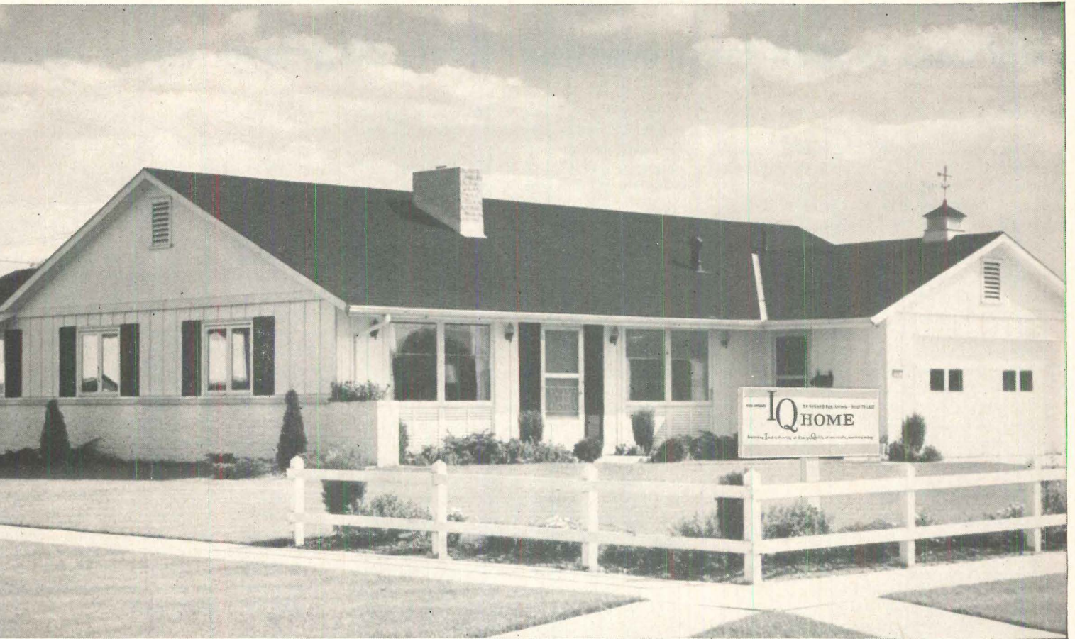
Schmitt of Bob Schmitt Homes, Berea, Ohio, uses Curtis windows to vary proportions of masses and styling with one basic plan.
