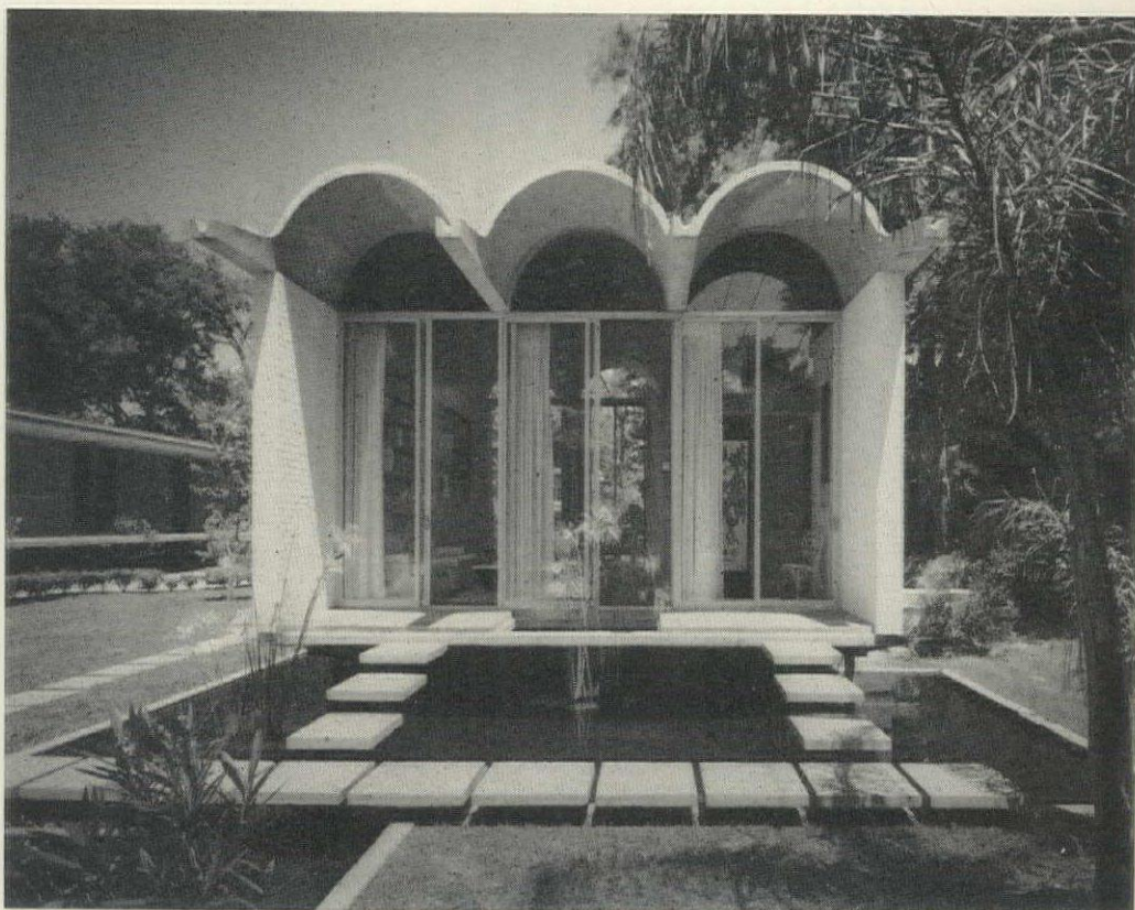
Guest pavilion is set above a pool which adds to the fanciful and floating effect. Extended roof beams become waterspouts in heavy rains.
