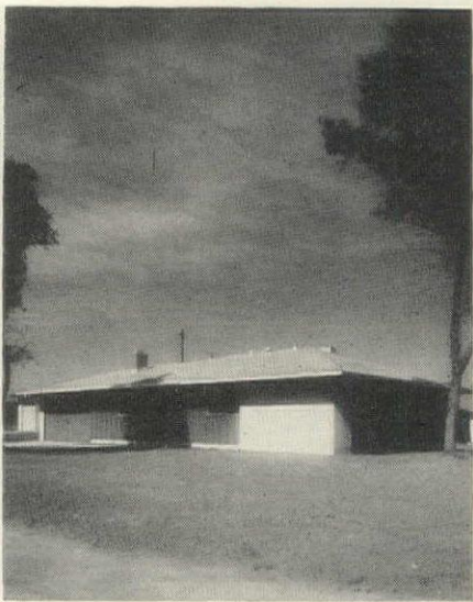
SIMPLE HIPPED ROOF covers both house and garage in this version of the basic scheme.
