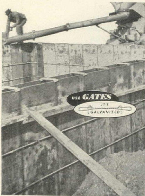
Vix Construction Company residential development, Englewood, Colorado
