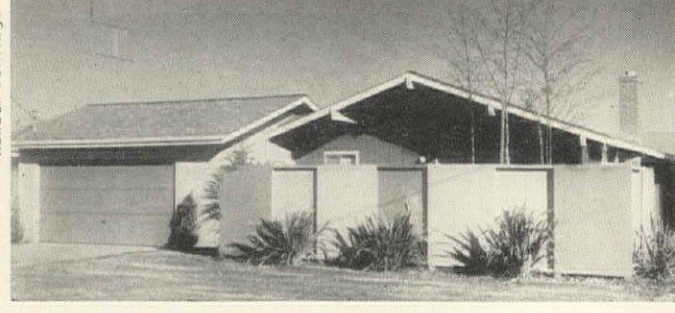
NARROW END TO STREET , this variation reverses orientation of house and garage; has glass gable end with fence to provide privacy.
