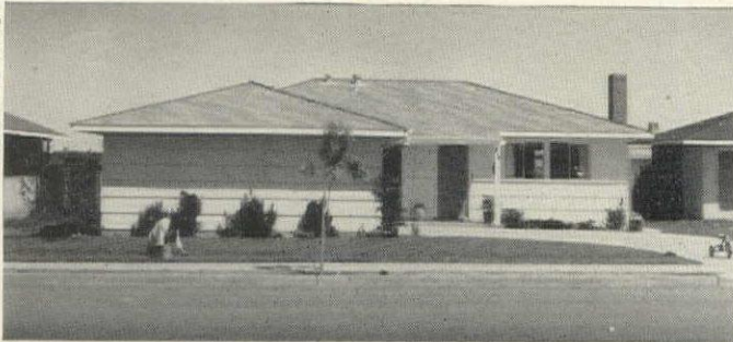
HIP-ROOFED MODEL has side-entering garage on bedroom end of house, gable-end fireplace.
