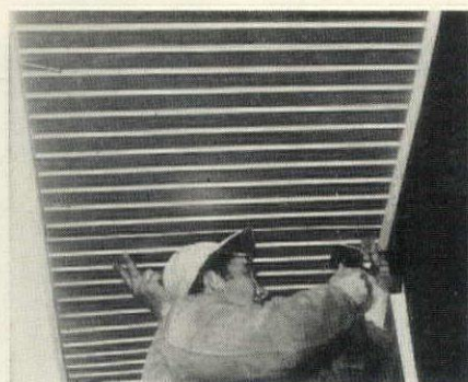
ALUMINUM SOFFIT cost Buchanan less (17¢ a sq ft) than soffit he previously used (18¢). Soffit panels are ribbed, diamond-embossed sheet (0.019" thick), perforated to let air circulate. They are supported by fascia board
