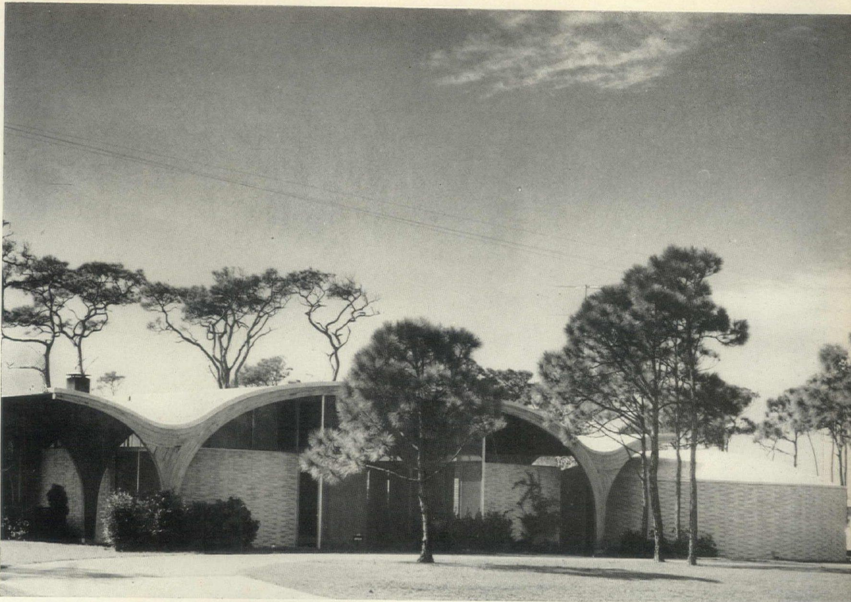
Arched roof stands free of actual enclosure of house. Arch height at center of span is 14'; wall height is 8'.
