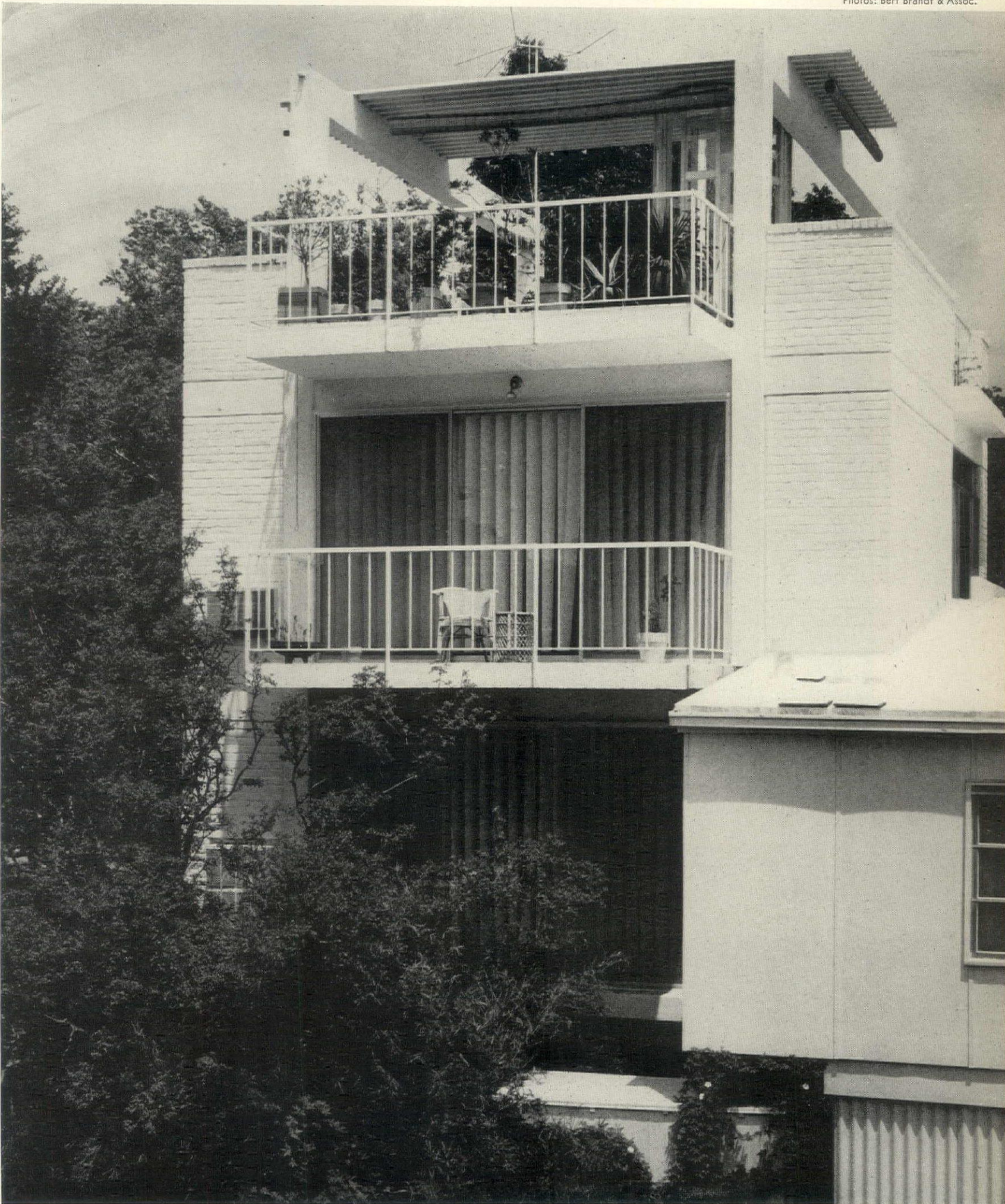
Balconies open off roof garden and third floor bedroom and library; they provide outdoor living at each floor and add valuable space.
