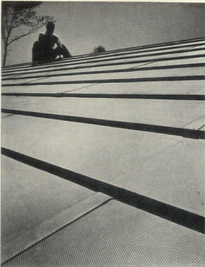
ALUMINUM ROOF CLADDING fits around plywood panels, stops water, holds panels together. Battens cover openings where panel ends meet.
