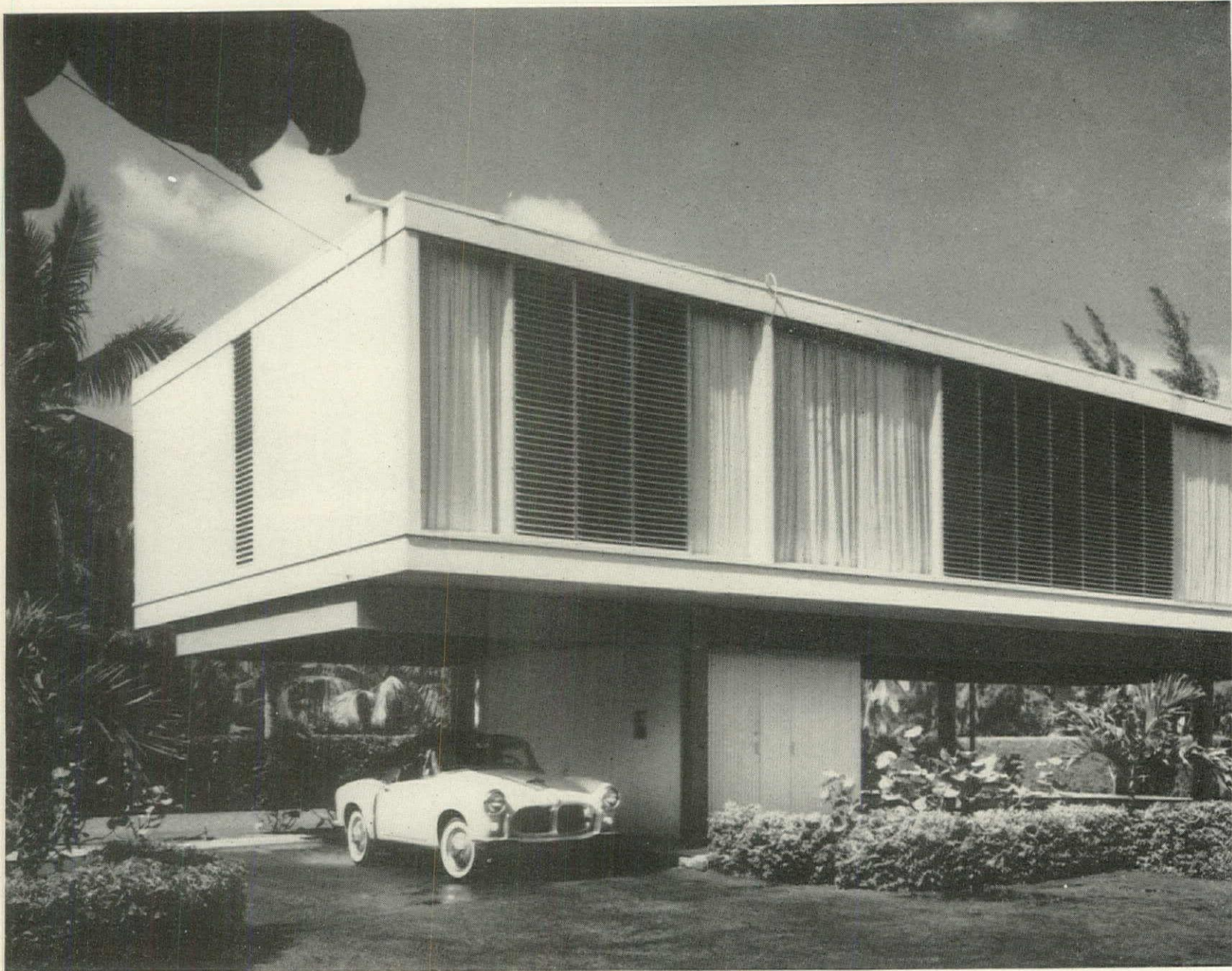
House is cantilevered from four steel columns. Stair was enclosed on lower level to separate carport from patio.
