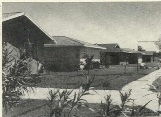
ROOF VARIATIONS enhance one-of-a-kind look by giving each house a different "profile" as well as a different "full face."
