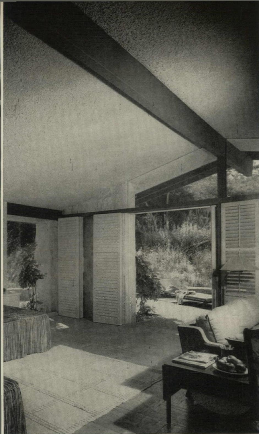
THE TEXTURED-PLASTER ceiling unites the indoors with the outdoors in the master suite living area ( Below ). Keymesh used over gypsum lath in this construction.
