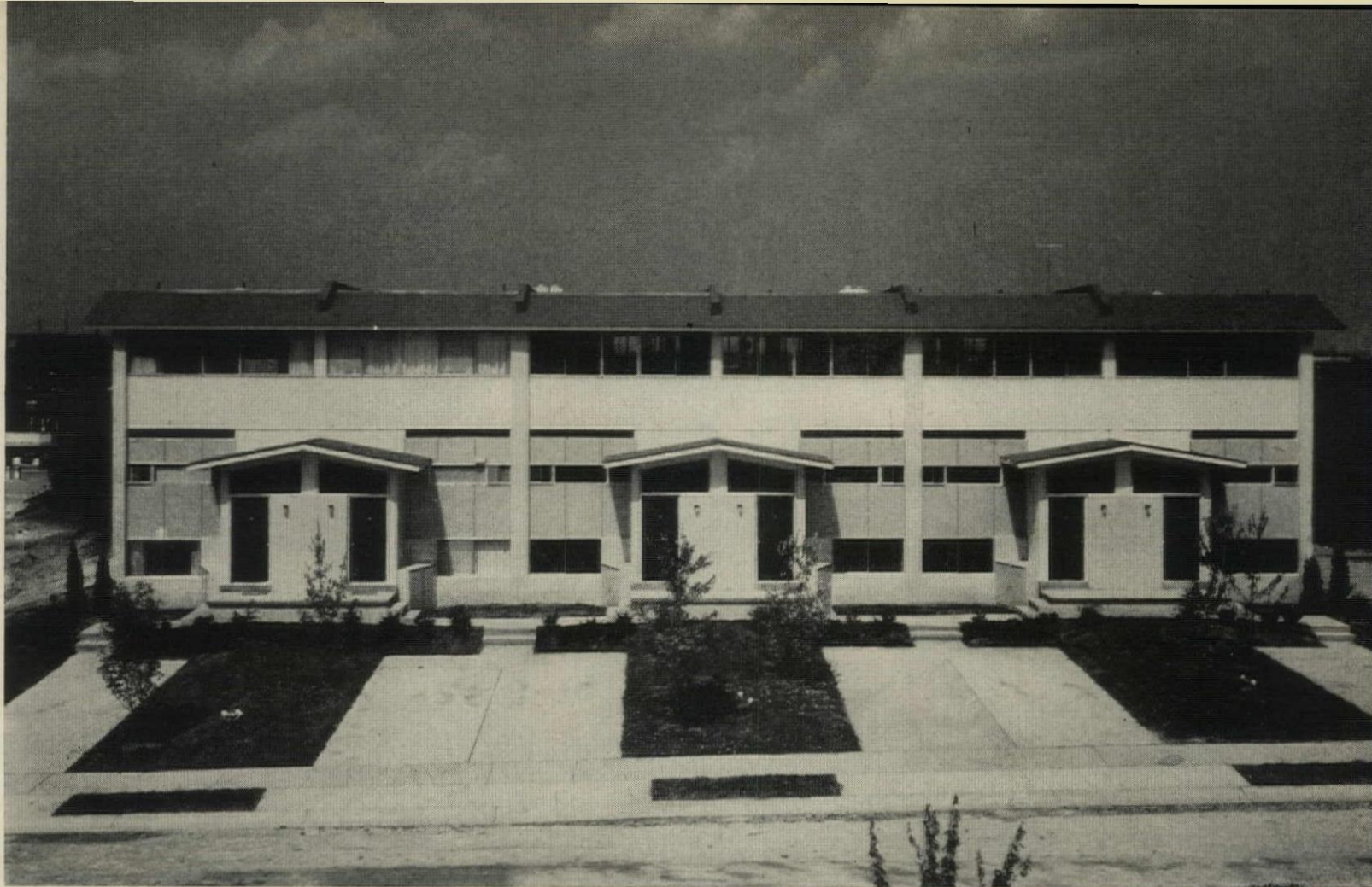
CONTEMPORARY DESIGN is used on six-unit building. Units are 16' wide, have split-foyer entries, and aluminum wall panels, sell for $11,990.
