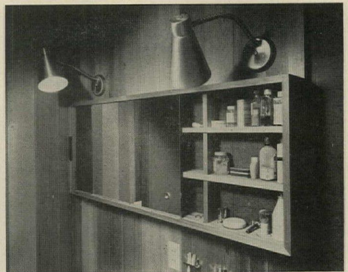
BATHROOM CABINET is simple wood frame routed to take sliding doors; one door is mirrored, one is Masonite. Unit was made on the job.
