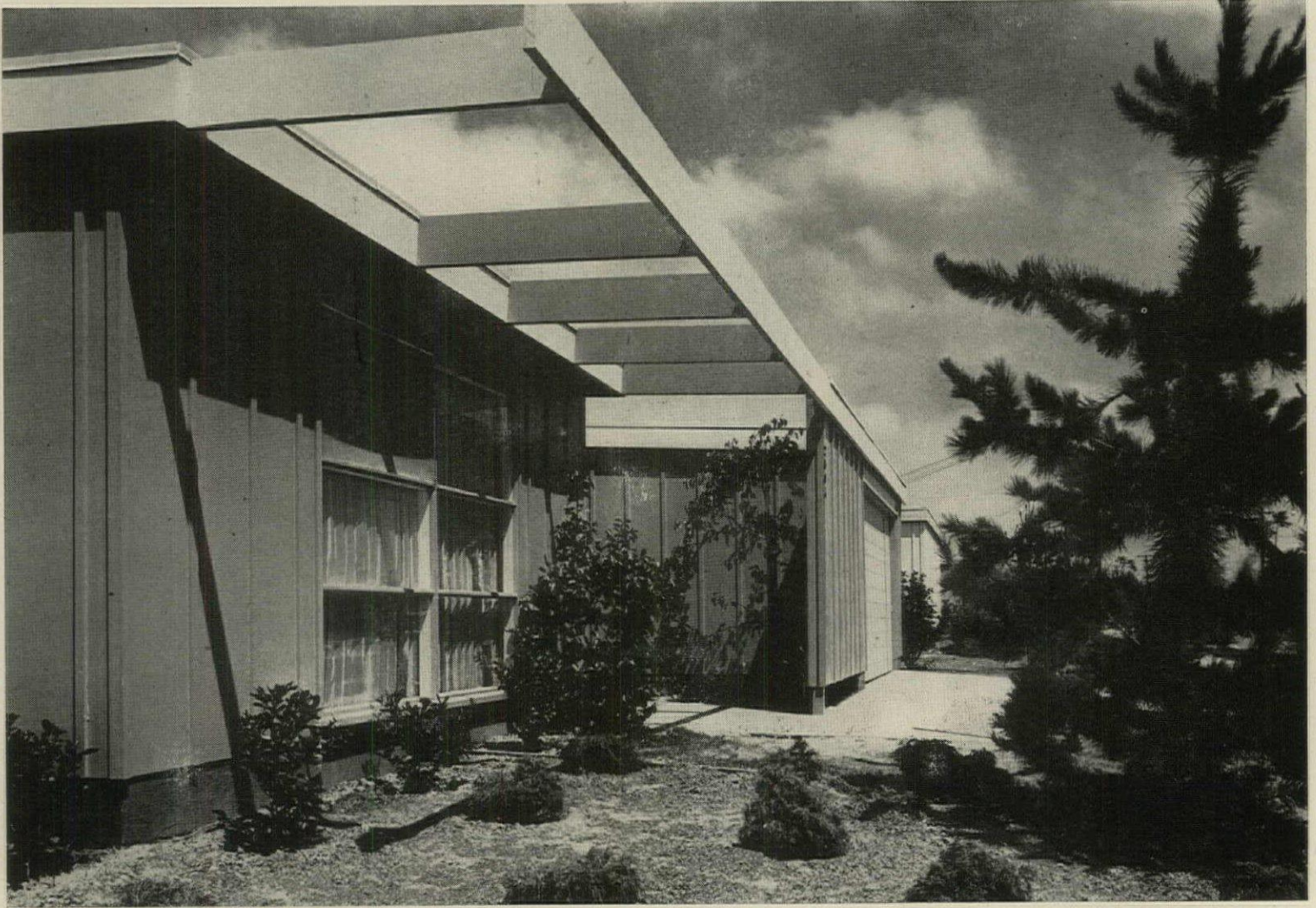
NEWEST HOUSE in AHG's line is the $18,850 four-bedroom "Hacienda." Fifteen sold before the model opened; it is now AHG's fastest seller.
