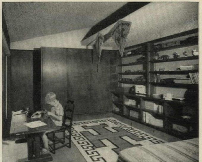
THE ROUGH-TEXTURED plaster ceiling is ideal for the boy's bedroom. Keymesh and Keycorner are adding superior crack resistance to this construction.
