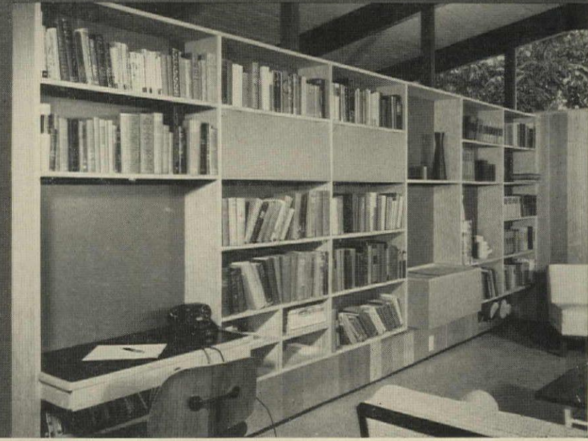
Storage wall is also used on living-area side. Shelves are wall-hung. Storage wall cost about $15 a lineal foot.
