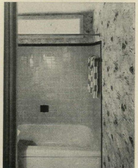
INSIDE BATH has opaque glass panel to borrow light from windows in master bedroom.
