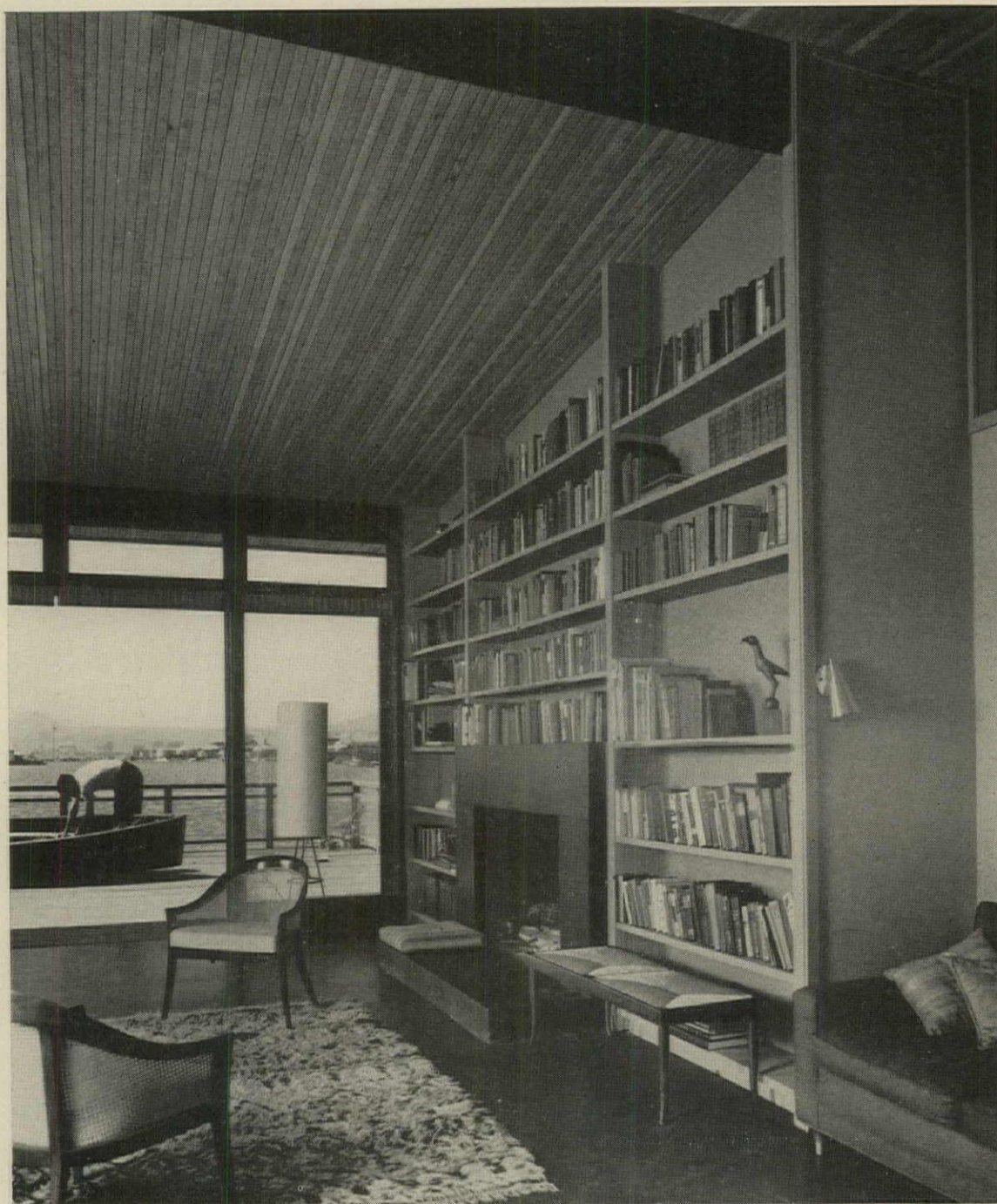
LIVING ROOM , like all other rooms in house, has exposed 2x4 ceiling. Fireplace is precast concrete, treated with black wax.
