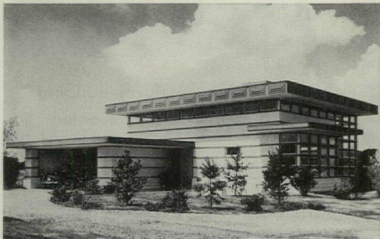
NEARLY SQUARE HOUSE is 18' high, has band of windows around house under 2' ornamental fascia. Cream ocher walls have blue battens.
