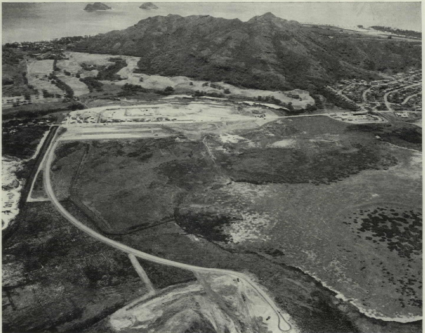
700-ACRE MARSHLAND TRACT is being built up with fill from mountain in foreground. A 72-acre lake will form at right.
