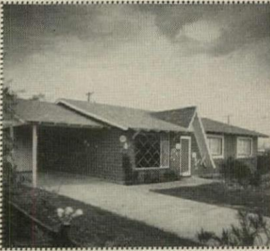
CHEAPER model ($9,950) is identical to original plan except "L" wing has been lopped off. There are 1290 sq ft of living area, at $7.75 a sq ft.
