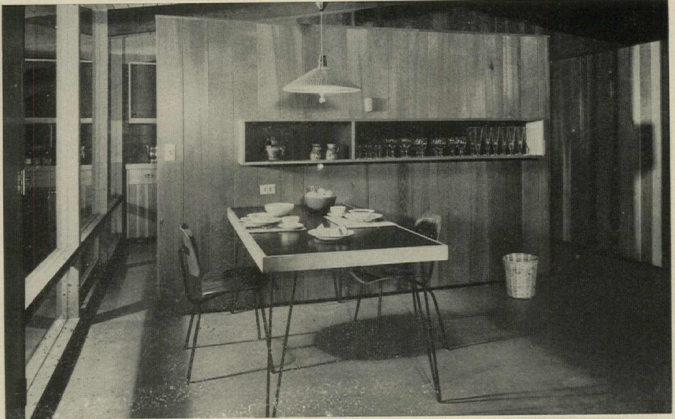
DINING AREA has wall-hung cabinet convenient to table for dishes and glassware. Cedar-faced partition is 6'-8" high, screens off kitchen.
