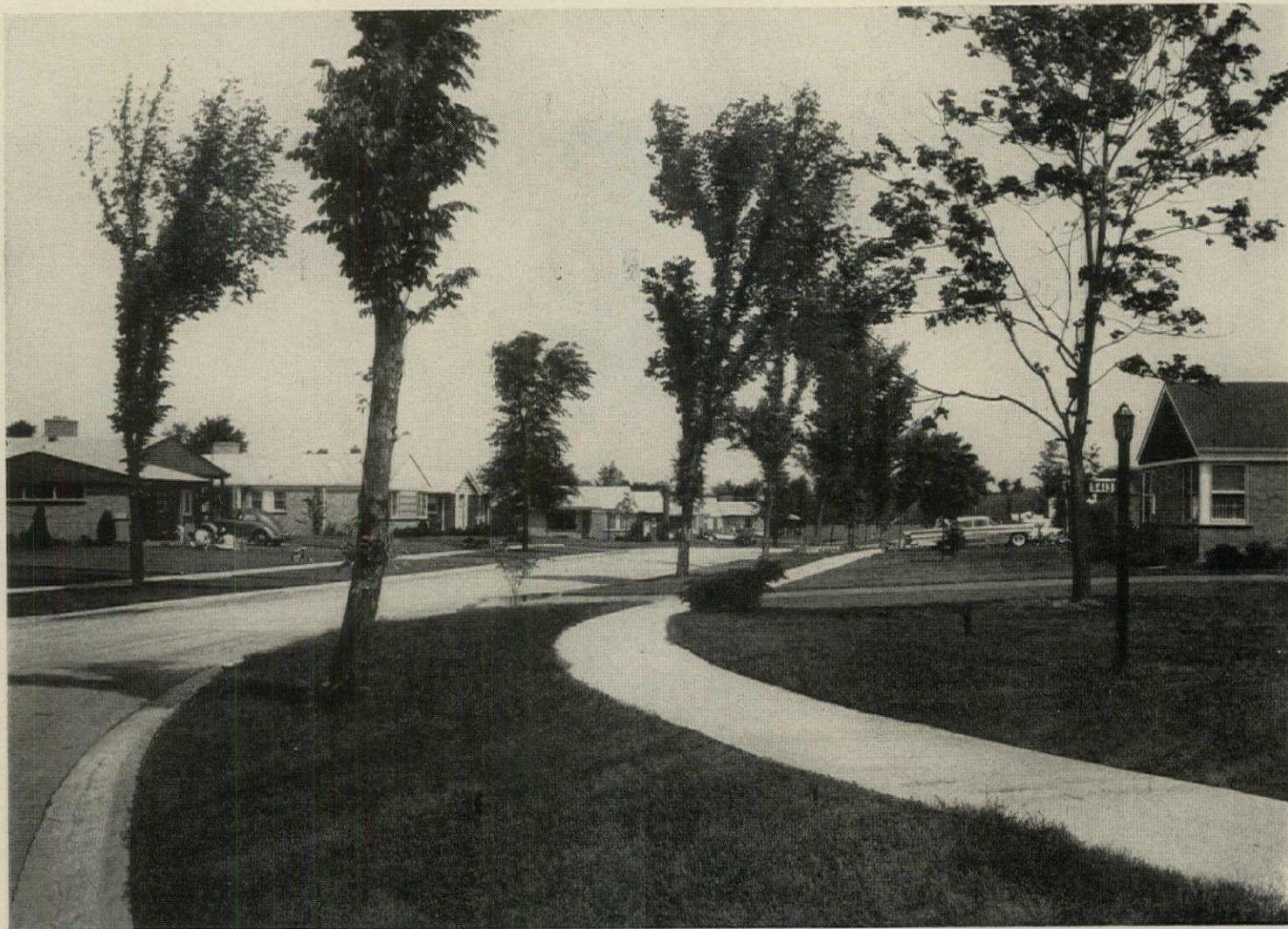
NO POLES OR OVERHEAD WIRES clutter up Paul Schwendener's development in Western Springs, Ill. Power and phone lines are underground.
