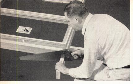
Seven steps instead of 22! Simply cut two load-bearing struts to fit header construction you use. Nail Strutwall to adjacent studs, tilt up with wall. Two-thirds of conventional framing, installing and finishing is eliminated.
