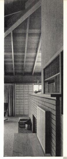
Because redwood provides a high degree of insulation, the ceiling in this handsome room also serves as sub-roofing. Note how the color variations in the boards add visual interest.
