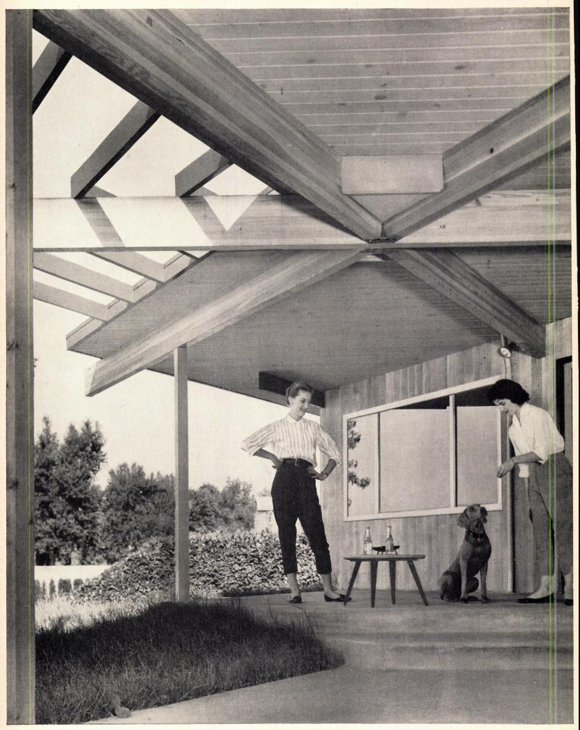
Strong selling point of this home is a roofed-over patio featuring laminated wood beams continued from inside the house. Beams support extended roof and with
