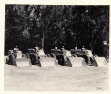
Four new power shovels have been added to the Case rubber-tired line for 1960. Smallest unit is 2-wheel drive, 1-cu yd model with a 3000-lb capacity. Other units are 4-wheel drive, carry 5,500 to 9,000 lb. Optional fittings include pallet forks, block forks, dozer blades, brush stackers, snow plows.
