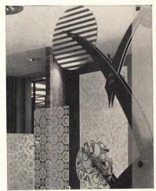
Laminated glass is made of two layers of plate glass bonded with a vinyl buty-rate inner layer. Decorative imbedments are held in the sandwich. Vinyl butyrate not only prevents shattering but in special formulations can act as light, heat, and sound insulation.
