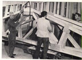
ROOF TRUSSES are standard with builders in many areas. Nail-glued truss shown here is one of several types used.
