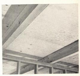
**Underside of floor** presents an attractive panel and beam basement ceiling, unmarred by a complicated network of joists and bridging—a big feature with home buyers.
