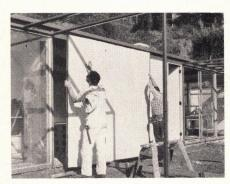
**NON-BEARING PANELS** being set into place are ½" plywood, sandwiching wool insulation.
