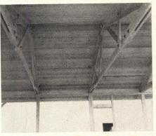
Potlatch decking is made of new glued-up lumber that can be made in almost unlimited lengths. Stock now being made (used above) is 13/8" thick, 22" wide, 16' long. Plylumber can span 8' between trusses.
