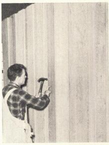
Redwood siding is now made in a reverse board and batten, smooth on one side, resawn on the other. Textured face takes paint better, resists weathering, hides scuff marks. Boards are 3/4" thick, battens 3/6" thick, to give more coverage per board foot.
