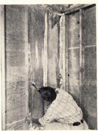
For light tacking jobs—where there's room to swing and long reach is an advantage—the H5 Stapling Hammer gives you fast fastening action. Light—yet strong enough to drive staples with 36", 14" or 56" leg lengths into soft materials or wood.
