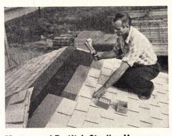
Most rugged Bostitch Stapling Hammer of them all—H4 Heavy Duty Model. Cuts asphalt shingling time on new roofs by half or more, say builders who wouldn't be without it. Every swing drives a 34" galvanized staple into the work, spreads the staple legs for greatest holding power.
