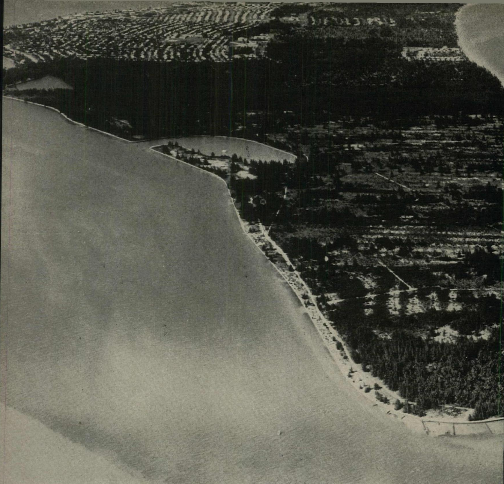
AT CAPE FLORIDA, 547 acres of pines and palms are being converted into a $500 million island development 5 miles south of Miami Beach.
