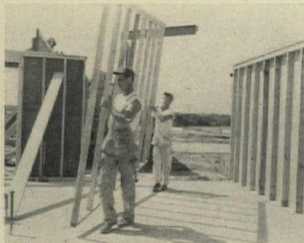
9:25 AM Light interior section is easily carried by two men. One exterior panel is left out so men can get into house.
