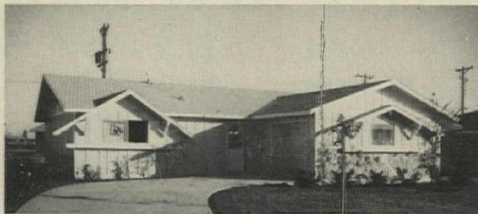
EXPERIMENTAL MODEL has frame walls, foam-core partitions.
