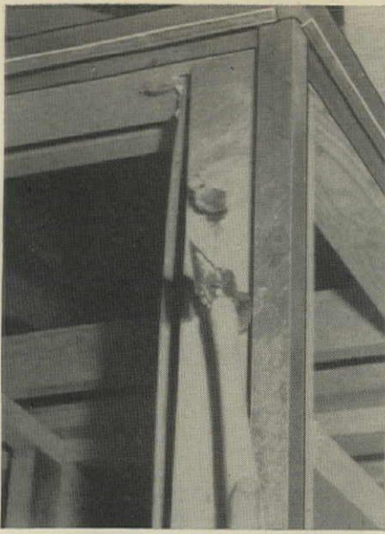
AT OUTSIDE CORNER a clip aligns all three steel channels. Strips can be adjusted to make true vertical or level lines.
