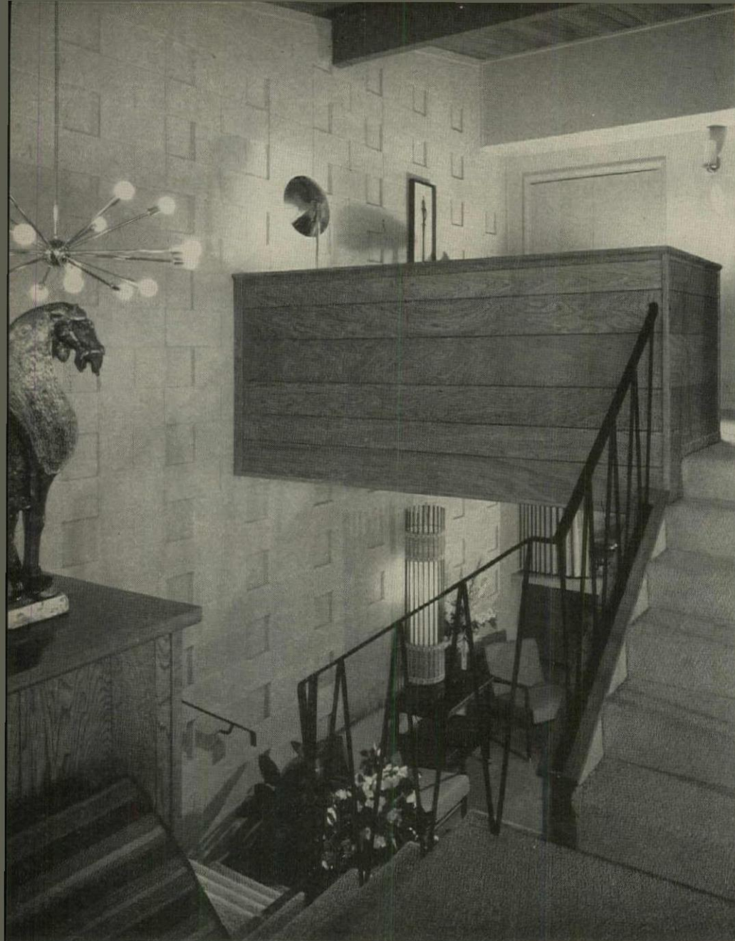
Offset units of standard block form an eye-catching wall to complement the natural wood of the balcony.
