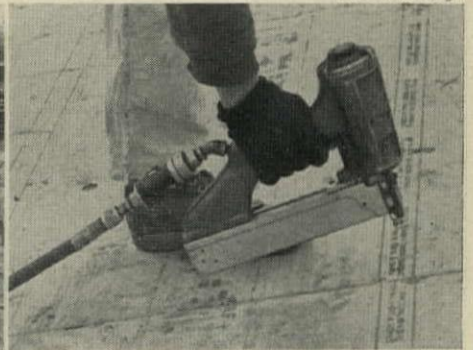
ON-SITE EQUIPMENT includes bell-bottom trencher . . . power wagon and tools . . . staple gun for roof sheathing.
