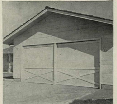
GABLE END facing street gives different look to this garage. Colors alter patterns.
