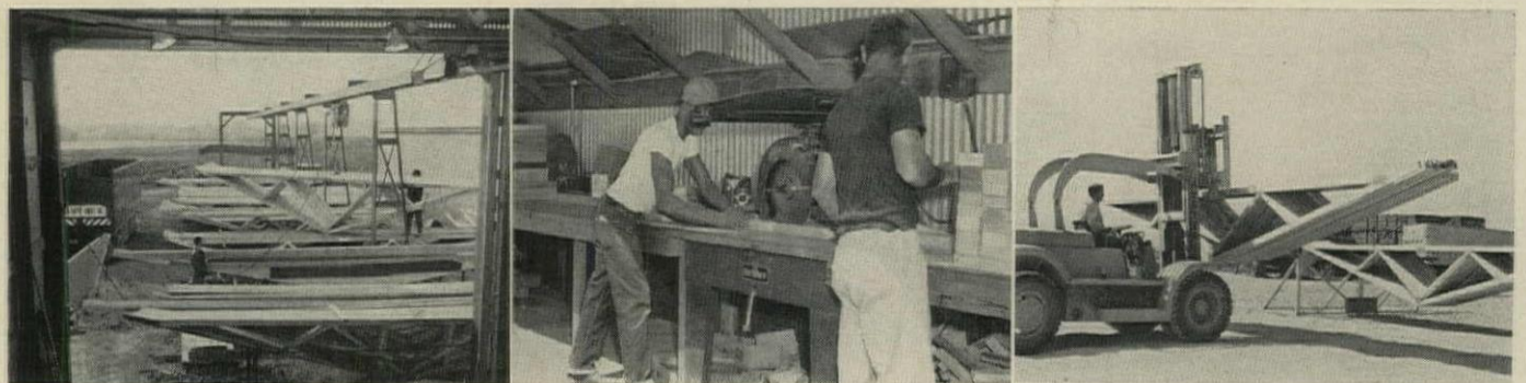
POWER EQUIPMENT at plant includes 2½-ton crane (left), power saws which precut standard pieces, and forklift truck.
