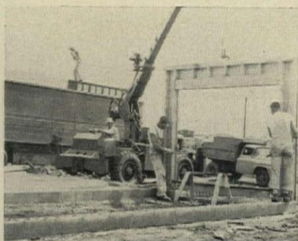
8:05 AM First panel is dropped in place. Crane can swing many panels from trailer and spot them on the slab without moving.
