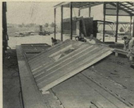
AT END OF LINE completed panel is lifted from the table by overhead hoist. From here, panel moves to shipping dock.
