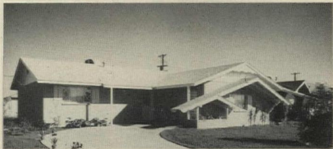
TODAY'S MODELS have block exterior walls, frame partitions.
