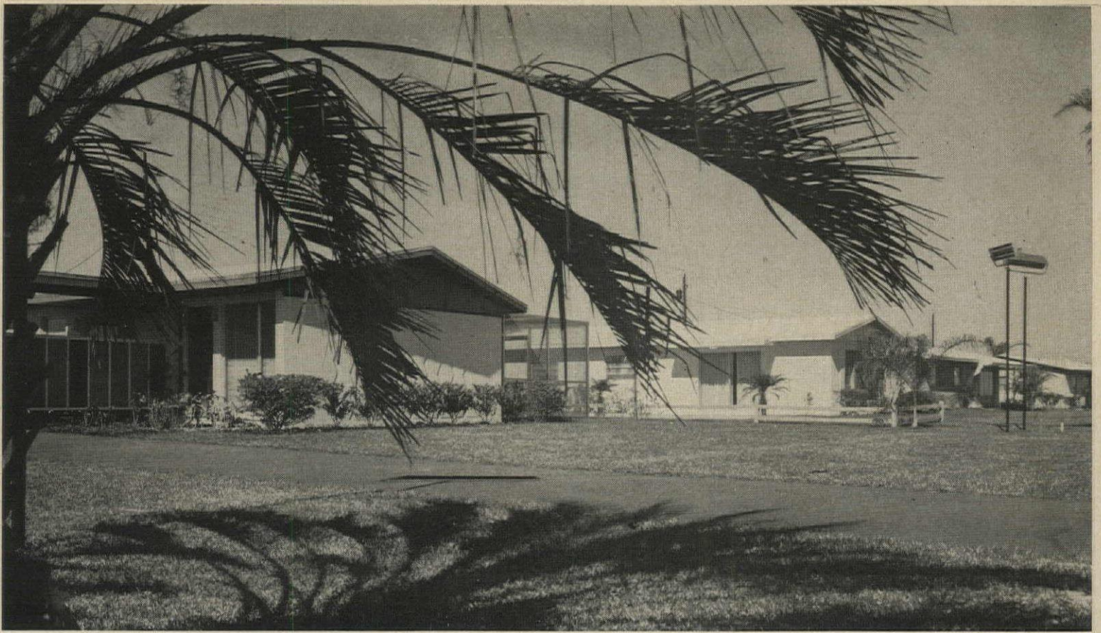
WIDE OVERHANGS and screened outdoor living areas on house at left are also available on rest of models (shown at right).
