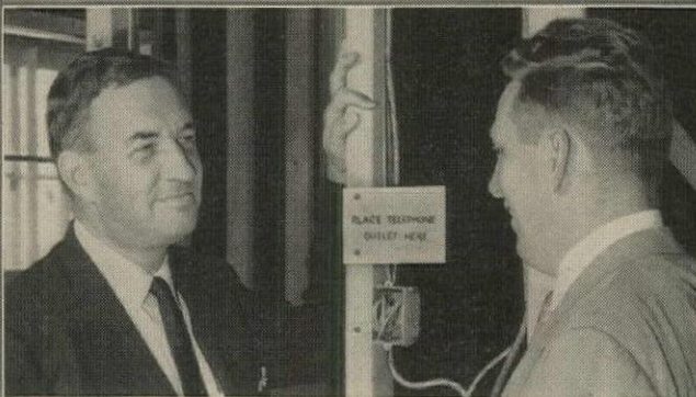
In an unfinished model, builder Bill Watkins discusses a kitchen phone location with telephone man C. L. Anderson.
