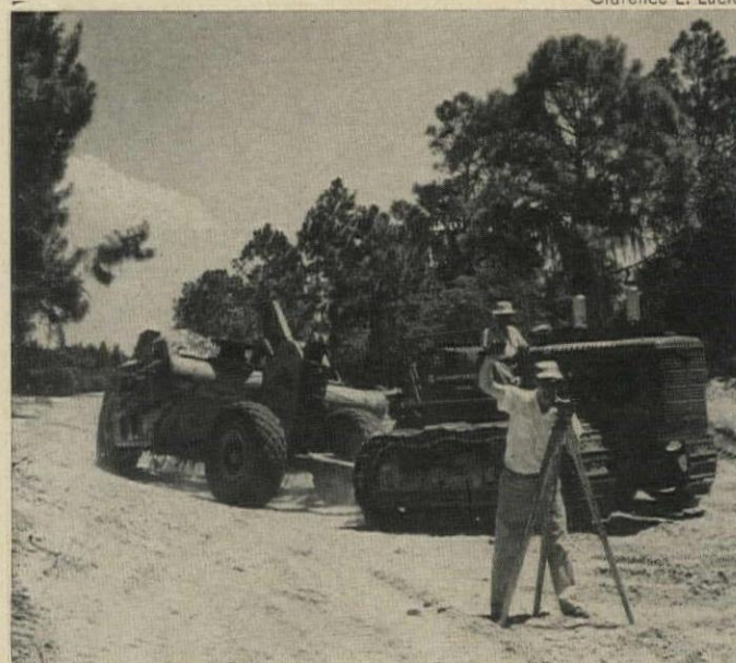
CURVED STREETS are carefully graded, have soil-cement bases. Most of tract was an orange grove and best trees are saved. Land at South Gate is high, did not require costly drainage installations.
