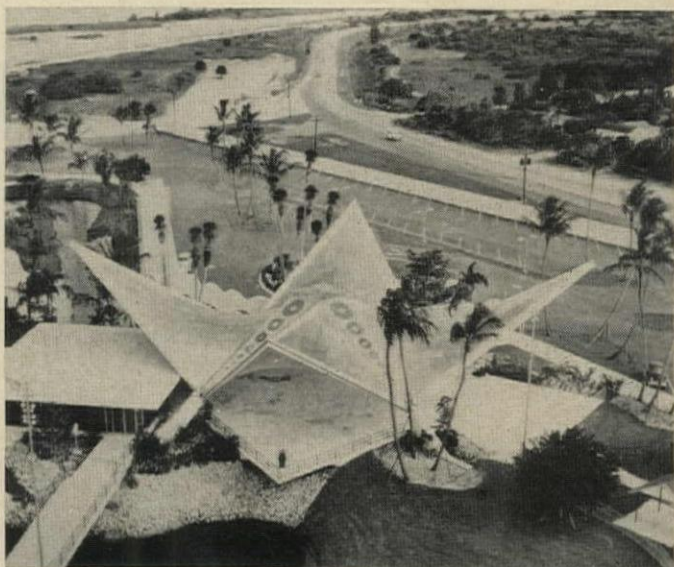
SALES CENTER with hyperbolic-paraboloid roof spanning 110' provides dramatic showcase for product display and sales offices at approach to model homes. Architect Charles F. McKirahan designed the pavilion.
