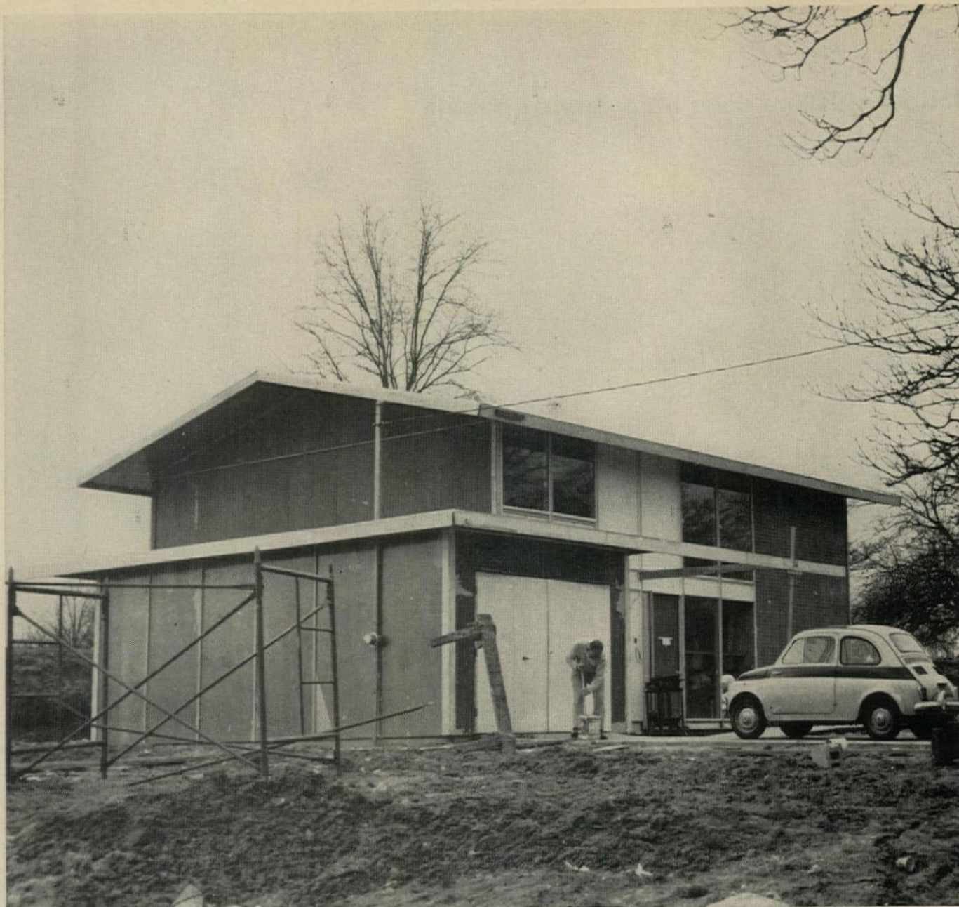
RESEARCH HOUSE gable-end panels are 4" thick, lap 3" wall panels to accent line. Triangular-top interior panels also support roof.
