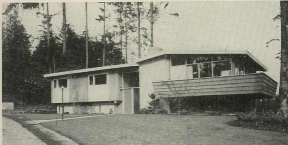
In Seattle , E.B. Vaughters built this $25,250 two-story house with a split-level entry from a design by Architect Seth M. Dulcher. There are 1,772 sq ft of living
