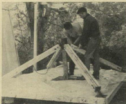
1 Paired 2x4 struts are bolted to panel, joined with welded connectors.
