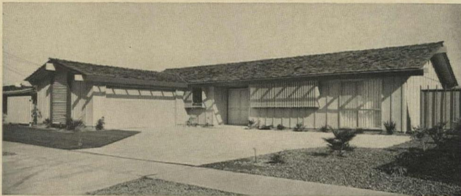
L-SHAPED HOUSE gets street-side protection from garage and fixed window shields. Living areas open to protected rear porch under main roof of house.
