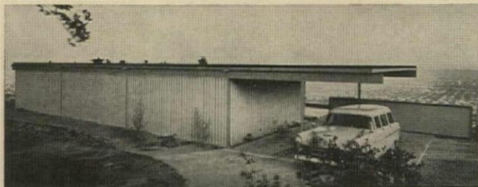
SOLID-FACED WALLS fronting street and carport are ribbed steel decking that repeat the roof motif. They have 2" of fiberglass insulation.
