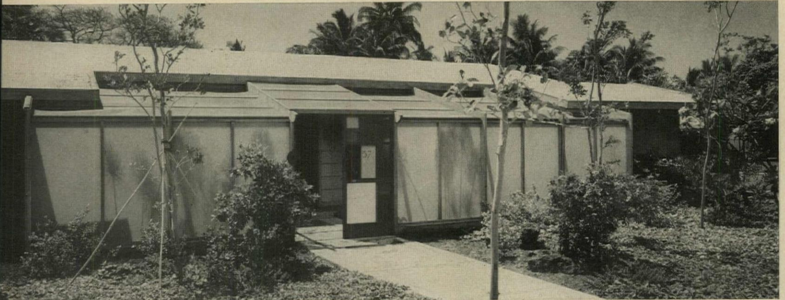
FRONT ENTRY, garden, and living room are shielded from busy street by obscure glass panels (see plan). Screened roof lets both sun and breeze filter in.
