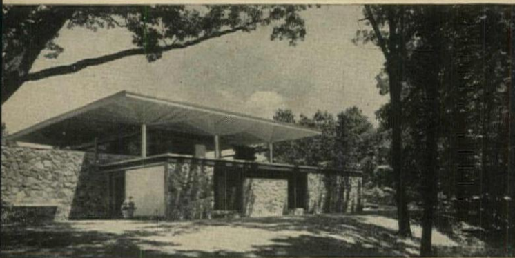
UMBRELLA ROOF over glass-walled second-story pavilion seems to float above fieldstone first floor.
