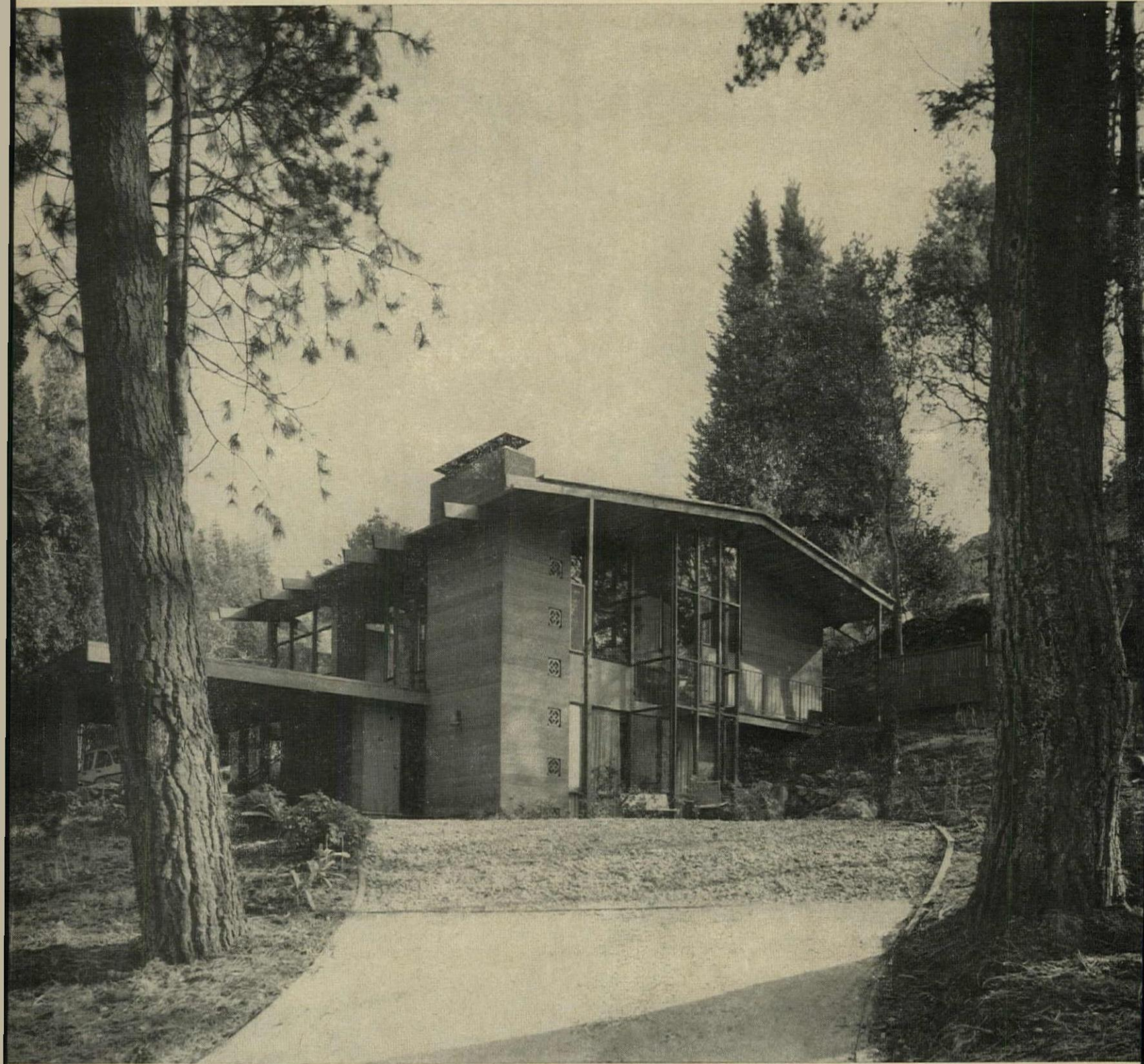
HILLSIDE HOUSE fits compactly into steep uphill site. Glass shaft in center extends through both levels, opens to walkway from living room to terrace.
