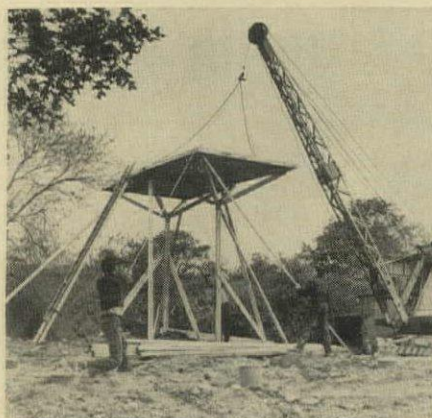
4 Crane erects umbrellas on circular piers where temporary bracing holds them.
