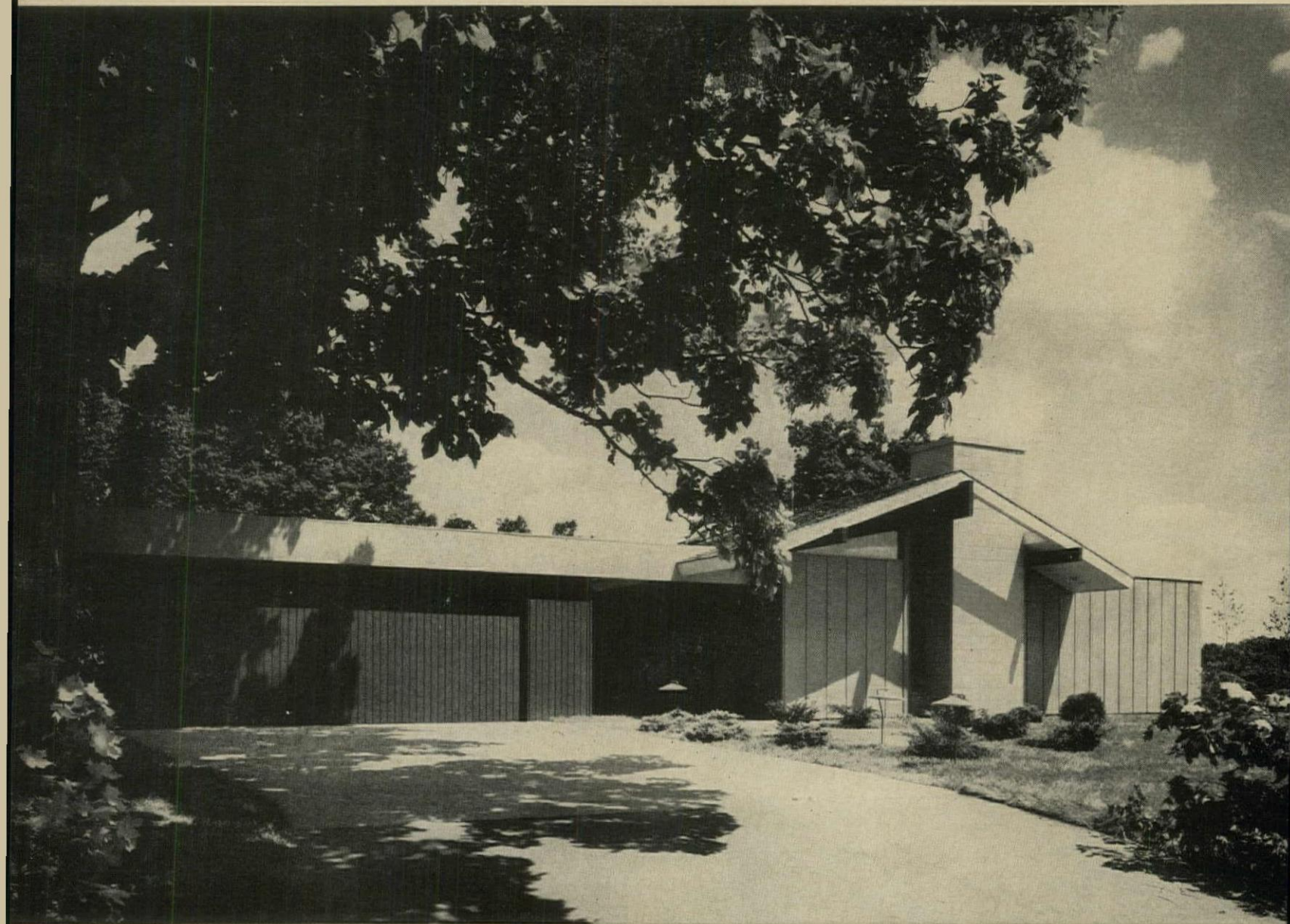
STREET SIDE of house presents an almost windowless facade—gains apparent size from the garage at the left and the extended wall of the house at right.
