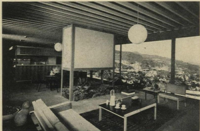
LIVING ROOM is separated from dining area by a freestanding fireplace-planter. Roof structure is expressed in exposed deck ribs everywhere but the kitchen.
