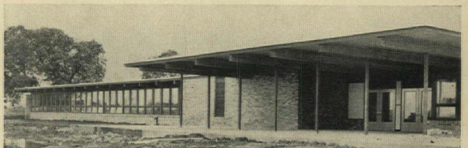
FINISHED SCHOOL has brick veneer, flat roof, sheltered entrance. Cost: $255,000.
