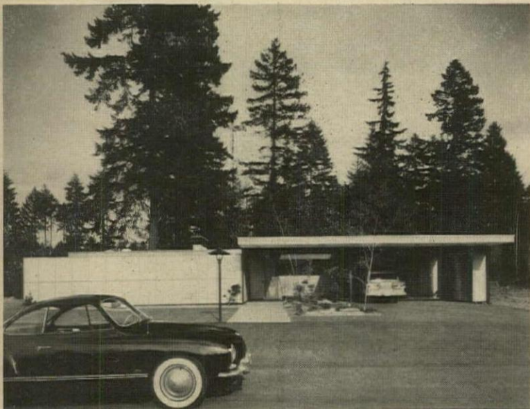
FRONT IS CLOSED by high patio fence at left and carport at right. Entrance is under carport roof in center, outside storage along wall at right.
