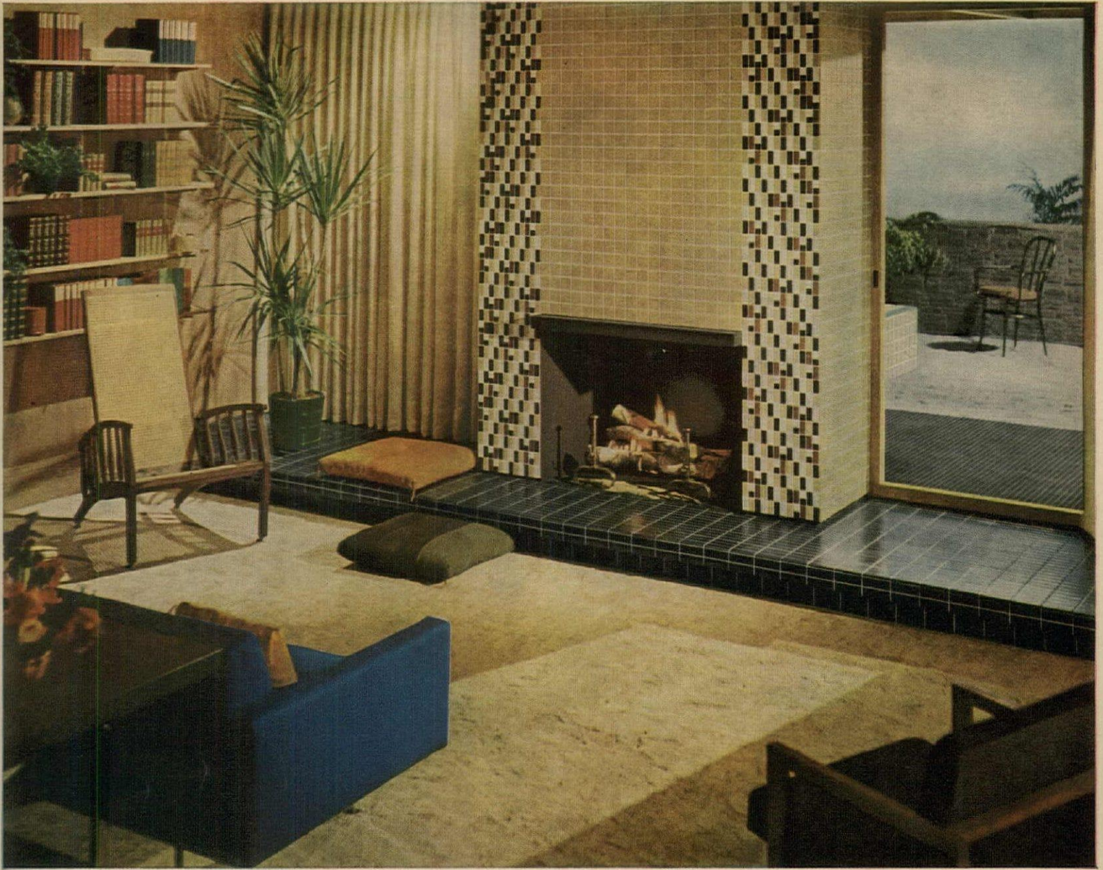
Tile Description: Chimney face and side wall in unglazed tile are 2\frac{3}{16} " squares, c.e. in Sand Gray Textone with special design of 1\frac{1}{16} " squares and 2\frac{3}{16} " oblongs, c.e. in Black, Sand Gray Textone, Rust Brown and White. Raised hearth is glazed Crystalline tile in Scored Design SD-4 in 362 Crystal Black. Color Plate 118.
