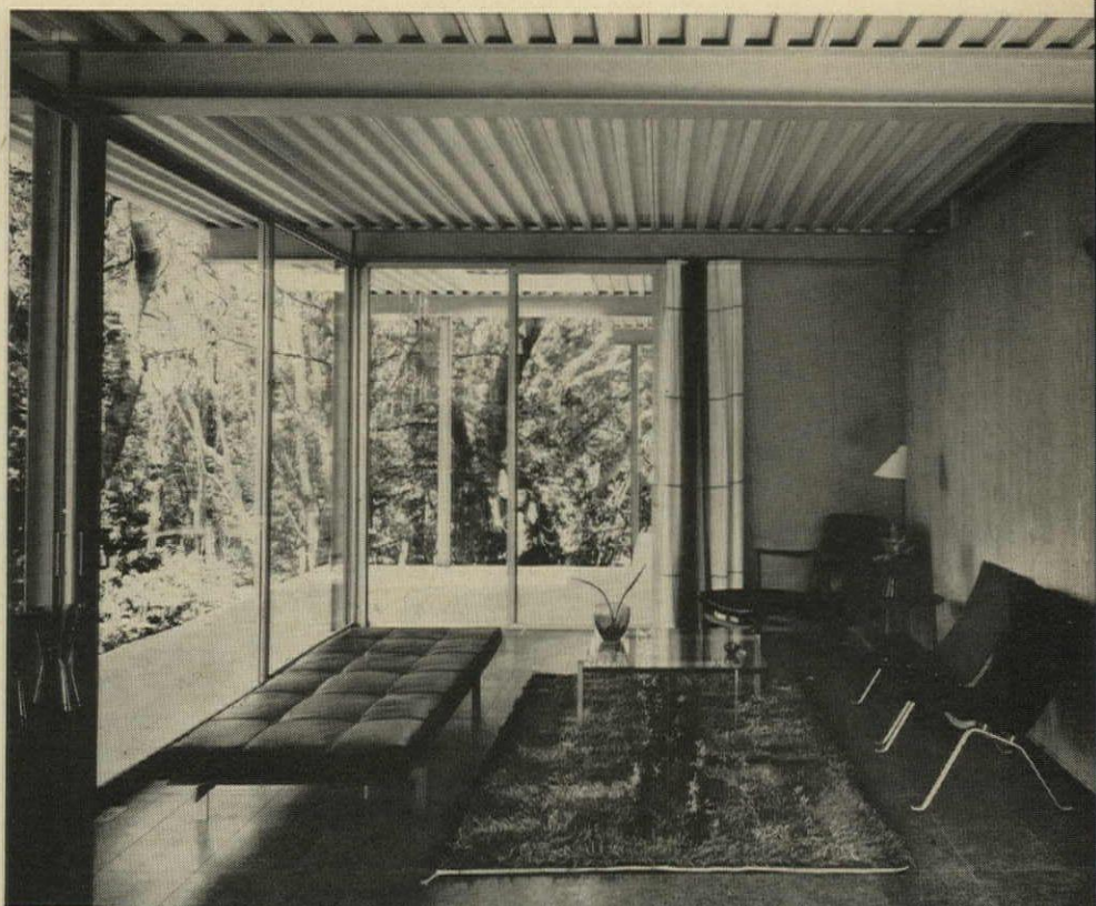
LIVING ROOM , to the east, is framed by L-shaped balcony. Wood wall, right, is light prefabbed partition that closes off kitchen. Ceiling is underside of ribbed decking.
