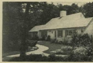
27. Architect Royal Barry Wills for a private client. p 144
