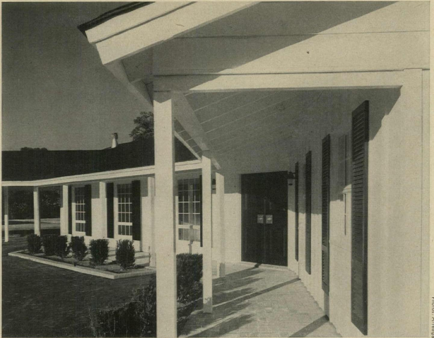
RAMBLING VERANDA gives shelter from carport to double-door front entry. Overhang is 7' wide, shelters deep windows from western sun.
