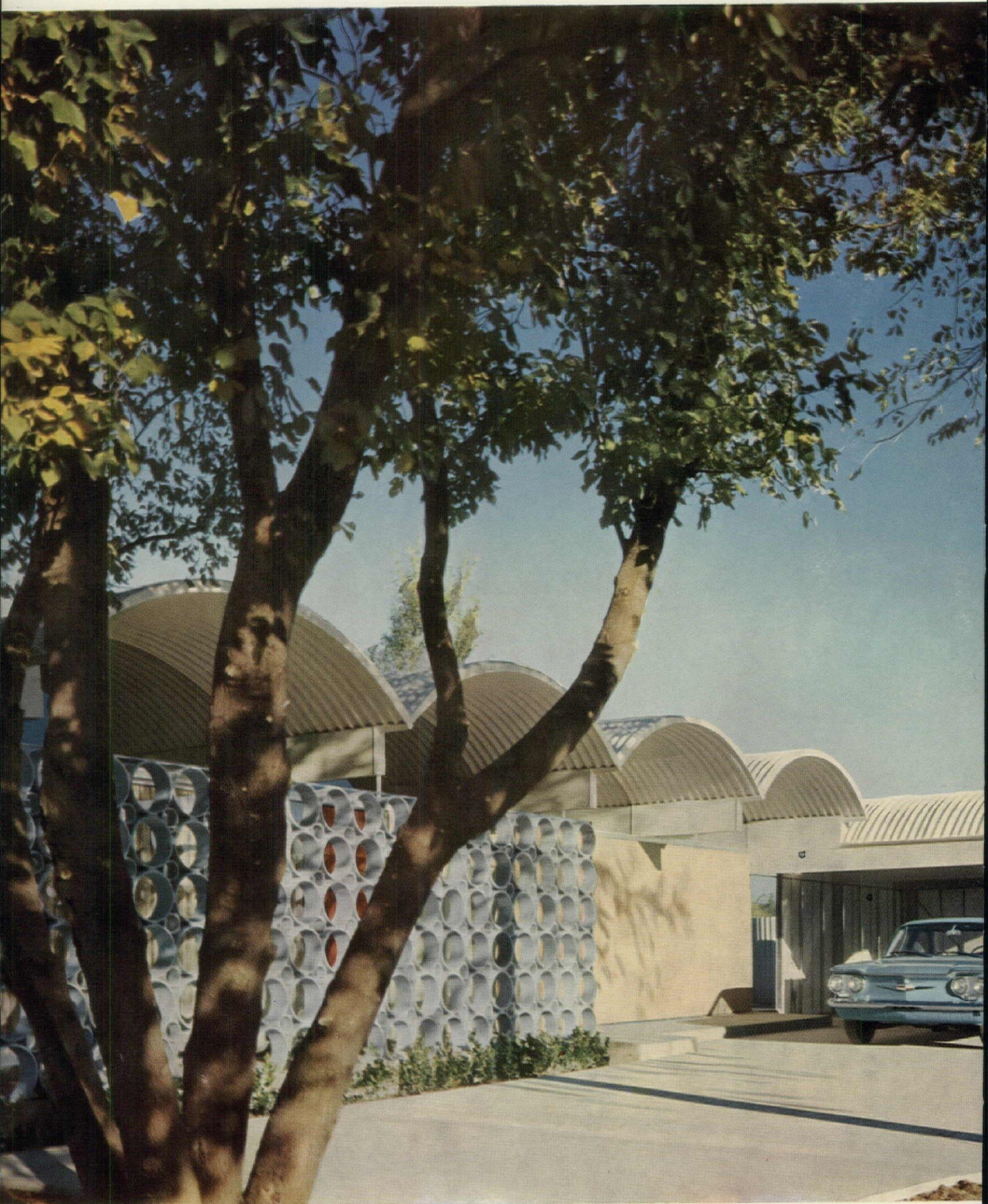
UNDULATING ROOF is made of corrugated asbestos-cement sheets with a 1" core of cellular concrete. Asbestos-cement pipe sections form screen at left.
