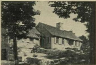
4. Architect Royal Barry Wills for a private client. p 114
