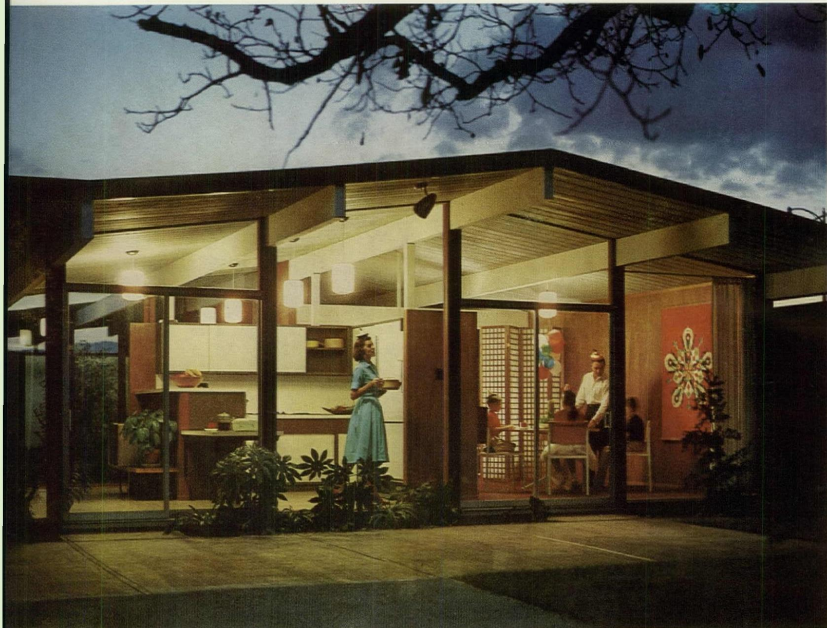
GLASS GABLE END opens family room, kitchen, and dining room to rear terrace enclosed by high fence (not shown). Inner court is through family room at left.
