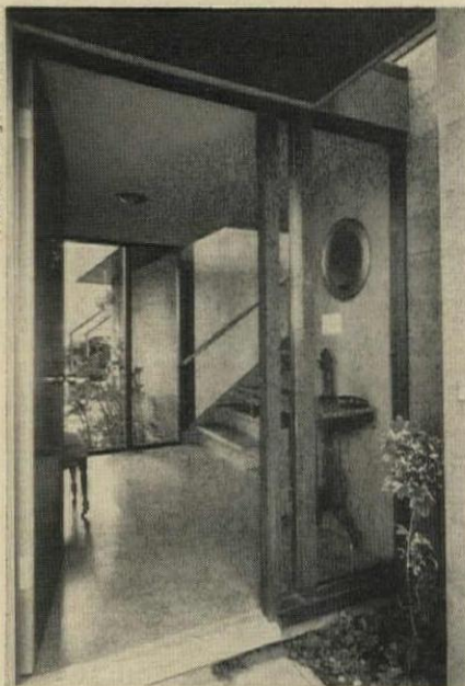
LIVING ROOM is on upper level. Walls, as in much of interior, are paneled. Roof deck is 2x6 t&g. Fireplace panel is gold leaf. Note break in glass wall for shaft.
