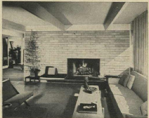
MASSIVE FIREPLACE adds balanced solidity to the otherwise open living-dining-kitchen space.
