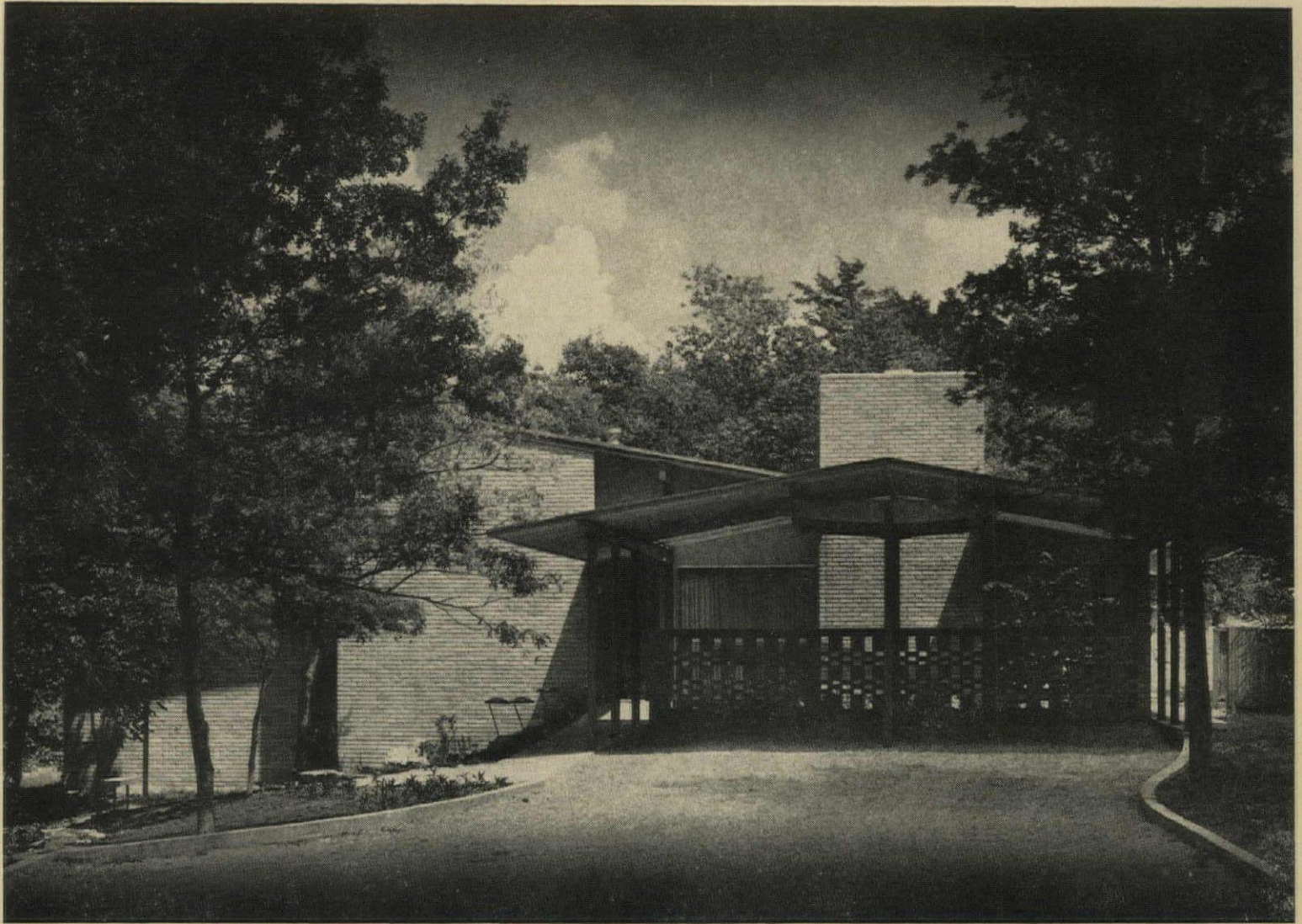
SIDE-BY-SIDE SPLIT uses brick in big easy-to-build masses, relieved by decorative handling of wood in carport. Entry is through garden behind carport.
