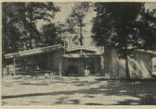
42. Architects Davis, Brody & Wisniewski for a private client. p 168
