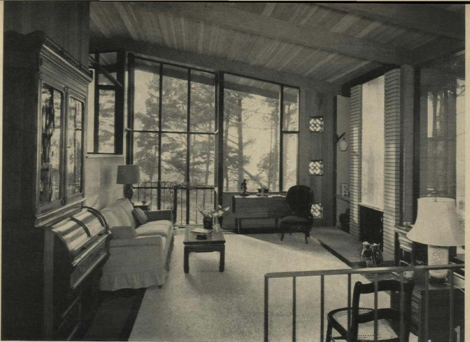
LIVING ROOM is on upper level. Walls, as in much of interior, are paneled. Roof deck is 2x6 t&g. Fireplace panel is gold leaf. Note break in glass wall for shaft.
