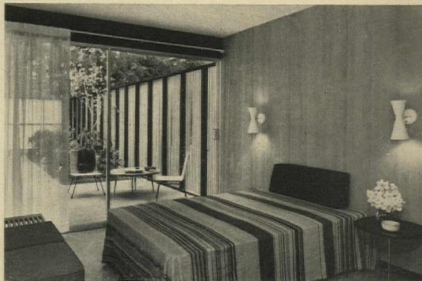
MASTER BEDROOM opens to terrace through sliding glass doors. Paneling on wall at right is 1x4 rough sawn cedar; fence outside doors is 1x1 cedar slats in redwood frames.
