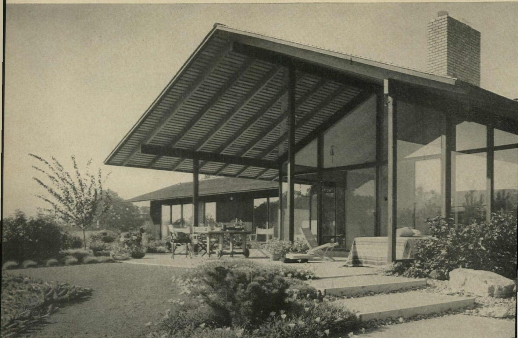
GABLE OVERHANG runs 15' beyond front wall. Texture on underside is strip sheathing for cedar roof. Glass panels on right keep out northerly winds.
