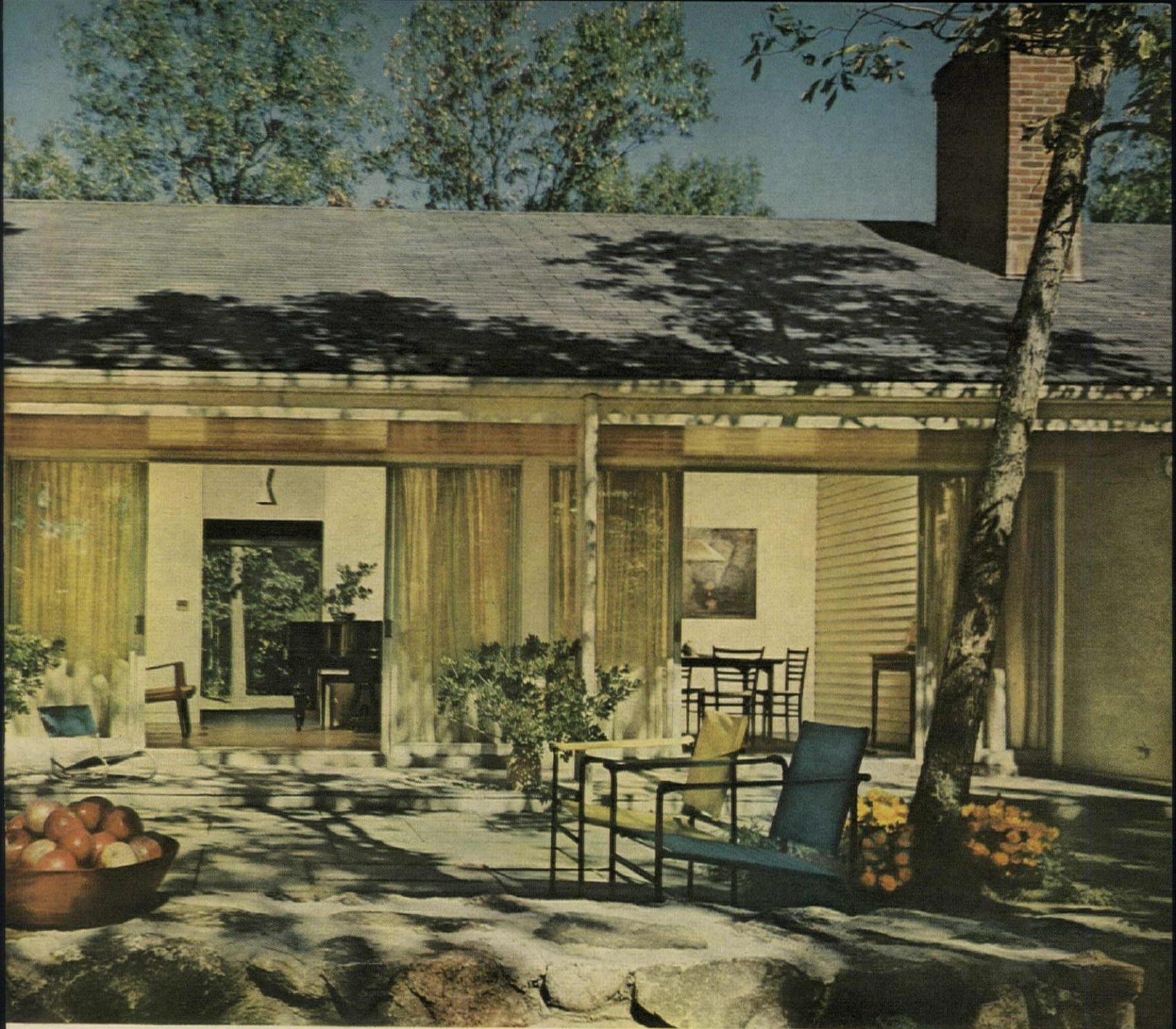
CONTEMPORARY REAR ELEVATION has sliding glass doors that open length (33½') of living and dining rooms to 5'-deep veranda and terrace in foreground.
