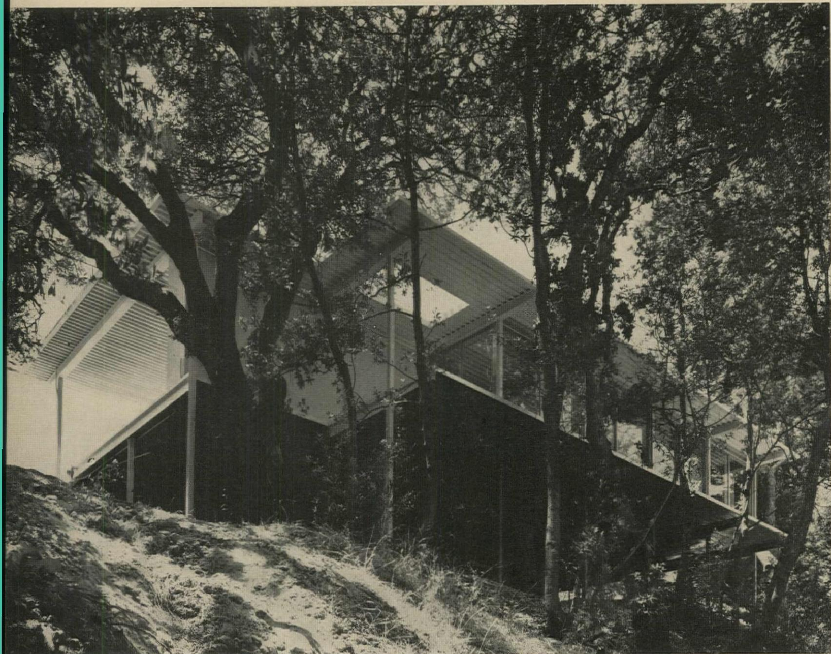
LIGHT STEEL CAGE rides high over a steep slope so living areas look out into tree tops. Deck and roof cantilever to form shaded balcony.
