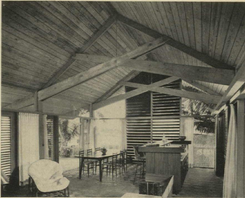
EXPOSED SCISSORS TRUSS adds cooling height to indoor living areas, continues past walls to shade decks. Big beams taper to reduce weight at outer ends.
