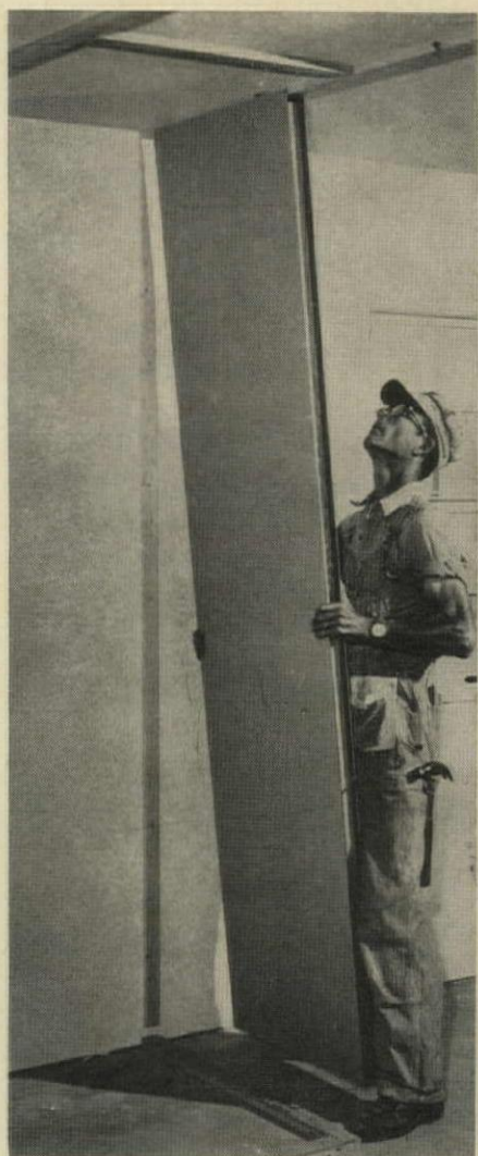
FIRST PANEL (2'x8') is slipped over ceiling runner, positioned on floor runner, and slid over wall runner. Top is secured with finishing nails, bottom with anchoring nail through lip at corner of frame.
