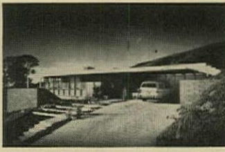
16. Architect Carl L. Maston for a private client. p 126
