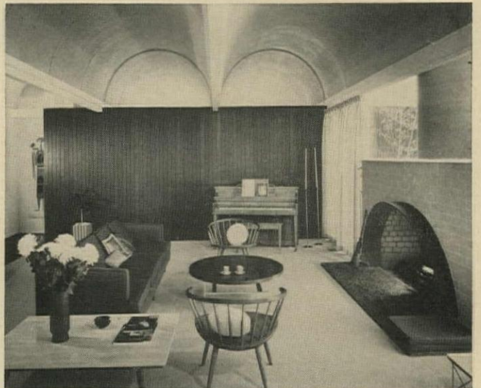
LIVING ROOM ends in a wall of U-grooved 1x3 fir, stained dark walnut. Arched fireplace lintel is bent 1/4" steel plate.
