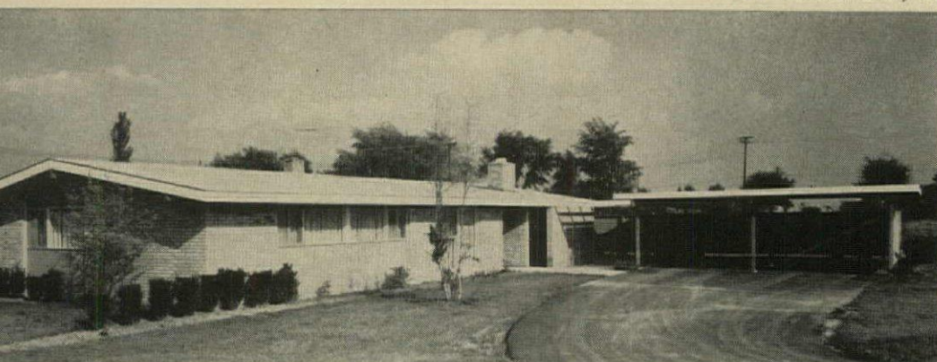
RANCH EXTERIOR alternates brick with door and window panels. Plan opens living room to terrace; kitchen and family room share second outside living area.
