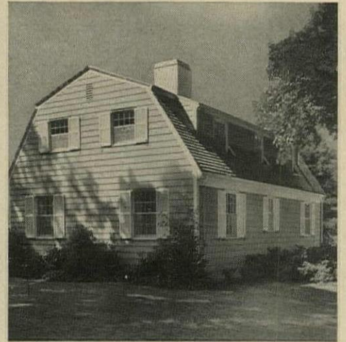
GAMBREL-ROOF HOUSE has scale of a cottage—but over 2,600 sq ft of living space. Often-overlooked roof type is pleasing—but adds to cost of framing.
