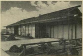
12. Architect Edward H. Fickett for Severin Constr, builder. p 122
