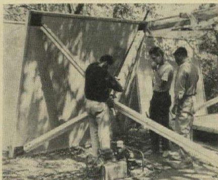
2 Umbrella panel is tipped up, double 2x4 post is bolted into center connector.
