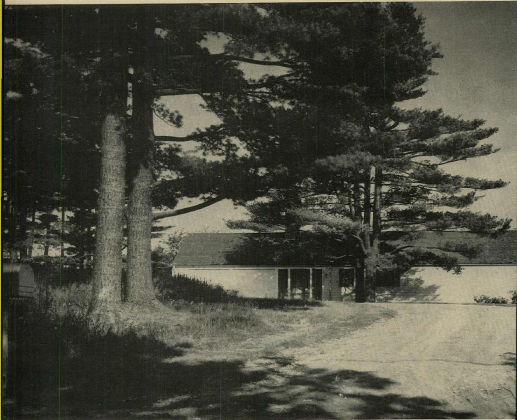
LOW AND RAMBLING HOUSE with classic New England lines stretches 110' and fits its site like an early farm house.
