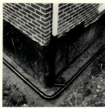
**New downspout** and drainage pipe uses a tapered fitting and a square-cut pipe end. There is no retooling of cut pipe ends. Fittings are driven on to form waterproof joints. This lightweight bituminized pipe comes in 10' lengths and in 3", 4", 5", and 6" diameters.
