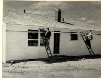
REPUBLIC HOUSE-LONG "K" GUTTERS cut installation time in half. Lengths up to 32 feet. No soldering, no joints to line up. No seams to mar appearance. Go up easy, fast, at a profit. Use coupon.
