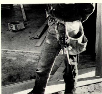
QUICK-DRAW NAIL POUCH, substituted for nail apron as result of study, is easier to get at when carpenter bends, kneels, or stoops.
