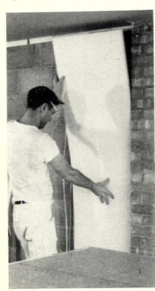
STEP ONE: Apply adhesive-coated Styrofoam insulation directly to masonry wall.
