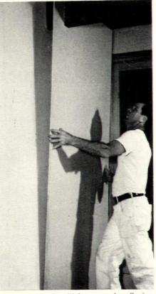
STEP TWO: After 24 hours, apply adhesivecoated gypsumboard to the insulation.
