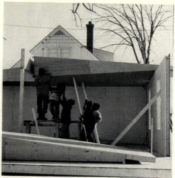
**ROOF GOES UP** in 4'x14' sections, is tied into box beam at ridge. Top of roof section becomes roof deck, bottom is finished ceiling.
