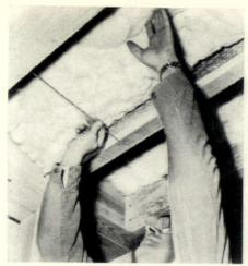
**Tiger Teeth** are sharpened heavy steel wires that jam between joists to hold crawl space or ceiling insulation in place without stapling, chicken wire, or nailer strips. Savings of as much as two-thirds of installation labor are reported.
