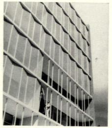
**SCREENING** is held in aluminum frames fastened to staggered mullions.
