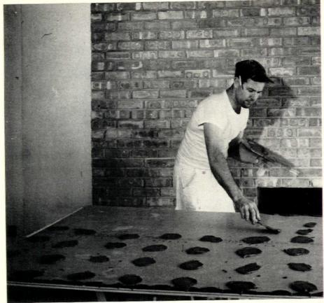
gypsumboard 8" oc. Styrotack grabs fast and can be shifted for final adjustment.
