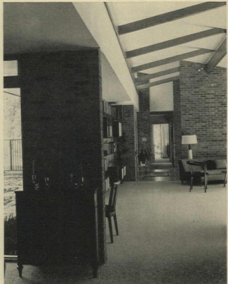
Main living area has high beamed ceilings, massive brick divider walls, and a long vista down the gallery from the dining area to the master bedroom.
