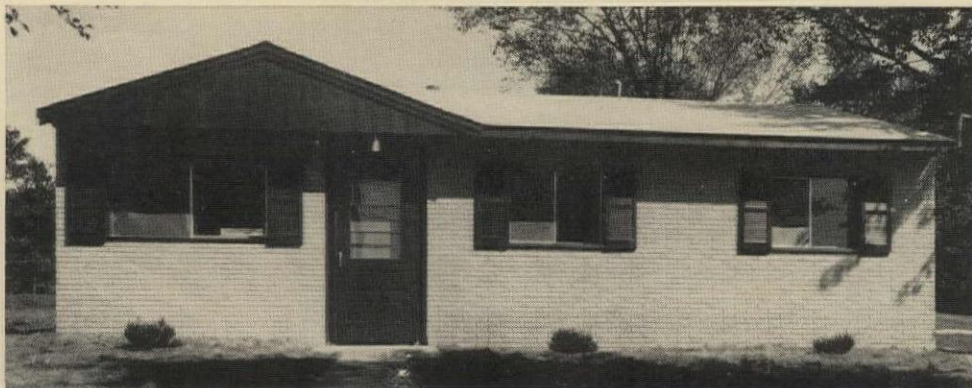
FOAMED-CONCRETE HOUSE , built by Frank Paxton Lumber Co., is 24'x36' and has three bedrooms.
