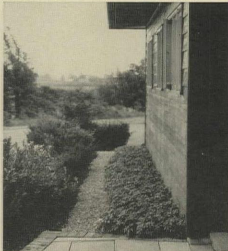
GRAVEL STRIP below roof drip line (where there are no gutters) reduces wash-out of plants.
