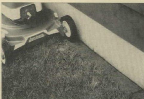
BRICK EDGE along planting beds, gravel drives, or walks makes power mowing a faster job.
