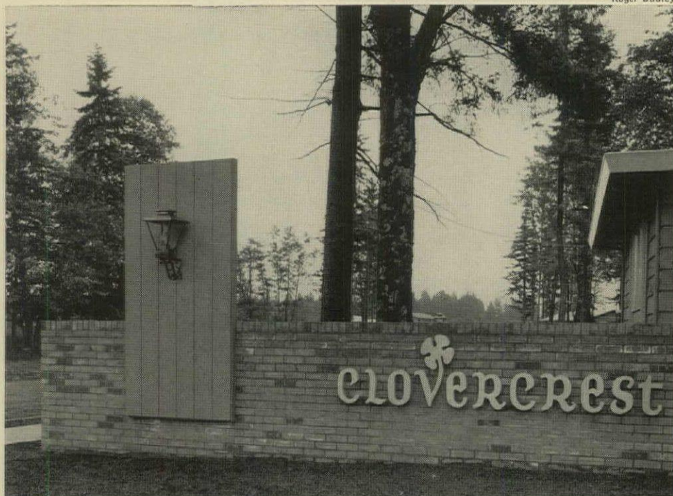
COMMUNITY ENTRANCE cost $612 (including brickwork). Cost was allocated to community de-
