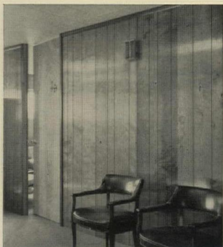
PREFINISHED WALL PANELS and ceiling-high prefinished doors are used throughout house.
