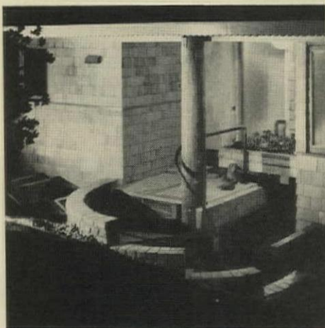
Structure of posts and beams is clearly expressed. Walls are set behind posts to avoid complicated (and hard to waterproof) connections.
