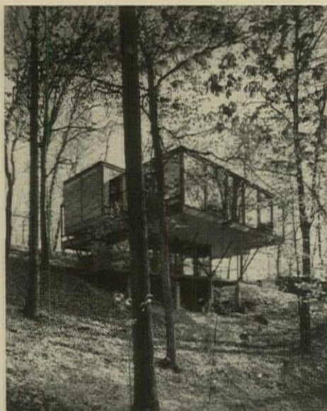
On downhill side, house seems to float above the site. Wall panels are glass or walnut siding.
