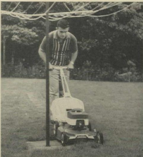
FLUSH PAVING around clothes pole and other obstructions eliminates grass trimming by hand.
