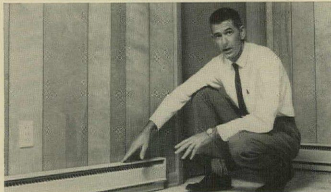
COMPACT ELECTRIC BASEBOARD UNITS were chosen by Bill Rowland for his new homes to help him cut construction costs. Because they are quick and easy to install, they save on time and labor.
