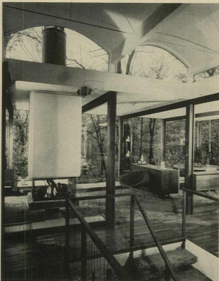
Living-dining area has all-glass walls on three sides, and a striking treehouse view. Posts maintain 12' module used everywhere in the design.
