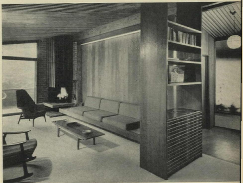
In living area, strong textured ceiling (laminated of alternate 2x3s and 2x4s) and wood paneling create a feeling of warmth and shelter.
