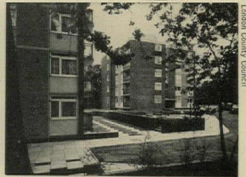
3. Apartments in London.
