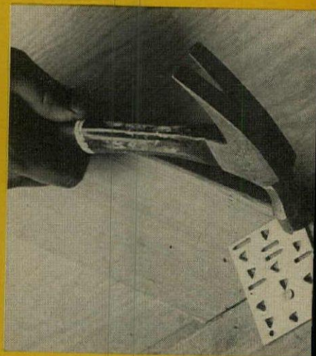
Reassembly of knocked down trusses requires only a hammer. The tough fibers of West Coast Lumber provides holding strength for connector teeth.
