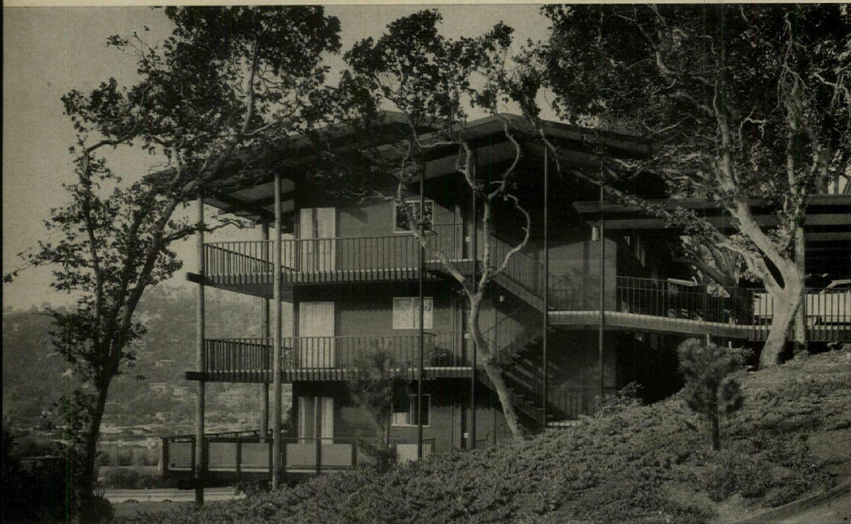
Carport platform bridges the slope between the driveway and outside entry stairs at midpoint of the living levels. No entrance is more than 1½ stories from carport grade. Wrap-around balcony has views in several directions.
