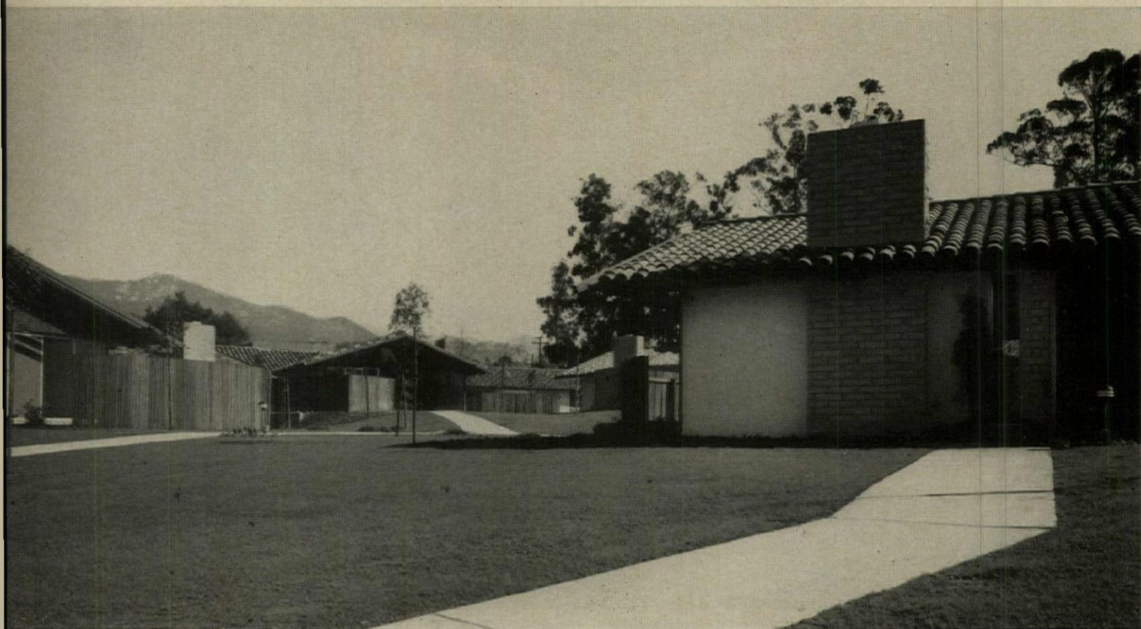
Greens and commons between buildings emphasize the openness and park-like atmosphere. They afford a view of the mountains and wooded slopes that surround the city. Power and phone lines are underground.
