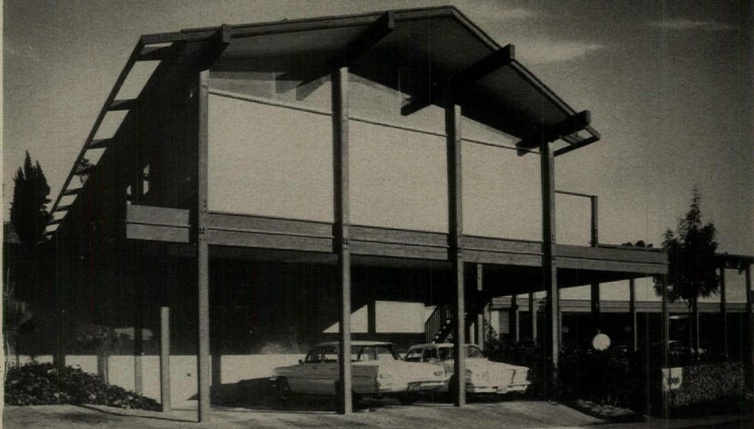
End wall presents an almost solid facade to the roar of traffic from a nearby freeway. Wall panels are plaster. Post-and-beam members are bolted. Wall extension at left screens patios of ground-floor apartments.
