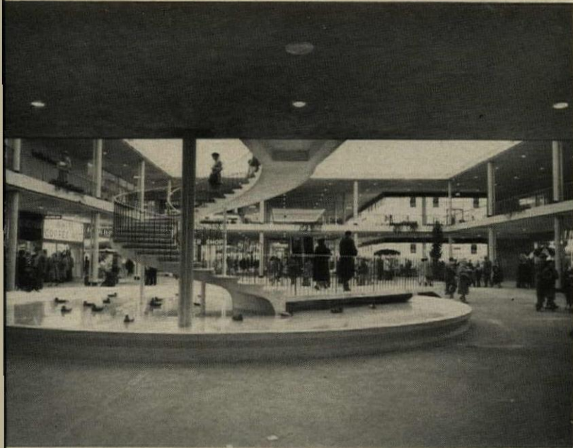
Mondawmin—a highly successful shopping center in Baltimore—was designed by a team of architects including Pietro Belluschi. "Architecture is our big extra pull," says Developer James Rouse.
