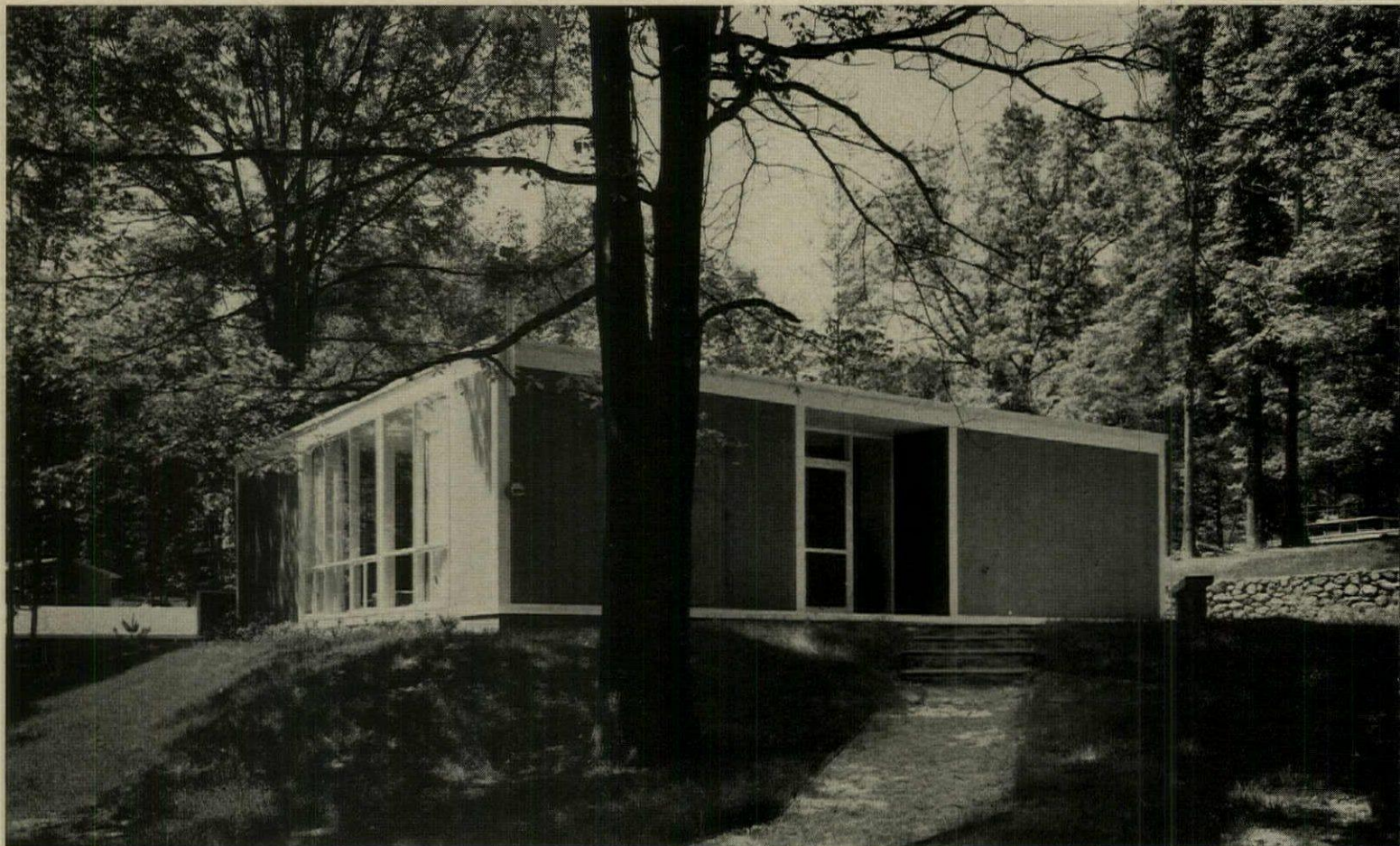
In Alexandria, Va., Builder Robert C. Davenport introduced this $16,500 house designed by Charles M. Goodman Associates in 1953. Result: ten sold in six weeks, with FHA financing.
