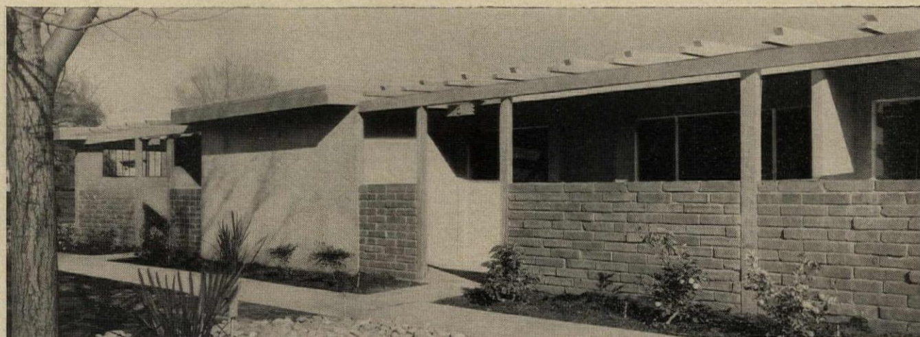
River College Manor Apartments, Sacramento, California. The first unit of 32 total-electric apartments was eighty percent rented three weeks after completion. Construction is
