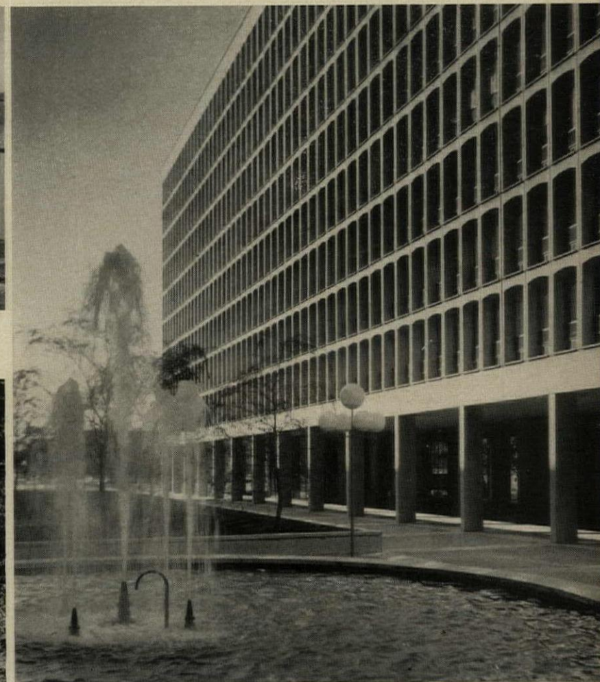
Apartment in Webb & Knapp's Hyde Park project in Chicago has remained fully rented "after a start slowed by a fringe location." Architects: I.M. Pei & Assoc. with Harry Weese & Assoc.
