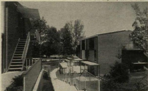
Outdoor structural components—fences, trellises, and sunshades—are steel. Brick-and-block end walls and foundations are only conventionally built elements in the apartments.
