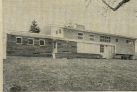
IN OHIO: "Our carpenters like to work with it." Sims Bros. Inc., Marietta
