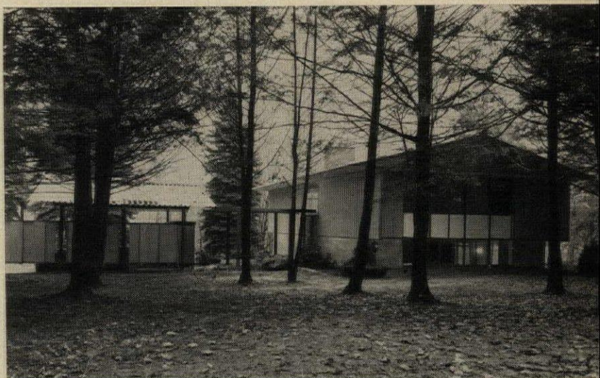
Steel research house, sponsored by Techbuilt and Armco Steel, and designed by Carl Koch, was built to test mass-produced components. It will soon be offered as a package by Techbuilt.
