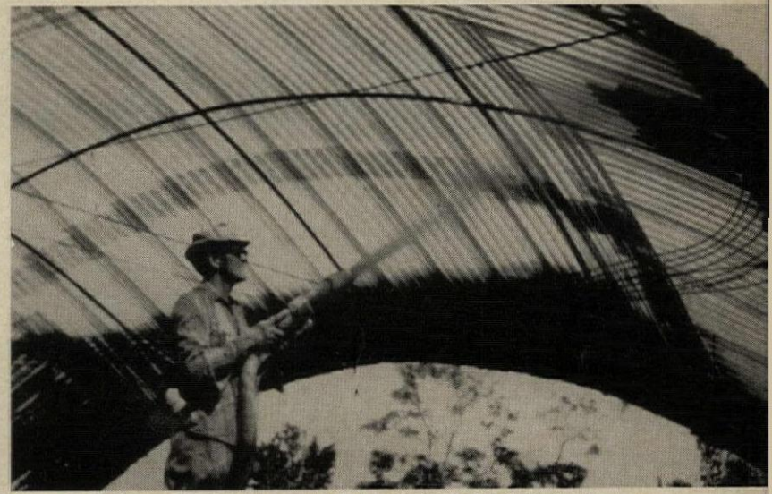
SPRAYED CONCRETE clings to metal lath and rings of reinforcing bars, at right, supported on tubular framework. Spraying time: 24 man hours.
