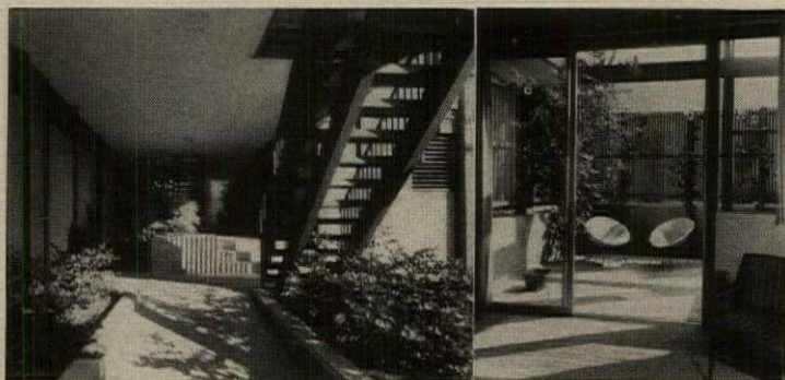
Protected passageway is entered by ramp (foreground of left photo), leads to ground-floor apartment and stairs to second floor. Each apartment has a private terrace (right) or deck screened by wood slat fences or solid panels.
