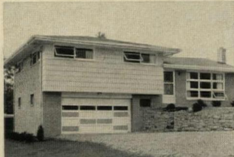
IN PENNSYLVANIA: "Saws in any direction . . . goes up with no splits or cracks." Colosimo Construction Co., New Stanton
