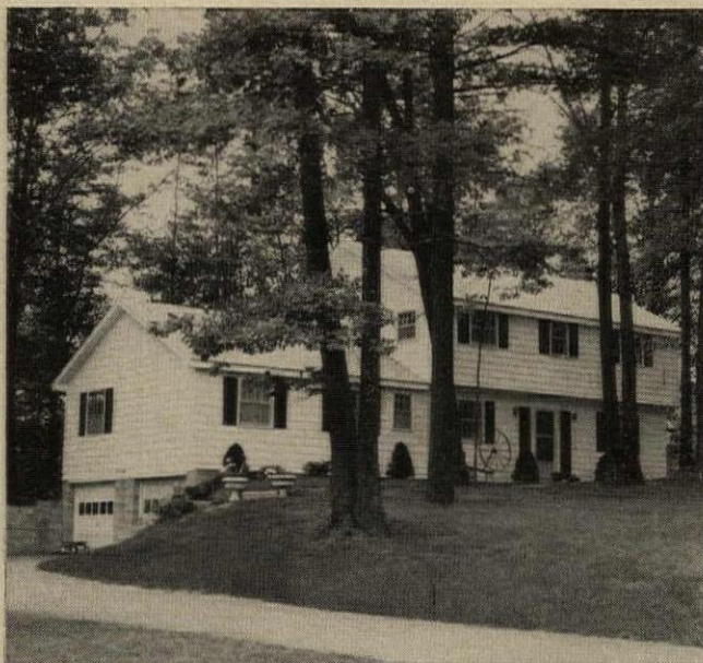
Clifton Knolls, Schenectady, N.Y. In the midst of a severe cold climate, these total-electric homes are kept warm with General Electric baseboard electric heat. Builder R. Van Patten says "... my buyers love it." 130 Gold Medallion homes are already sold; and another 500 are planned.
