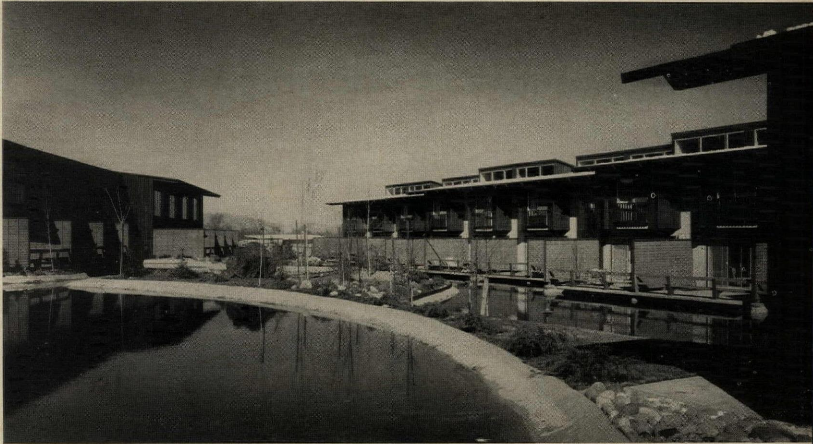
Lagoon flows beneath the edges of concrete decks, which have built-in perimeter seating as a protective barrier and wood screens for privacy between the decks. A pump recirculates water from on-site well through the lagoon.
