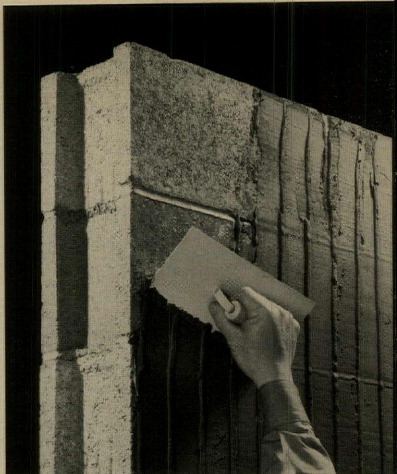
2. Start with Styrotac® bonding adhesive.
