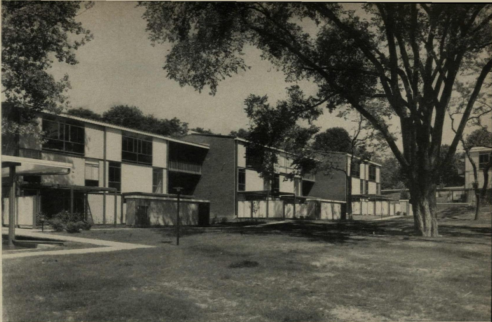
Staggered buildings face onto wooded commons, are set 20' apart for maximum privacy and cross-ventilation and connected by a covered deck that serves as a balcony for the third-floor, single-level apartments.
