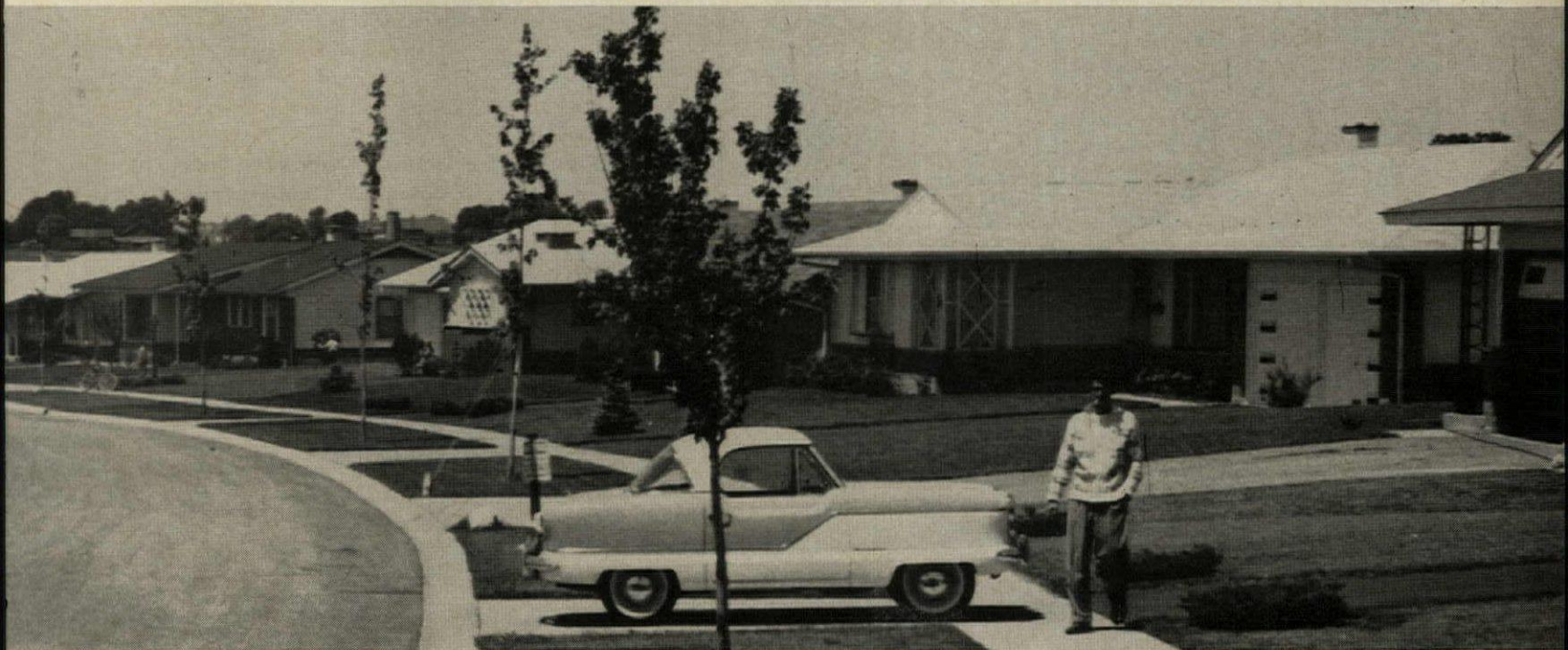
UNCLUTTERED STREETScape is at Centex Corp.'s Elk Grove Village where Commonwealth Edison put wiring underground for less than $100 per lot.
