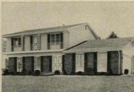
IN OHIO: "Reversible edges help us eliminate waste on gable ends." Smith-Kettler Bldrs., Inc., Cincinnati
