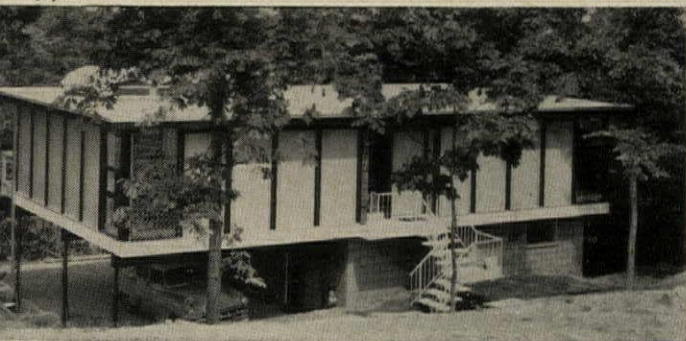
Another example of modular design: Alcoa's Alply panel house built by Pittsburgh Builder Thomas Douglas, designed by Paul Freeman. Contract price of the 1,700 sq. ft. house: $20,500.
