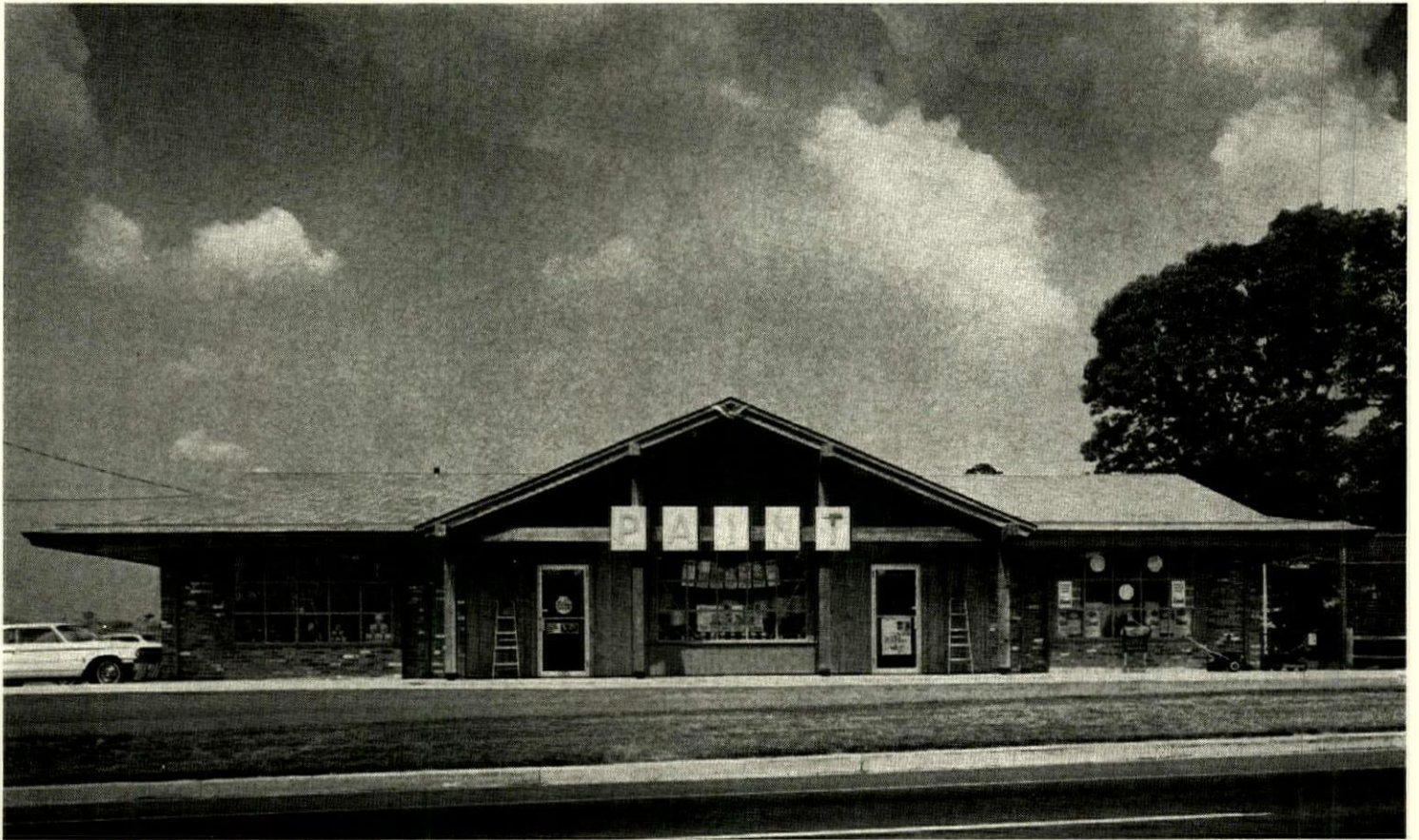
DESIGN of the "Home Beautiful Center" is deliberately house-like, and the finish is traditional board-and-batten with old brick.
