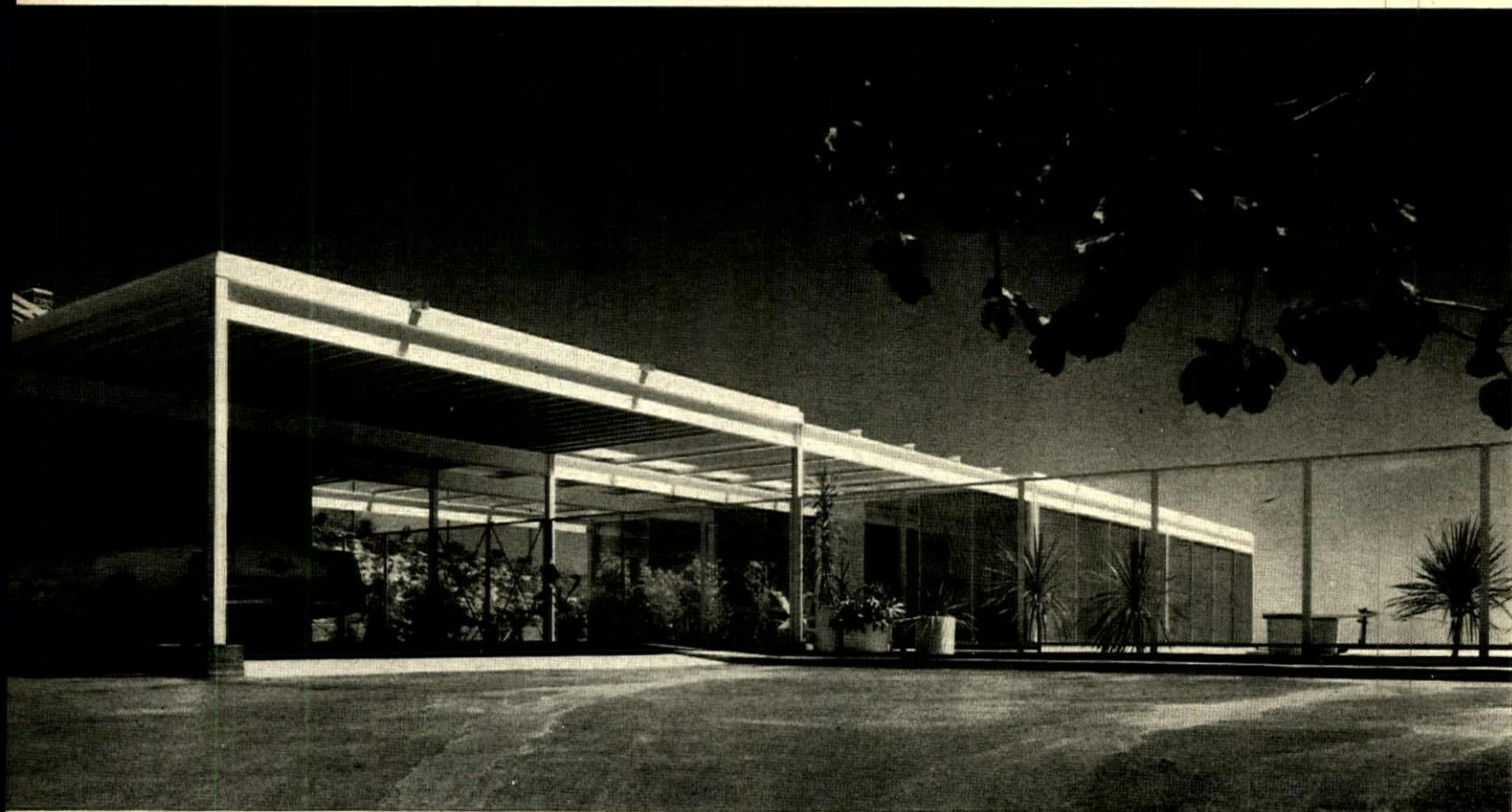
Simple framing shows clearly in the view from the street, with I-beams running the 92' length of the house. Storage, heating, and laundry facilities are housed in the steel-walled structure at the rear of the carport.
