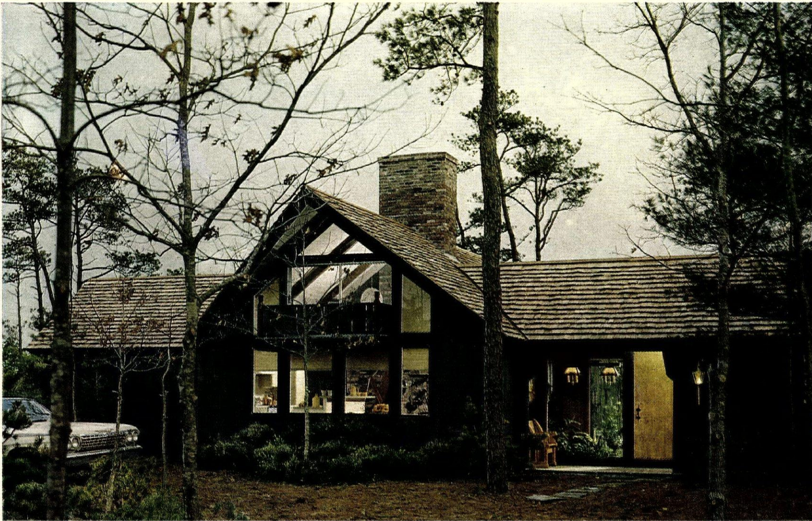
FRONT VIEW shows how architects used Cape Cod forms in a contemporary design, created a feeling of elegance with rustic materials (cedar shake roof; stained, rough-texture plywood siding).
