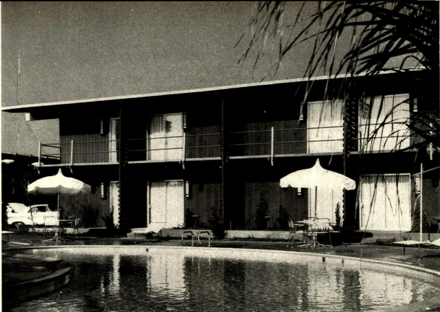
TYPICAL UNIT has eight rooms, is framed like a two-story house. Exterior finish is stained redwood, which needs no maintenance for years.
