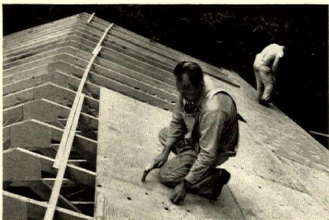
It takes about four man-hours to apply plywood roof sheathing to one of Mitchell's compacts. House on this page has 1,008 sq. ft. and sells for about $70 a month on buyer's lot. Mitchell offers dozens of variations in size, style, features. This model, the "Holly," designed by Robert Bruce Waring, is one of 12 plans available to builders under DFPA's Compact Homes program.
