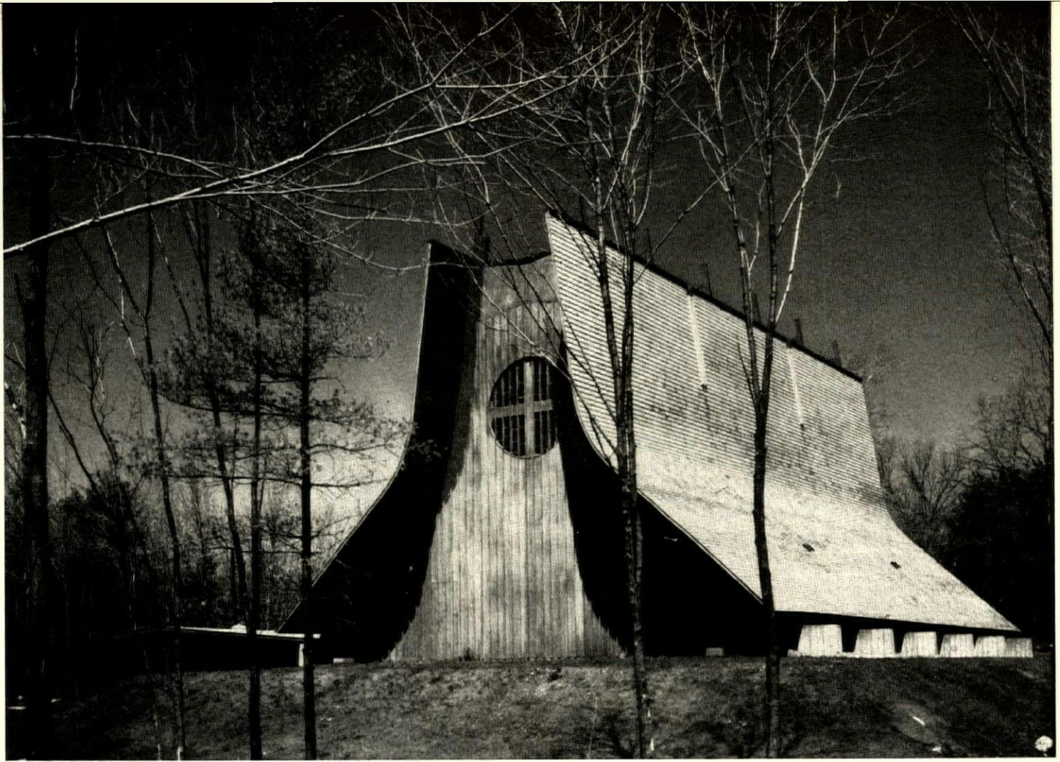
CURVED ARCHES give the church its basic form. They sit on concrete pillars, visible at right, and their ends project above the roof.
