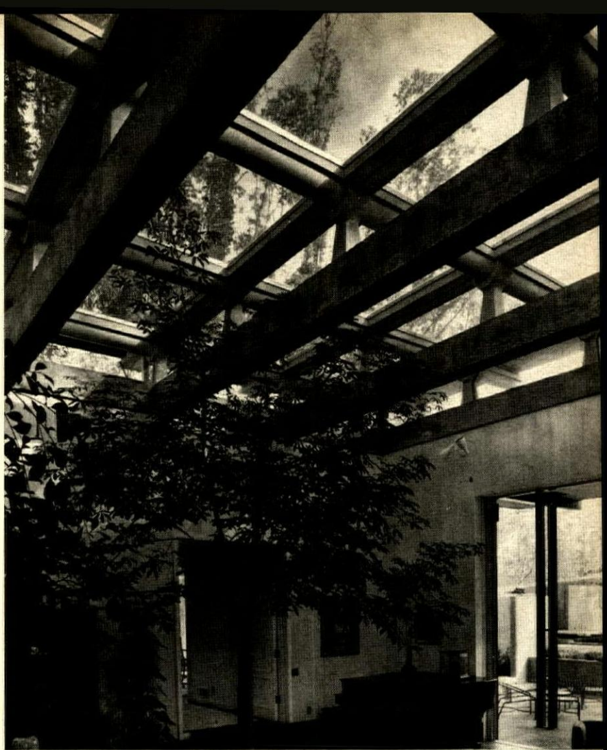
In patio-solarium, double dome skylights are supported on precast concrete units that act as supports, skylight curbs, and roof gutters. Clear plastic hopper windows just below the ceiling help ventilate the court.
