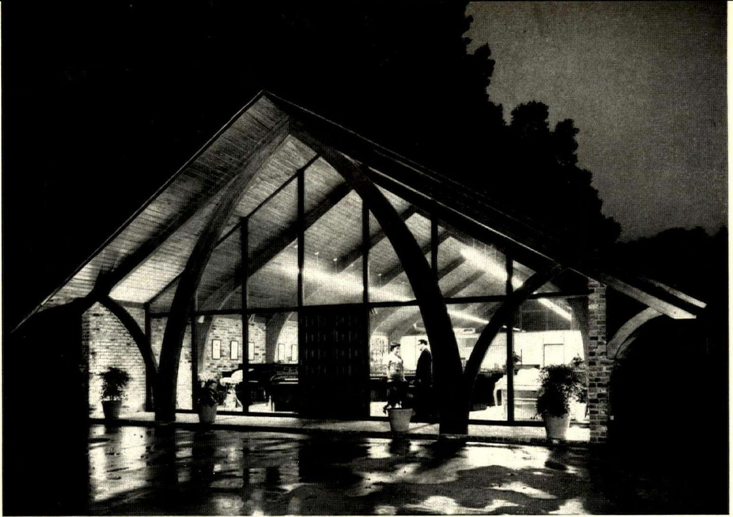
SPACIOUS FEELING of music store is augmented by glass end wall that rises to roof. Like bents inside, arches are laminated pine.
