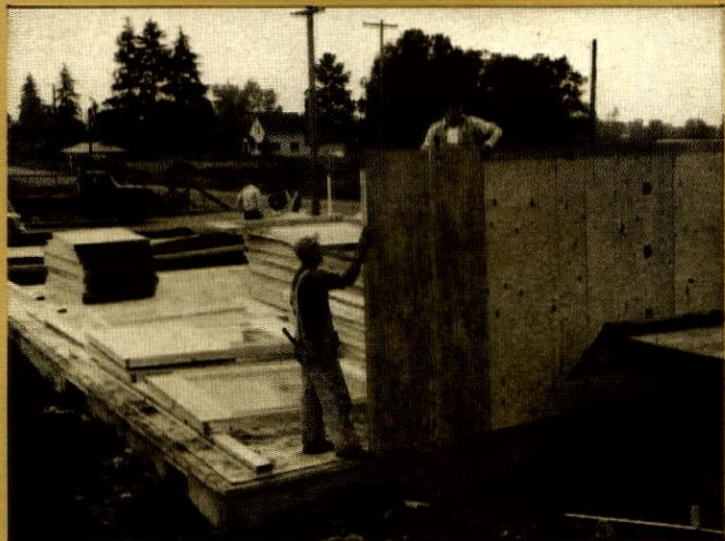
3. Wall components for this M/P model have plywood sheathing on studs; siding will be applied later. Components are stacked on the floor platform near where they'll be used.
