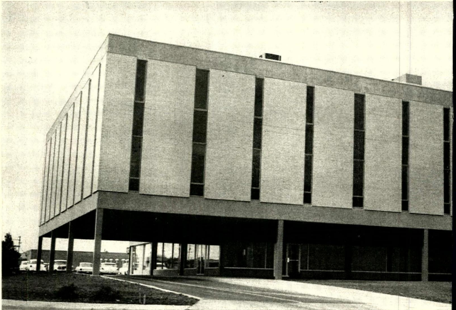
STRIKING DESIGN is achieved by alternating panels of brick with strips of glass. Steel columns support offset upper stories.
