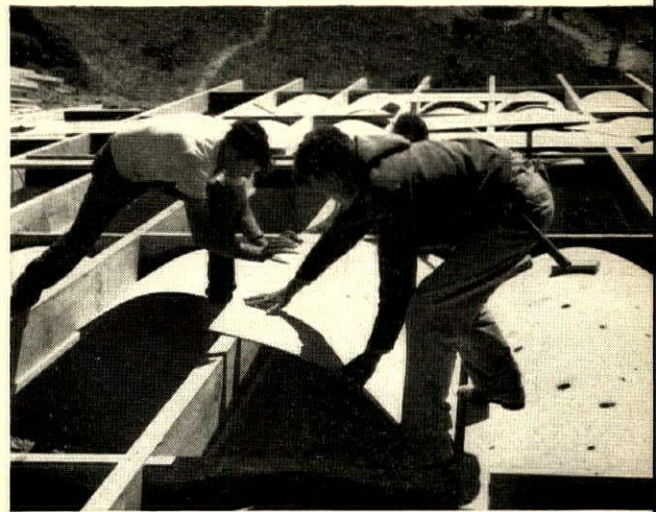
Curved plywood soffits conceal pipes, wiring and insulation under the floor. Pre-painted panels of 1/4" EXT-DFPA plywood were sprung between 4x12 framing. This is an easy way to conceal the clutter under a hillside house. The heating and cooling system are also out of sight, in the attic plenum.
