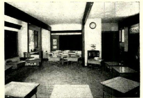
TYPICAL CLASSROOM has sand-finished plaster walls, cheaper here than drywall because it could be left unpainted. Flooring is asphalt tile.
