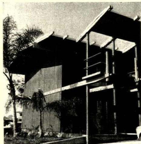
END WALL of unit is blank to block traffic noise. Canopy at right adds design interest, covers the walkway to the parking lot.
