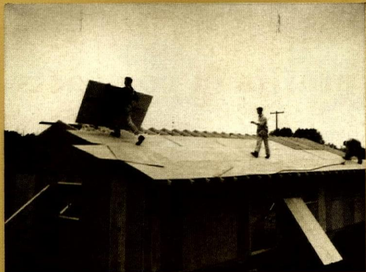
6. As soon as roof sheathing is on, the house is enclosed and doors can be hung. Interior work—which uses as many prefinished parts and materials as possible—can start any time. It's 1:30.
