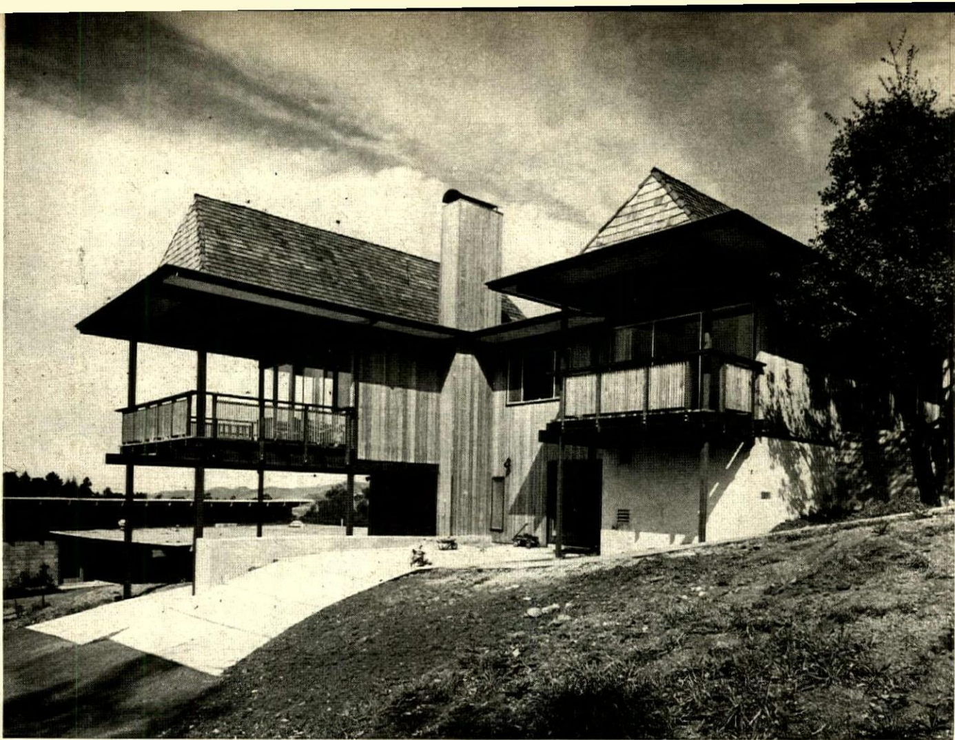
Generous open porches face the view, are accessible through sliding glass doors. Wide soffits, with tension cables at each end of the rooms, contain the thrust of the pitched roof, which has no collar beams.
