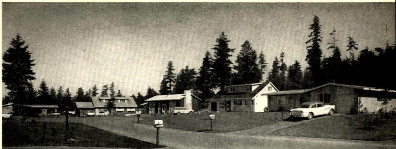
Most Mayer/Peterson houses are between $10,000 and $17,000 and are in medium-sized developments like this, a group of 17 near Lakewood, Washington. Most of these were sold before completion. All houses use plywood component systems, but vary widely in siding and architectural styles ranging from ranch to colonial (below).
