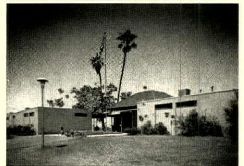
STREET SIDE of club has almost solid block walls. Pro shop, focal point of design, is set back to create an entry court.
