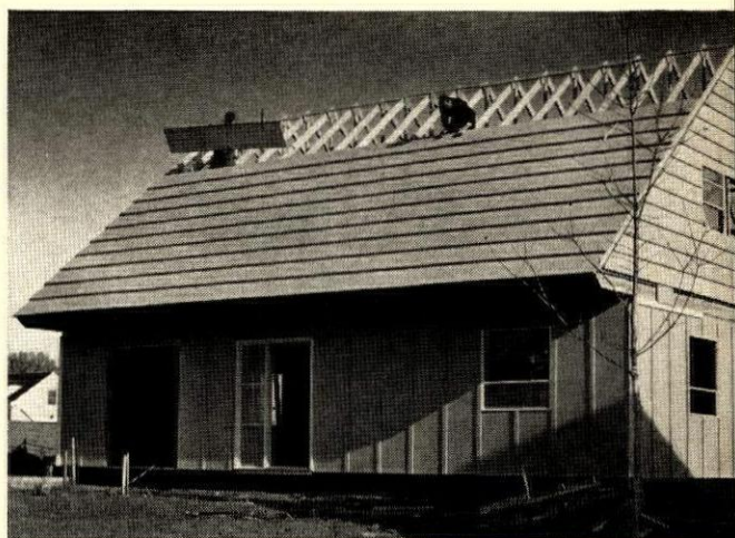
High-speed roof system uses 2 x 10-ft. Bermuda shingles made of Hypalon-surfaced plywood. It took four men six hours to install, starting at eaves with concealed nailing and folding up successive courses of the shingles. Hypalon film acts as a continuous hinge at interlocking horizontal joints.
