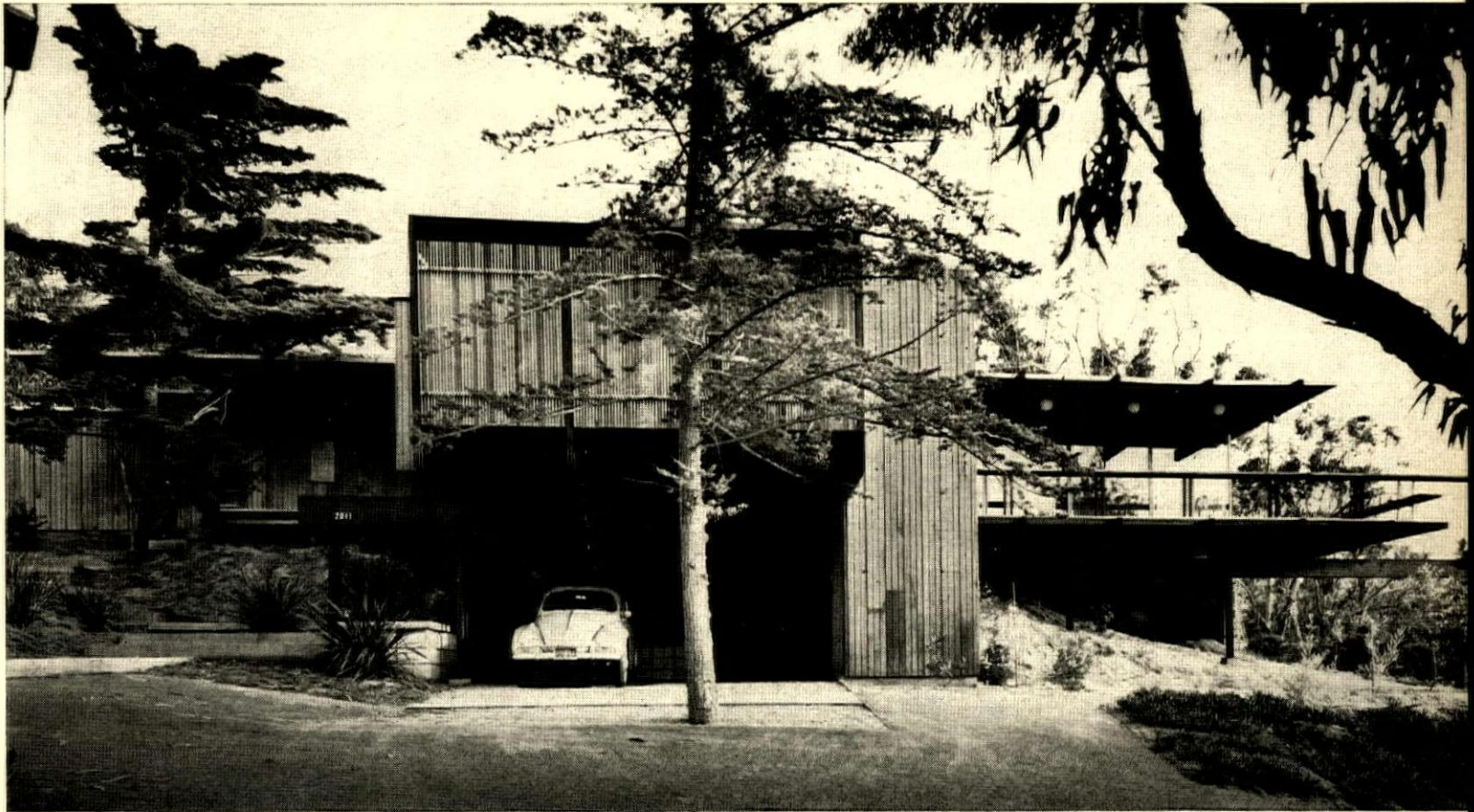
Two-story look results from projection of master bedroom suite (above carport) and living room wing (right) over the downhill slope. A future studio, with a private entrance, is planned for the space beneath the living area.
