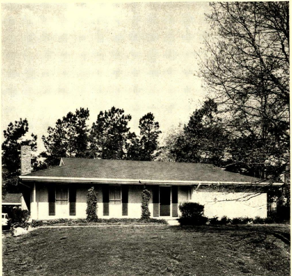
CLEAN FACADE opens only the living room to the street, while bedroom wing at right opens only to the side yard. Strong eave line helps make the house look longer.
