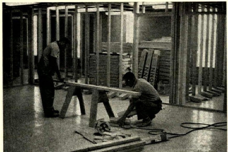
PARTITIONS are conventional wood framing. They were custom-installed to tenants' specifications after building was otherwise complete.
