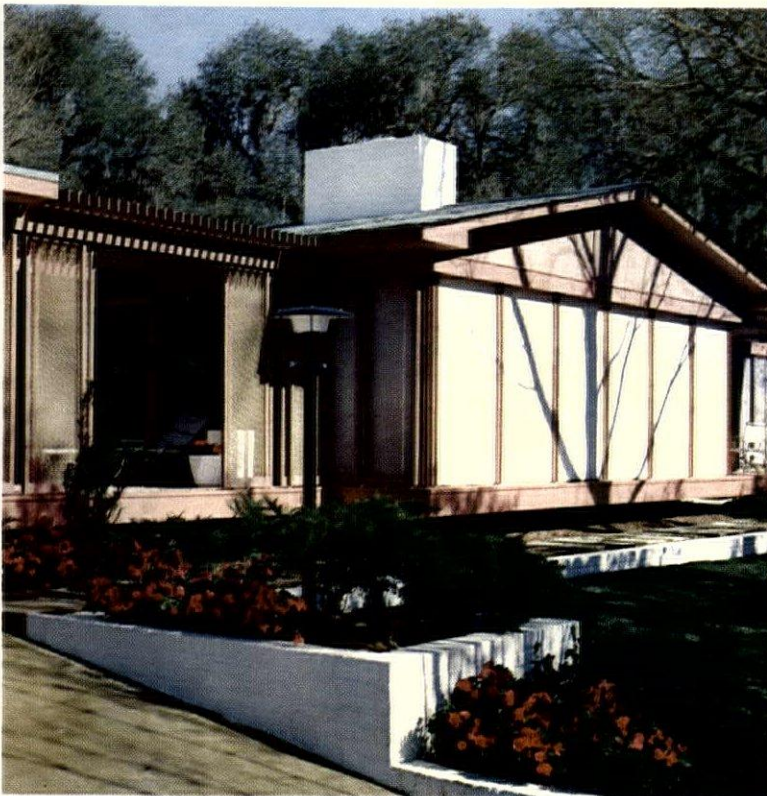
Location: Baton Rouge, La., Architect: John Brenneman, A.I.A., Home-Building Editor, LADIES' HOME JOURNAL. Builder: Crawford Corp., Baton Rouge, La. Building panels by United States Plywood Corp. are surfaced with TEDLAR.
