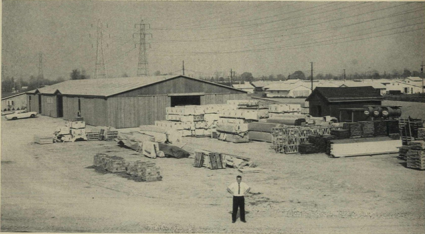
BUILDER ROBERT SCHMITT stands in front of his on-site factory-warehouse. Weatherproof materials are in yard. Shed, right, is for plumbing fabrication.
