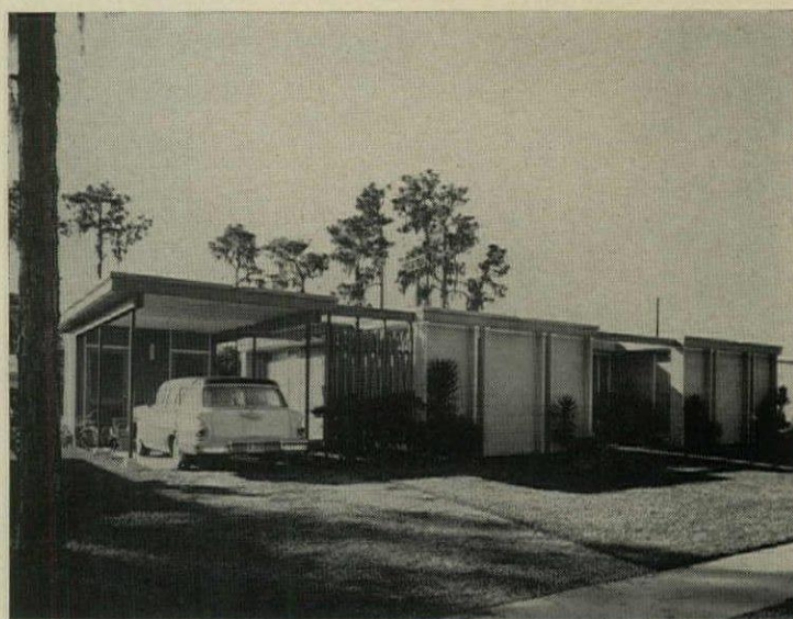
CONTEMPORARY HOUSE , designed by Architect Dean Rowe, has concrete block in stacked bond, little glass facing the street. About 10% of Carrollwood's homes are contemporary; the rest lean heavily to traditional.
