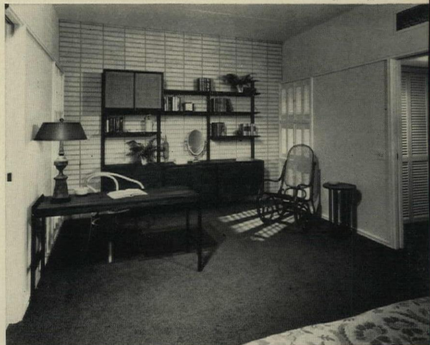
SEATING AREA of master bedroom was furnished by Designer Dean. Low ceiling of closet area and entry to room, right , was created by inverted channel beams which house the air conditioning ducts (note register).
