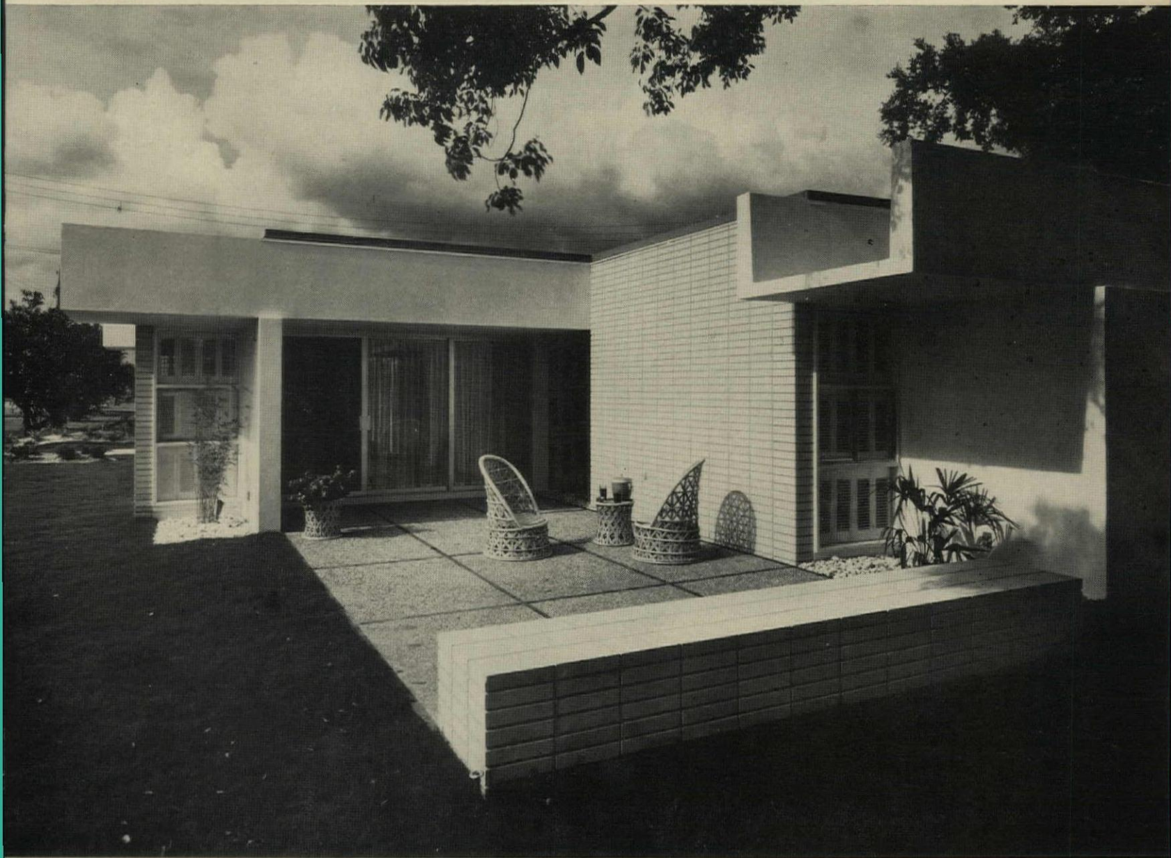
TERRACE is off the living room, which opens onto it from under a deep overhang formed by one of four inverted channel beams supporting the concrete roof slabs. Landscape Architect: Jack O. Holmes.
