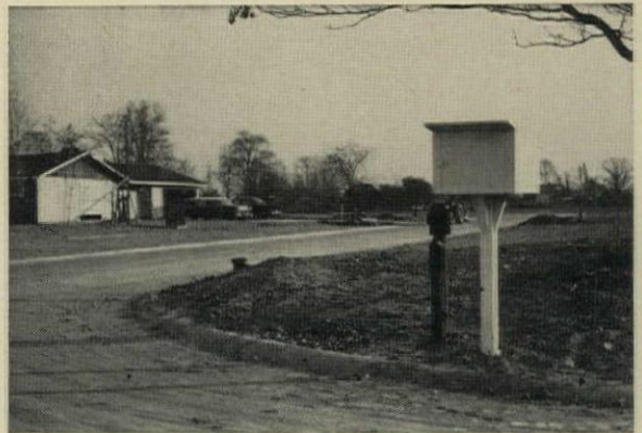
FIELD TELEPHONES are installed at strategic points around the site so field supervisors can easily contact the warehouse. Phones are connected to the site's underground circuits.
