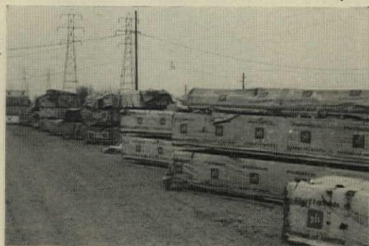
FRAMING LUMBER is stacked outdoors according to length. Diagonal piles let a forklift maneuver easily.
