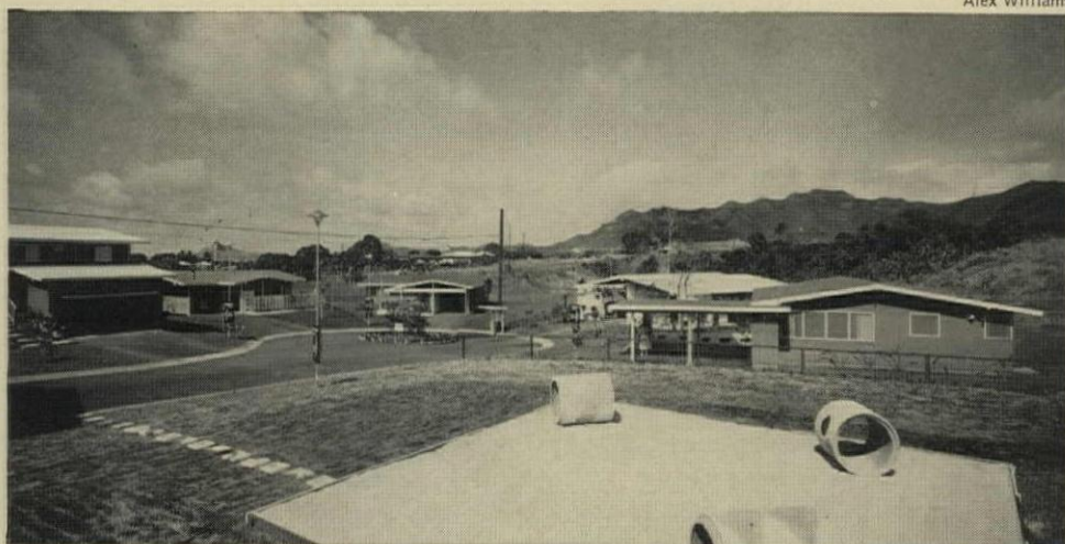
FIVE MODEL HOUSES and play area are arranged around a fenced-in cul de sac at Blackfield's current Keapuka development of 1,800 homes on the
