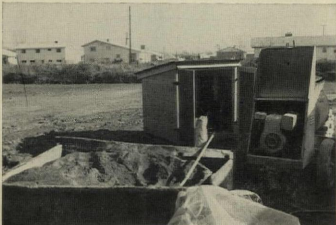
MORTAR PACKAGE includes an open box for sand, a closed box for cement bags, and a concrete mixer. Boxes are carried by a forklift truck, and the mixer is towed behind the truck.
