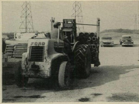
HEATING TILES piled on a fenced pallet are taken from the outdoor storage area. Tiles are delivered to Schmitt on pallets to cut out intermediate handling.
