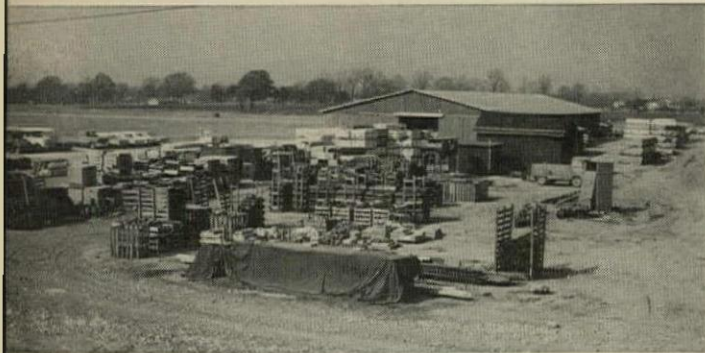
RAINPROOF MATERIAL (tile, fixtures, etc.) are stored on pallets in yard.
