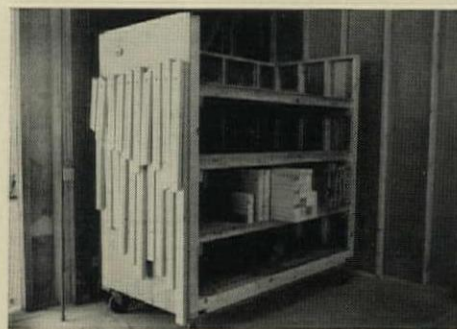
TRUSS WEB MEMBERS are stored in dolly. Hanging pieces are patterns for standard sizes.
