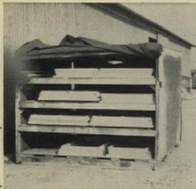
WINDOWS AND DOORS are put in phase boxes for forklifting to site. Canvas cover protects them during trip.
