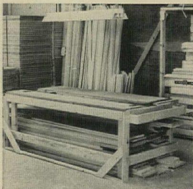
DOOR HANGING JIG was built by Schmitt's men. A finished prehung door can be turned out in seven minutes.
