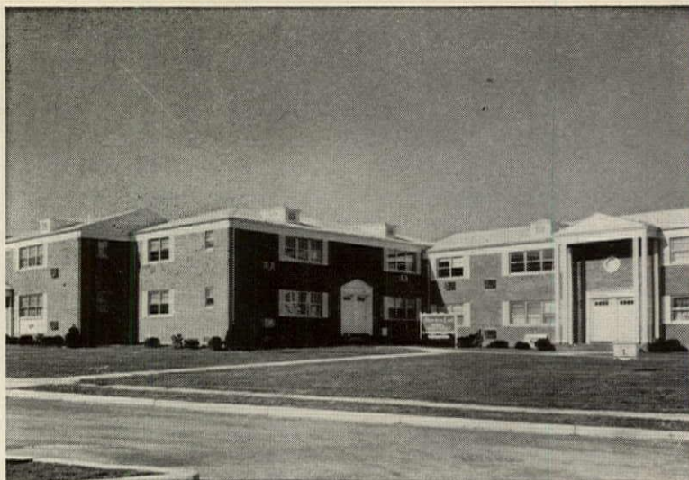
Aberdeen East, Matawan, New Jersey , is an attractive community of 240 Gold Medallion Garden Apartments being built by Arthur Goldberg and Paul Waters of Parr Associates, Inc. The sales appeal of these total-electric apartments is enhanced by the modern General Electric lighting and underground power system.
