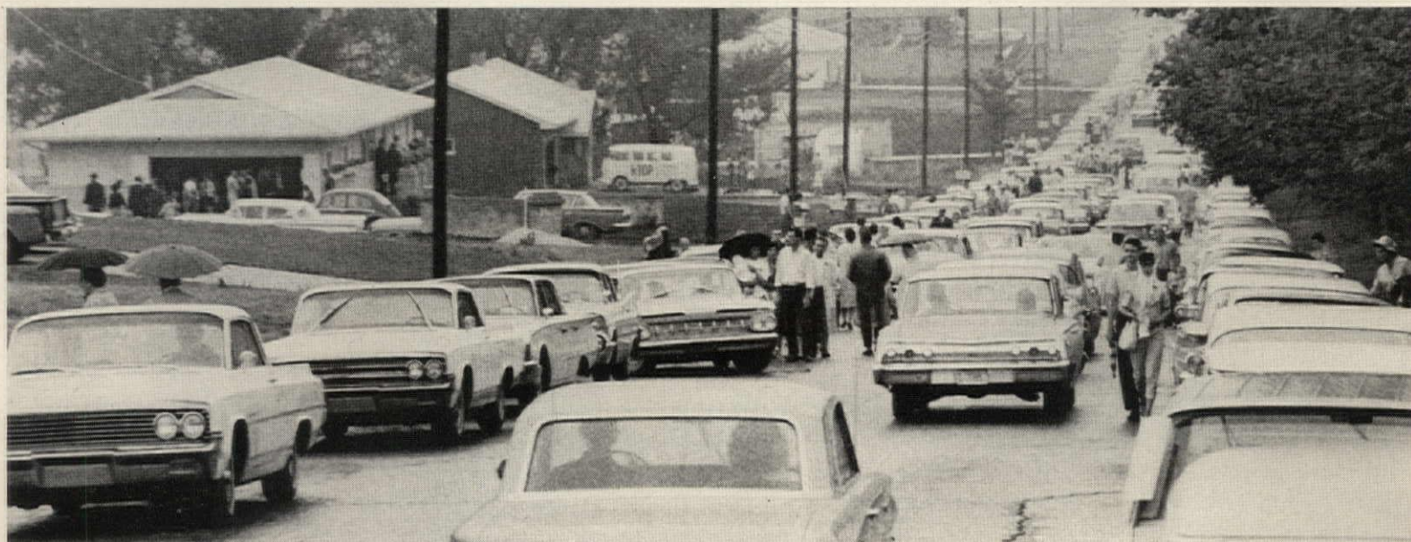
Lakeshore Estates, Topeka, Kansas , where 20,000 people turned out on opening day in the rain to tour George Emery's new Gold Medallion home community. Three hundred all-electric homes will feature a General Electric range, dishwasher, Disposall®, refrigerator, separate freezer, built-in stereo, intercom, hot water heater, central air conditioning and General Electric's ceiling cable heat.
