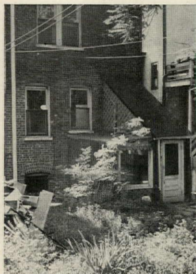
REAR TERRACE of heavily reworked private home is built on 8' footings joined to rear wall and filled with sand as base for slab. New lintels over enlarged doors and windows are 8" WF steel.
