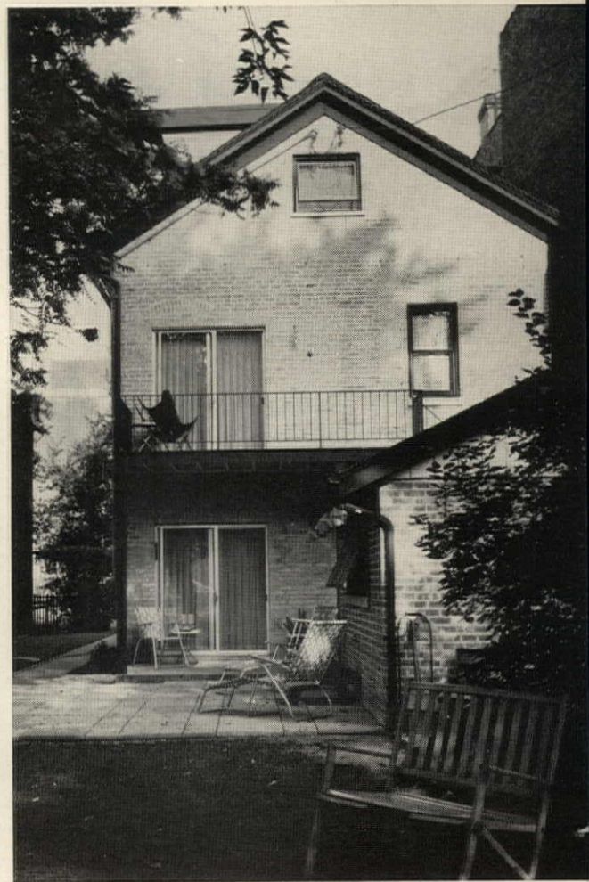
BACKYARD WING , built of used brick salvaged from neighborhood demolition jobs, houses laundry and workroom. Attic was converted to living space by raising rafters to create dormers.
