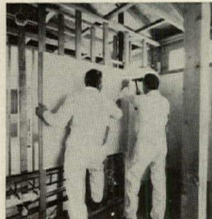
3. Gypsum board covers flanges.
