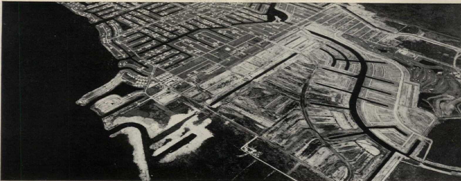
Cape Coral, Florida , where Gulf American Land Corporation is building Medallion Homes on carefully planned waterfront lots. Each contemporary Florida home will feature a modern General Electric kitchen and electric climate control for year-round comfort. All-electric living, coupled with well-planned community facilities, are making Cape Coral one of Florida's most successful residential communities.
