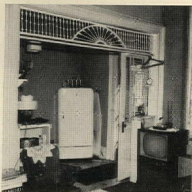
KITCHEN WALL turns annex into full kitchen and creates formal dining room ( plan opposite ). Baseboard for new partition comes from salvage. Old grille and casing are saved for restoration jobs.
