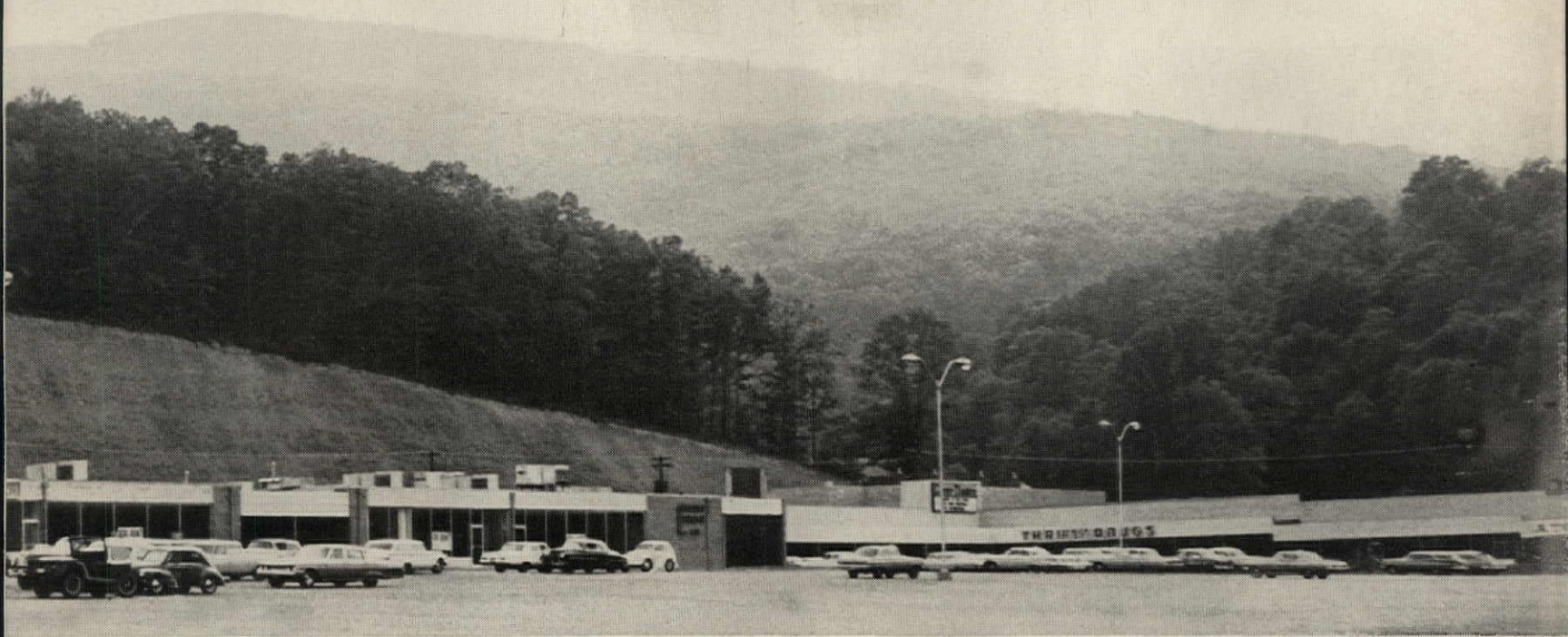
Searstown, Cumberland, Maryland. C. Yoder & Sons, Heating and Cooling Contractor.
