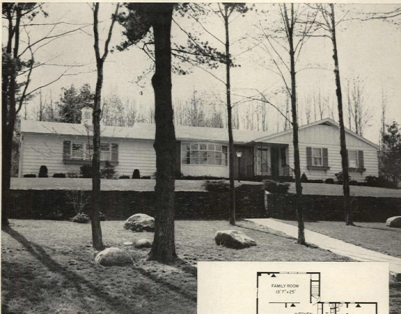
Builder: Crowley Realty Corp. Feature: Concealed Telephone Wiring
