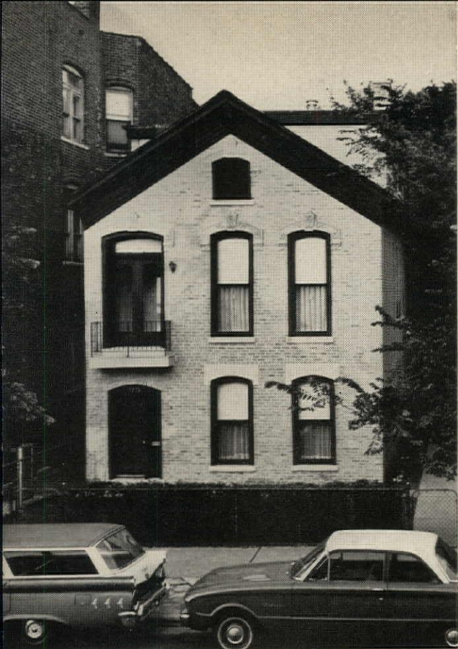
LOWERED ENTRANCE and second-level balcony simplify this "Chicago cottage" facade. To remove old front steps, remodelers had to build new inside stairway for second-floor access.
