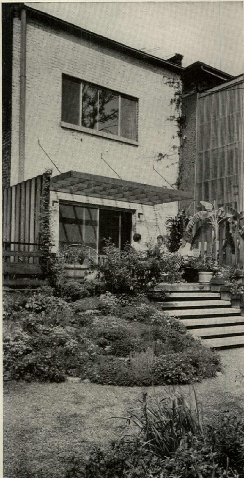
REAR TERRACE of heavily reworked private home is built on 8' footings joined to rear wall and filled with sand as base for slab. New lintels over enlarged doors and windows are 8" WF steel.
