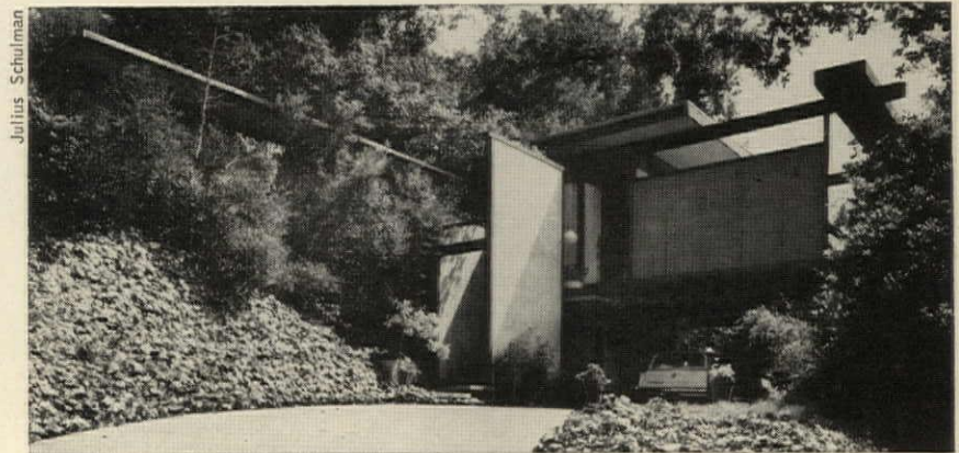
From street, length of house on upper level is hidden behind shrubbery. Deck above carport opens off high-ceilinged living room, but is screened on the street side by a lattice wall.
