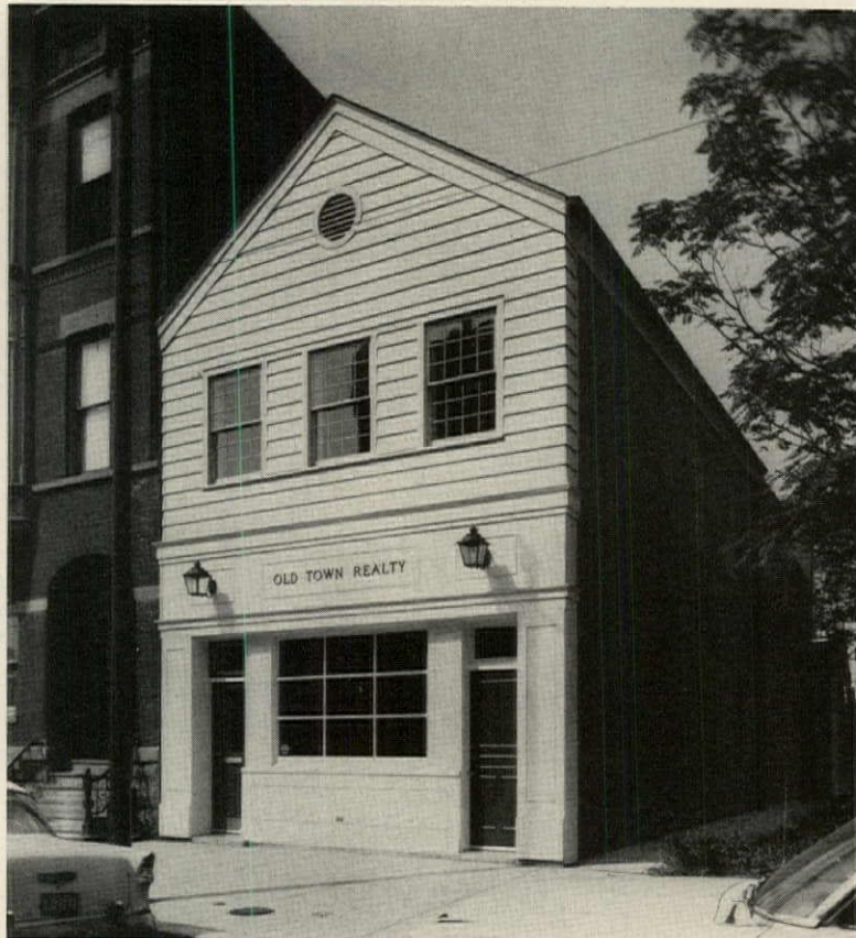
REMODELER'S OFFICE , formerly one of the neighborhood's shabbiest structures, was a bargain for Halligan. He removed false front to reveal roof peak and applied new colonial facade.
