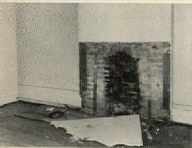
FIREPLACE WALL was already there. Remodeler exposed existing brick wall by pulling off plaster surrounding old fireplace, then constructed new hearth and mantle with matching used brick.
