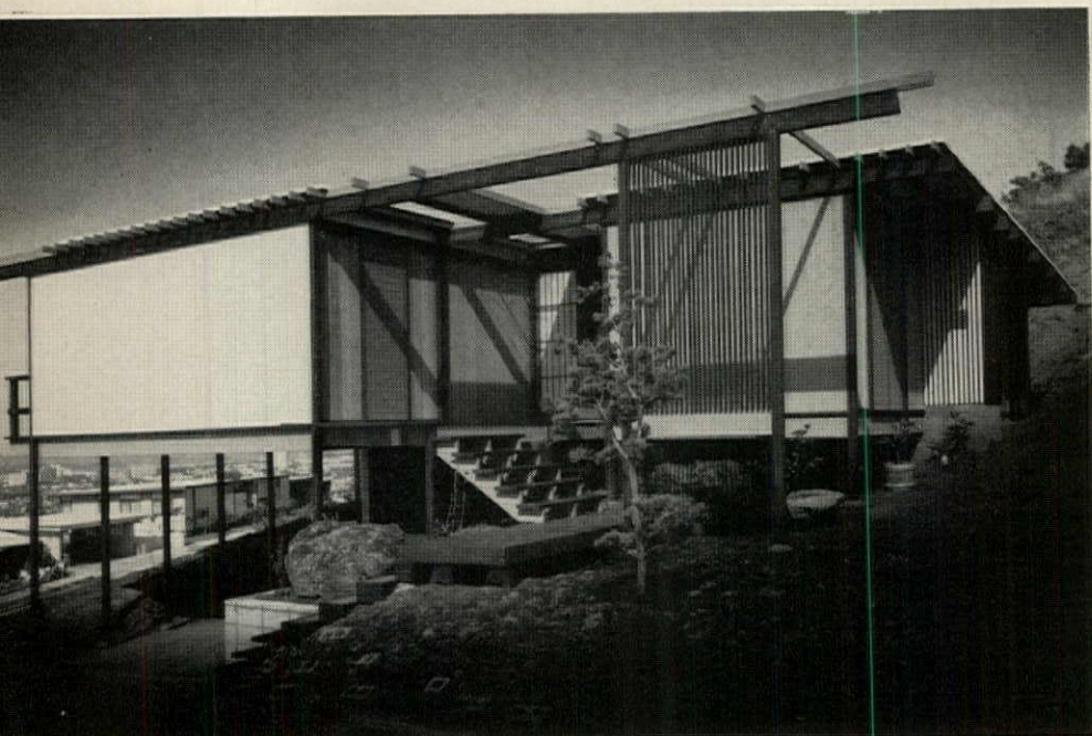
Steep site dictated post underpinning, and in Japanese fashion posts are set on natural rounded-rock footings. Roof framing is 2 x 4 joists on edge ( section, opposite ).
