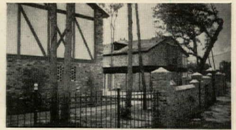
BRICK WALL on one side and bayous on two sides keep the five-acre triangular track private.
