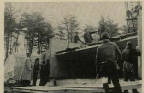
3. Hinged floor section is lowered by crane. Roof panels, foreground, are bolted on later.
