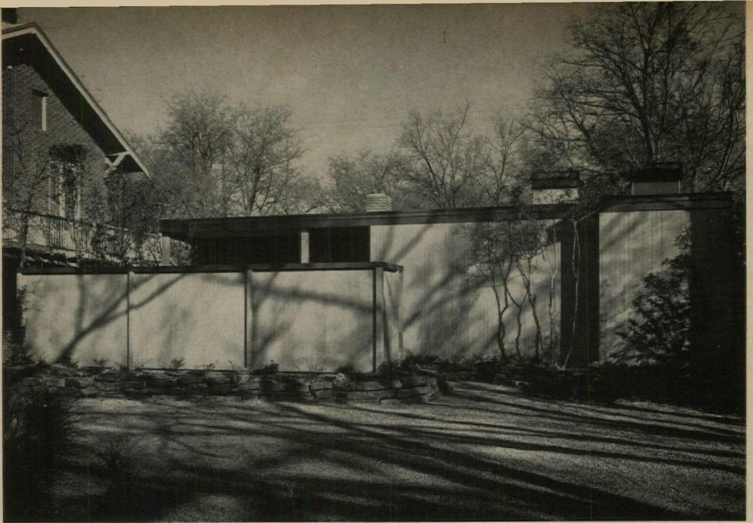
STREETFRONT PRIVACY on narrow lot was achieved by screening entry and living room window with 6' fence made of exterior siding boards.
