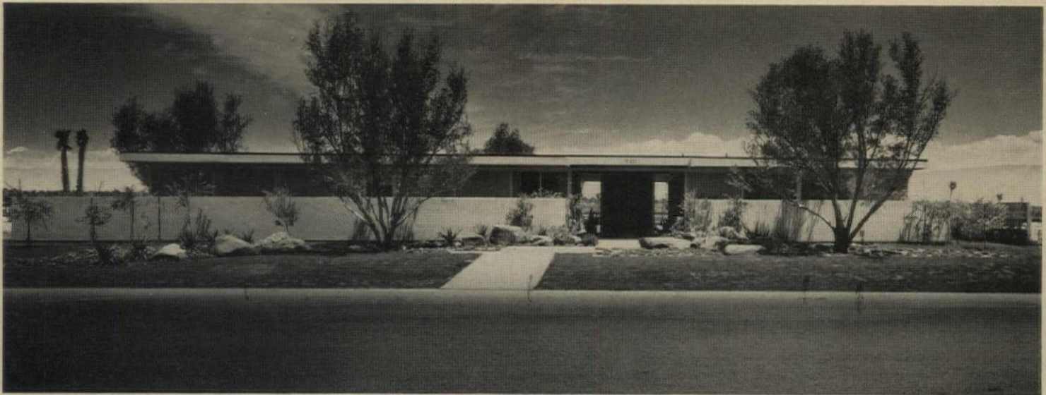
LONG FRONT WALL conceals all rooms but leaves see-through entry exposed. Post-and-beam exterior is finished with stucco and stained redwood.
