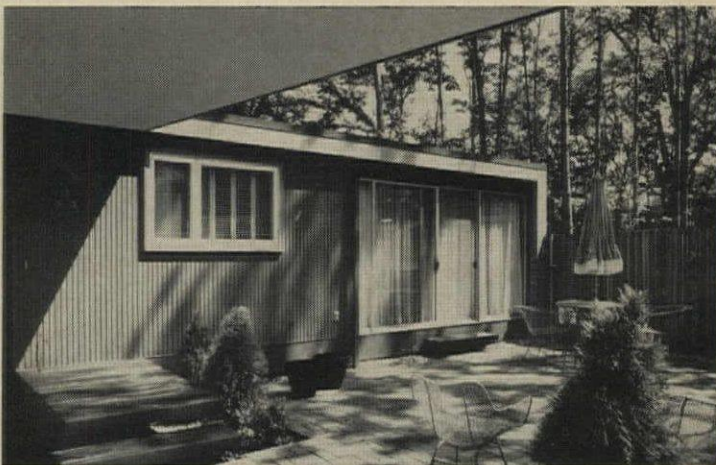
FRONT PATIO , off dining room, is screened on two sides by redwood fence and carport. Deep overhang of carport, foreground, covers approach to entry.
