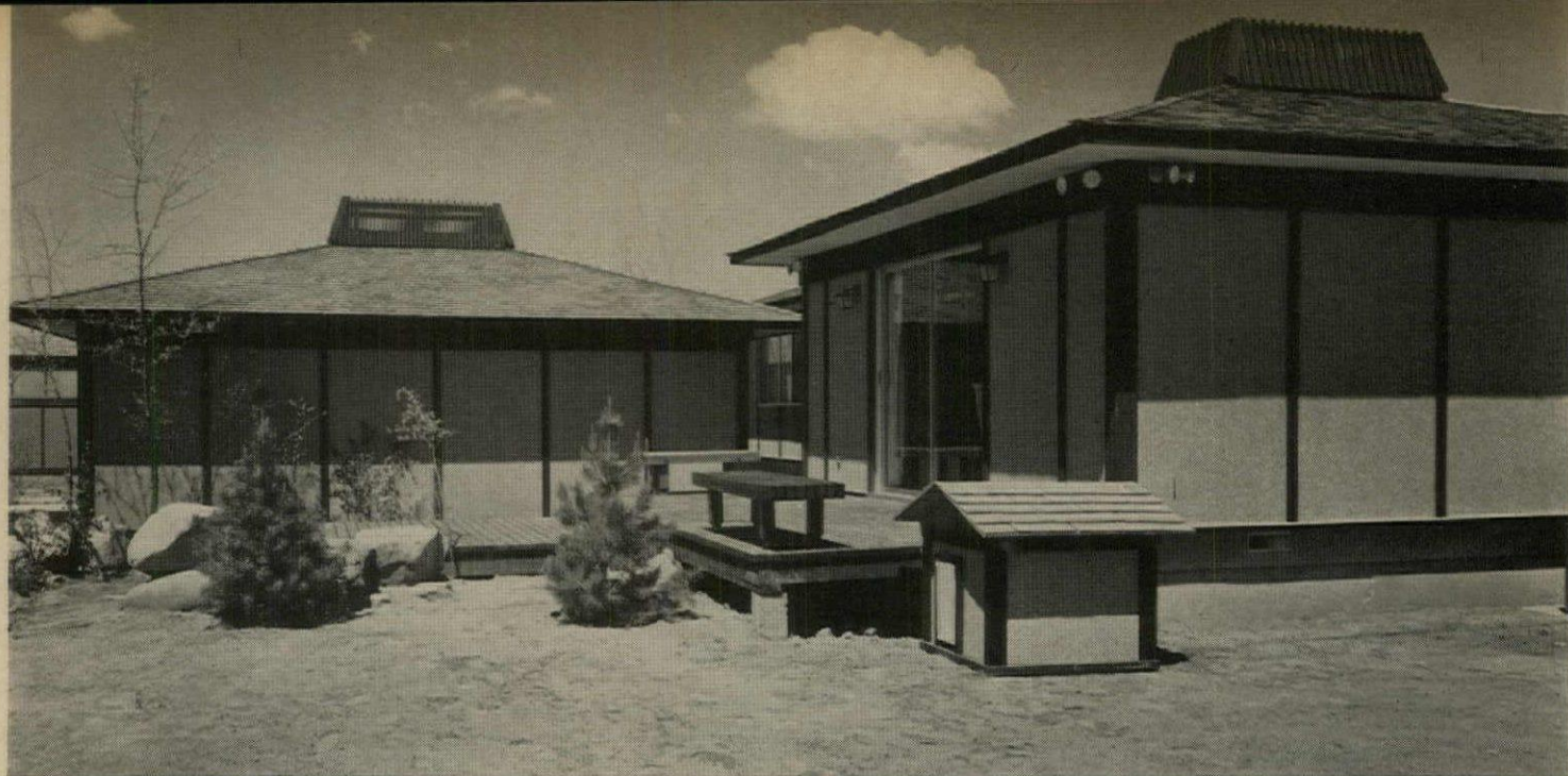
MODULAR PAVILIONS offer wide choice of siting plans and elevations. Buyer has option to expand any floor plan by 4'. Doghouse is optional.
