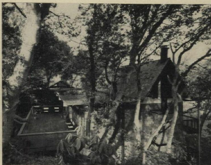
HIGH-PEAKED ROOF permits big glass gable ends above living room. Cantilevered fireplace at upper level is cedar-shingled as part of wall.
