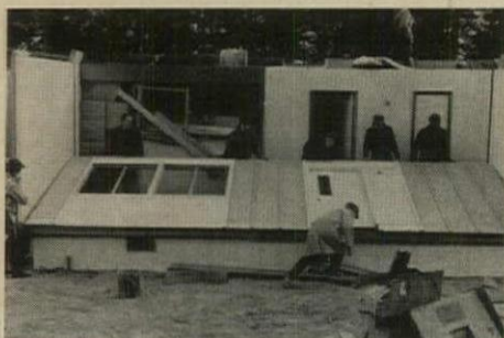
4. Front wall, hinged to floor, is tilted up. Foam sealer strip is placed between hinge leaves.
