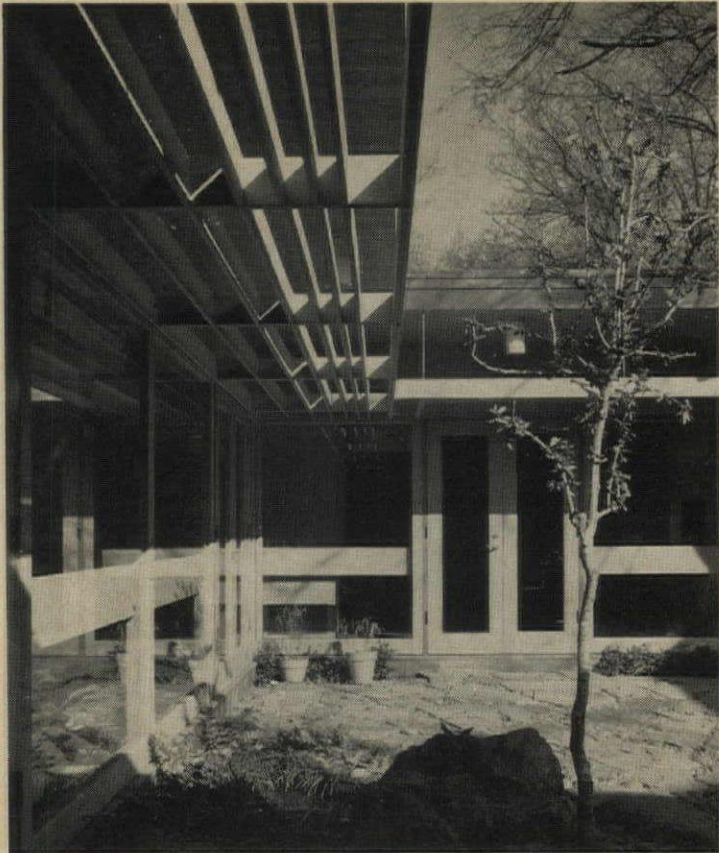
OFF-CENTER COURT is enclosed on three sides by C-shaped house. Grid under high overhang is sun baffle for south-facing window walls.
