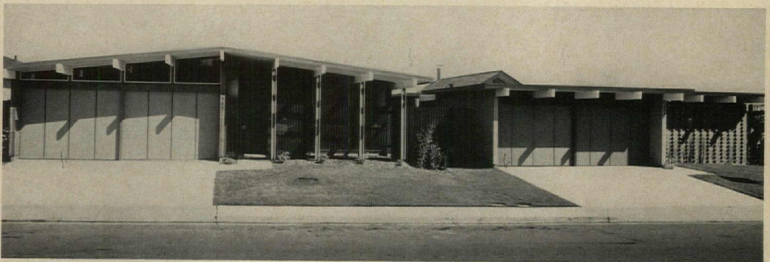
VARIED ELEVATIONS for same plan—sloping roof above entire house, left, or flat roof with open gables—avoid row-house look on narrow lots.
