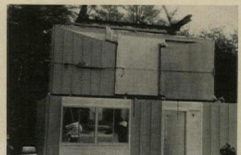
6. Upper-level section is set at center of lower section. Partitions are shipped loose inside.
