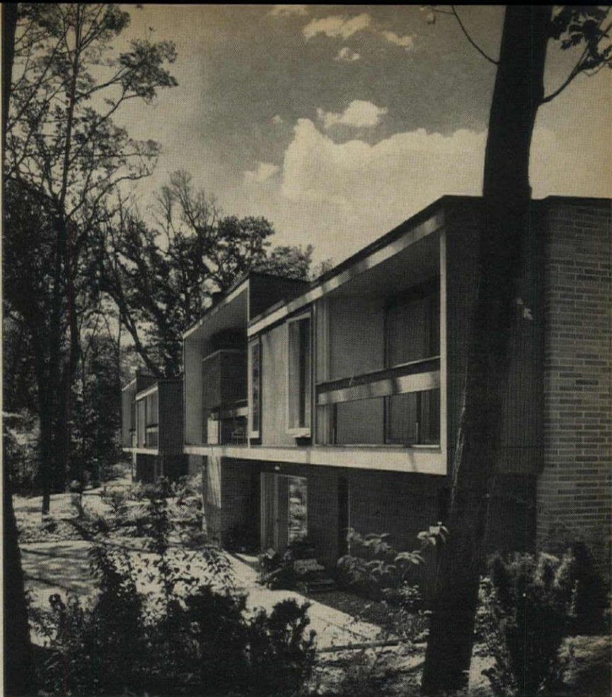
REAR BALCONIES are enclosed by redwood sidewalls. Only other windows are at front. Neighboring houses cannot be seen from any position inside.
