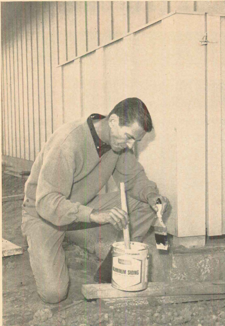
Silicone-alkyd finish , available in seven colors, is formulated especially for unpainted aluminum but can also be used on steel, iron and galvanized metal. The manufacturer says it will last nine years. Dow Corning, Greensboro, N.C. Circle 206 on Reader Service card
