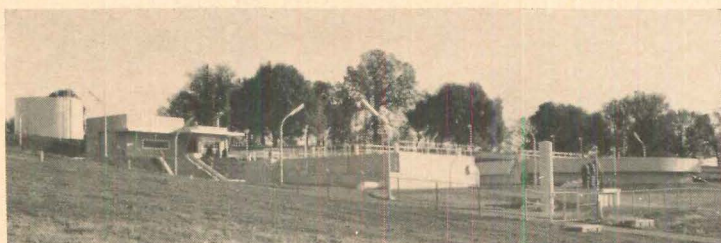
WATER TREATMENT PLANT is at north end of project. It (and sewers) can serve 3,000 homes.
