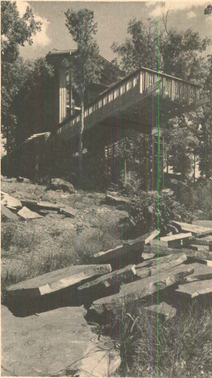
PROJECTING DECK above slope extends the living area, leaves rocky site undisturbed.
