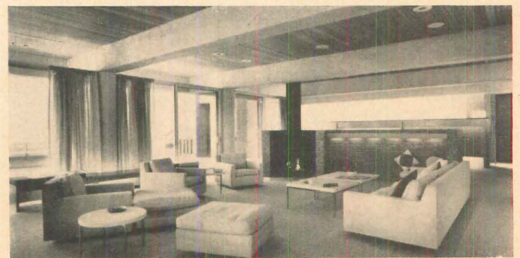
MASSIVE BEAMS of concrete span the open living area, support upper roof deck.
