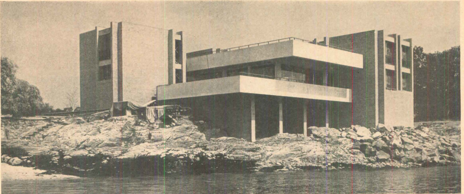
VIEW FROM WATER shows rocky site, concrete supports for center section. High concrete parapets protect both upper and lower decks.
