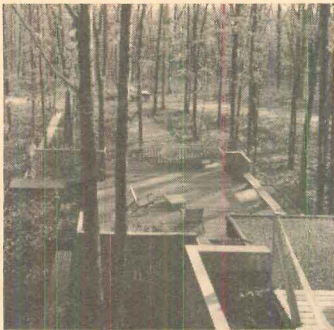
DESCENDING ROOFTOPS form series of terraces and decks.
