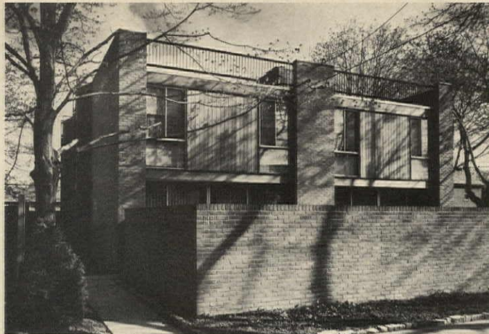
INSIDE WALK leads past patio gate to two house entrances beyond. Patio walls do not come under setback rules, can thus be close to street.
