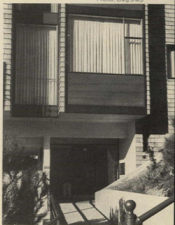
MAIN ENTRANCE is off pedestrian walkway at second parking level. Structure is built right out to lot line on this side. Bay window above entrance projects over the line, provides dining alcoves for one-bedroom units.
