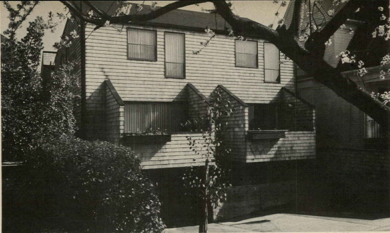
FACADE of front building is dominated by two walled balconies. Entrance to basement parking is at left, outdoor parking court is at right.
