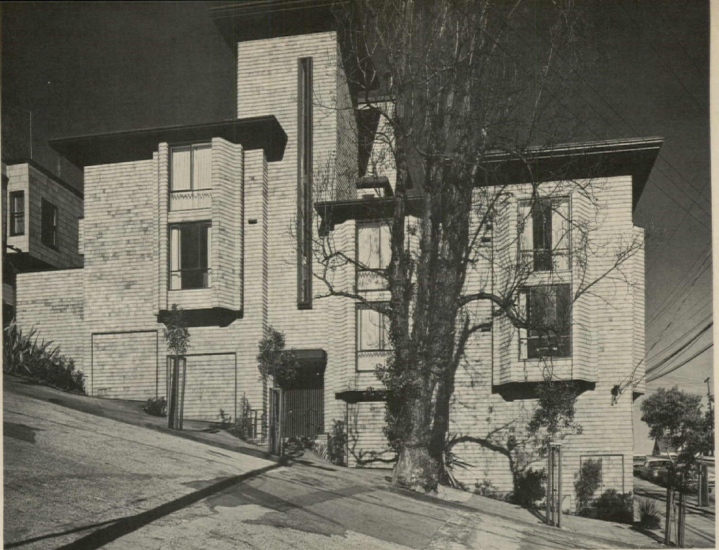
FRONT ELEVATION (see cover) includes main entry, flanked by three camouflaged garage doors. Tower above entry holds main staircase.
