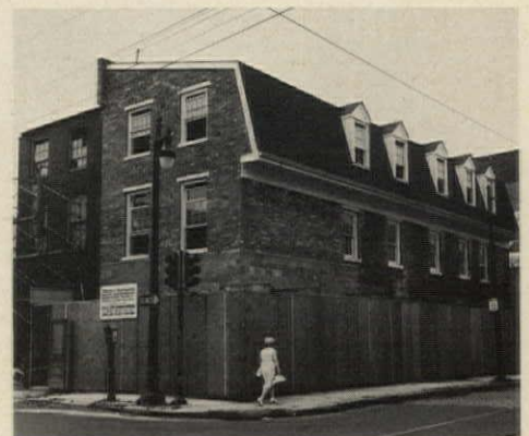
HIGH-PRICE REHAB is being overlooked as a testing ground for systems manufacturers.
