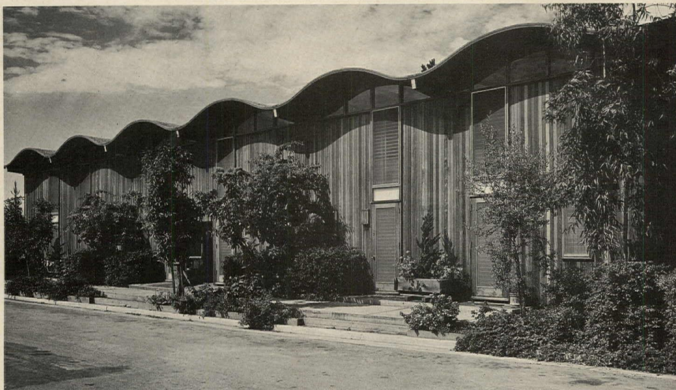
STREET ELEVATION has blank walls, louvered doors and windows to maintain privacy. Clerestories under roof vaults admit extra light.
