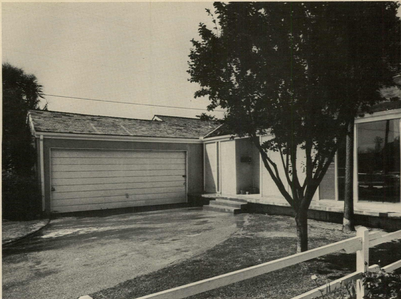
REMODELED HOUSE is an expanded version of a standard California ranch model. Before and after plans on facing page show how living
