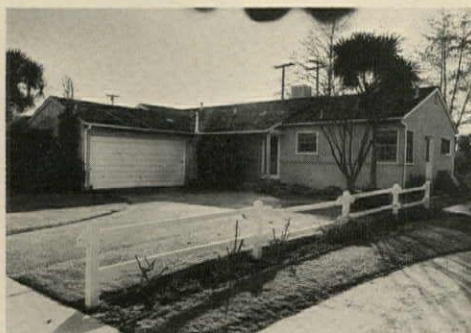
ORIGINAL HOUSE was typical tract model, well located, but too small for owner.
