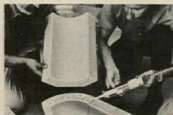
Prefabricated hydro-pool is delivered to installation site ready for assembly. Parts (top) include fiberglass modules, filter, pump and air inlets. Sealant is applied (above left) prior to bolting and final caulking. Jacuzzi, Berkeley, Calif. Circle 236 on Reader Service card
