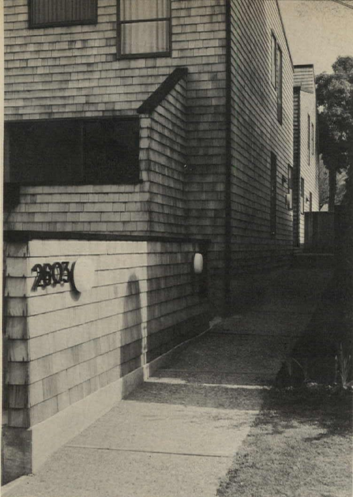
ENTRANCE WALK runs along right edge of lot to area between buildings (plan). Low wall at left separates walk from front parking area.
