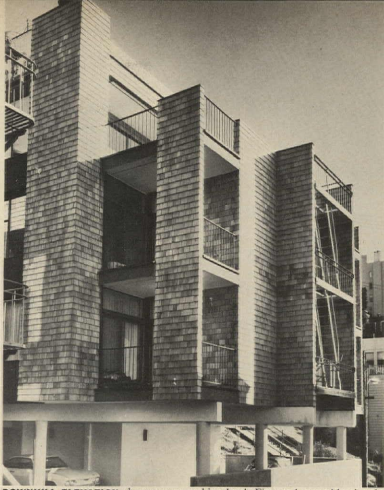
DOWNHILL ELEVATION shows upper parking level. First and second-level units have covered balconies, penthouse has open deck. Fire escape is at right.
