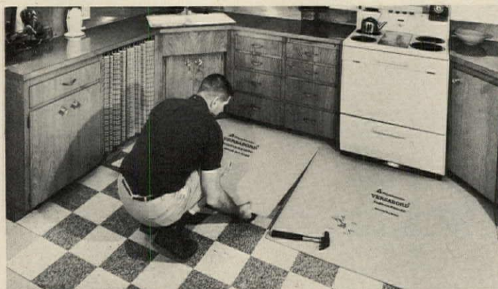
Particleboard underlayment , designed especially for floor remodeling, resists warping and denting because it has no grain. It comes in 4'x8' panels, 1/4" thick, and cuts with ordinary tools without flaking. Weyerhaeuser, Tacoma. Circle 222 on Reader Service card
