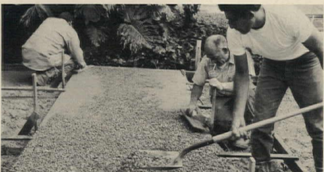
3. Colorful aggregate of uniform size ( \frac{1}{4} - to \frac{1}{2} -inch on this job) is seeded from shovel. In background two finishers have already begun tamping in aggregate with wooden hand floats.
