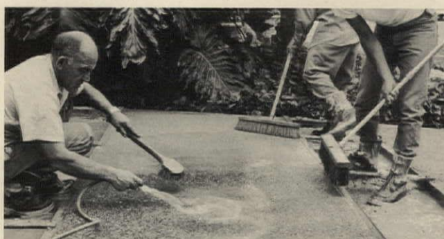
6. Medium-bristle push brooms are used for major brushing. The man with the hose touches up areas missed by the large brooms. This is the final step in producing the exposed aggregate finish.
