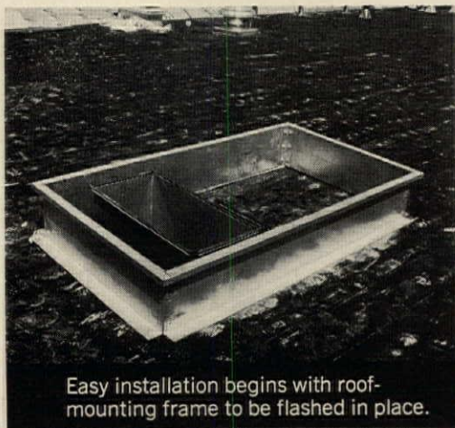
All ducts pierce roof within the frame.
