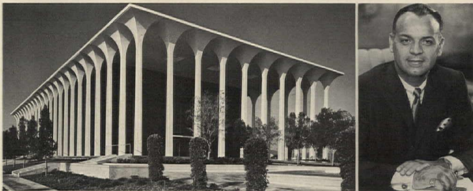
LAVISH HEADQUARTERS (left) reflects outsized empire created by Ross Cortese (right). Three-story structure has 70,000 sq. ft., 64 columns and glass walls. Cost: $2.5 million.
