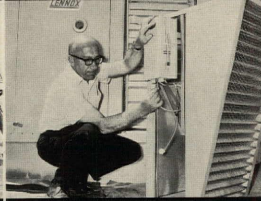
Simple "plug-in" connections for fresh air intake.
