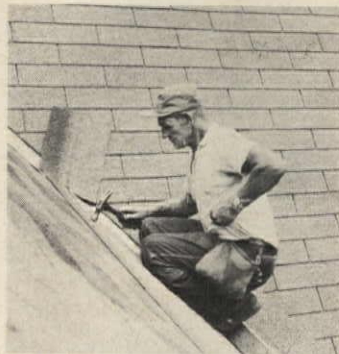
Self-sealing shingles —said to be storm-tight in hurricanes—feature extra-large granules on asphalt. The granules are fungus-resistant to preserve colors longer. Shingle strips have two 18" tabs. Johns-Manville, New York City. Circle 238 on Reader Service card
