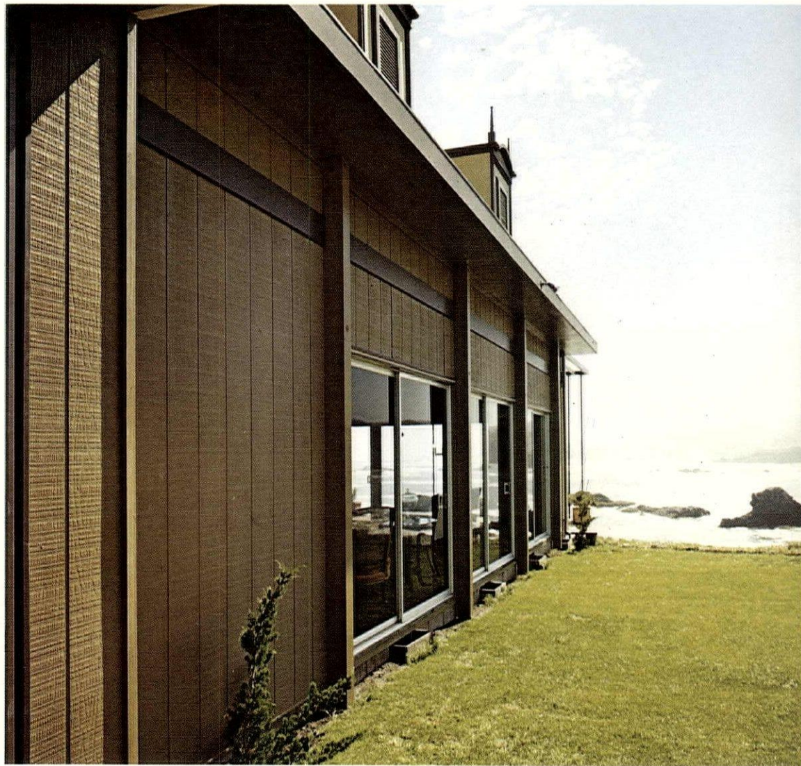
RUF-X-90 Panelgroove siding. \frac{3}{8} " square cut grooves on 4" or 8" centers, 4' wide up to 10' long—with rough-sawn deep textured finish.
