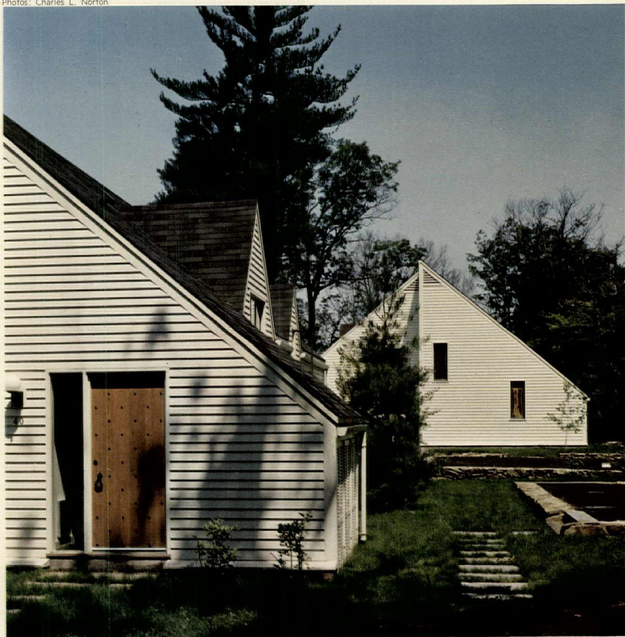
FARMHOUSE FEELING of apartments is maintained by white clapboards, steep gable roofs and set-in dormer windows.
