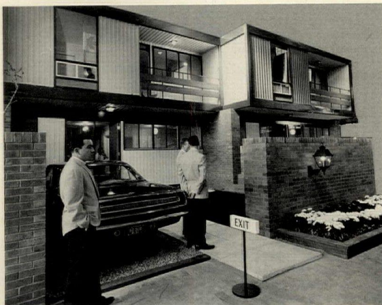
STEEL BOXES stacked on masonry walls to make 1,500-sq.-ft. townhouses were shown at a Toronto home show last year. But the system has yet to appear in the market.
