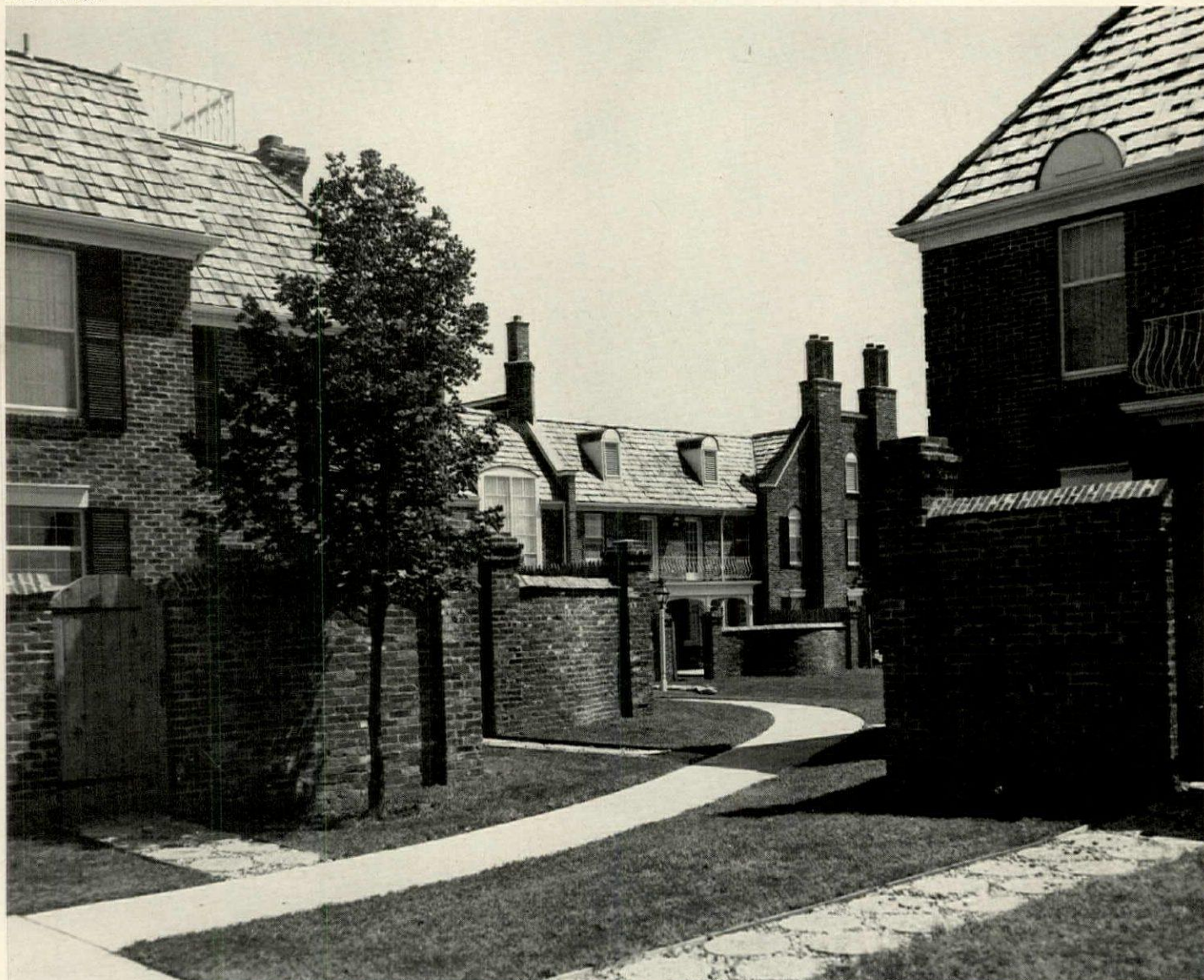
LANDSCAPED WALKS lead from parking areas, foreground, to private entrances. Patios are hidden behind the low brick walls.
