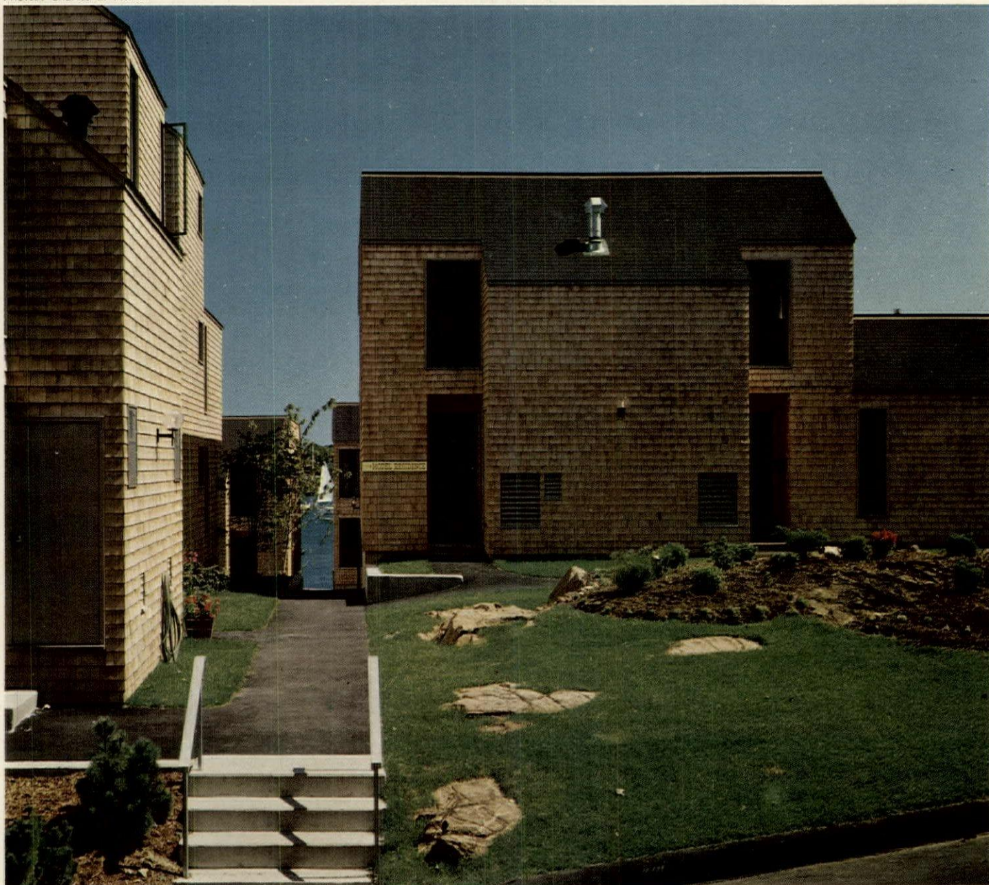
TRADITION is represented by shingles that will turn silver gray in the salt air. Slot windows were controversial items, but are now well liked.
