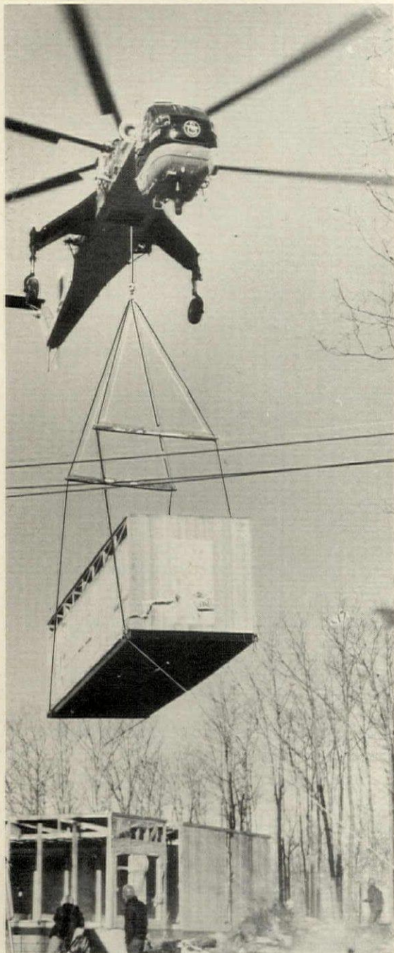
TEN-TON HELICOPTER , already used for jobs like that above, may carry 2½-high boxes into Baltimore.
