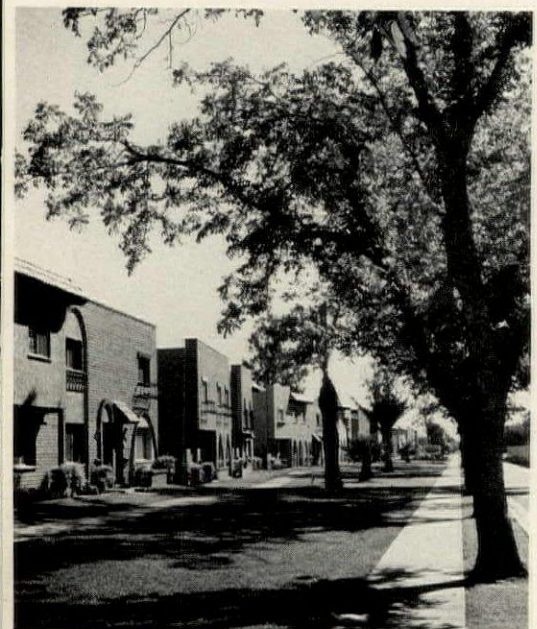
PHOENIX TOWNHOUSES reflect local flavor outside but have stock Hallcraft plans inside.
