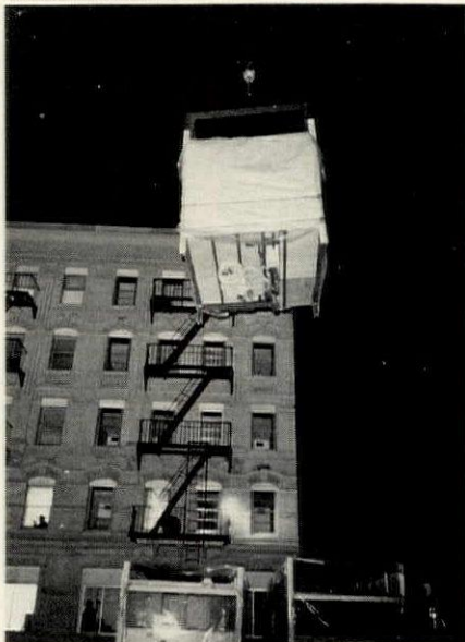
REHAB BOX is hoisted through the roof.
