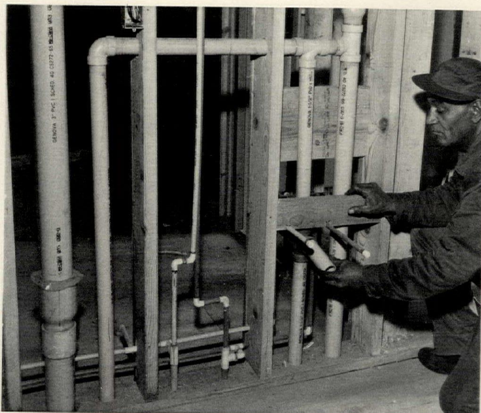
ALL-PLASTIC PLUMBING SYSTEM of B.F. Goodrich polyvinyl chloride has passed FHA requirements for rehabilitation work. Estimated cost saving compared with copper pipe: 35%.
