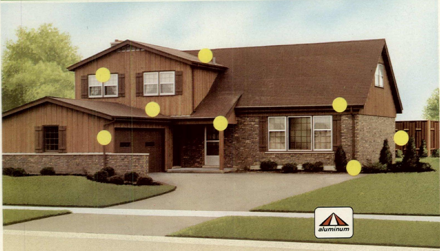
The "Concord": Pembroke Greens, Naperville, Ill.; as built by Harris Home Builders (land developers and home builders in Chicago area); Mr. William F. Harris, Pres.
