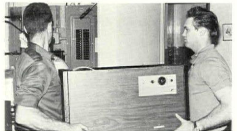
INSTALLATION of Ozonator, which weighs about 100 lbs., requires a two-man crew. The metal enclosure is 30" long, 18" high and 17" deep.
