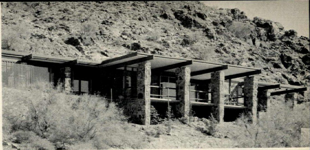
STONE PIERS support deep overhang on southern elevation, also serve as partial sun shields.
