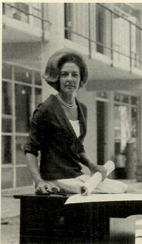
DEVELOPER CASTER At a construction site in Phoenix
