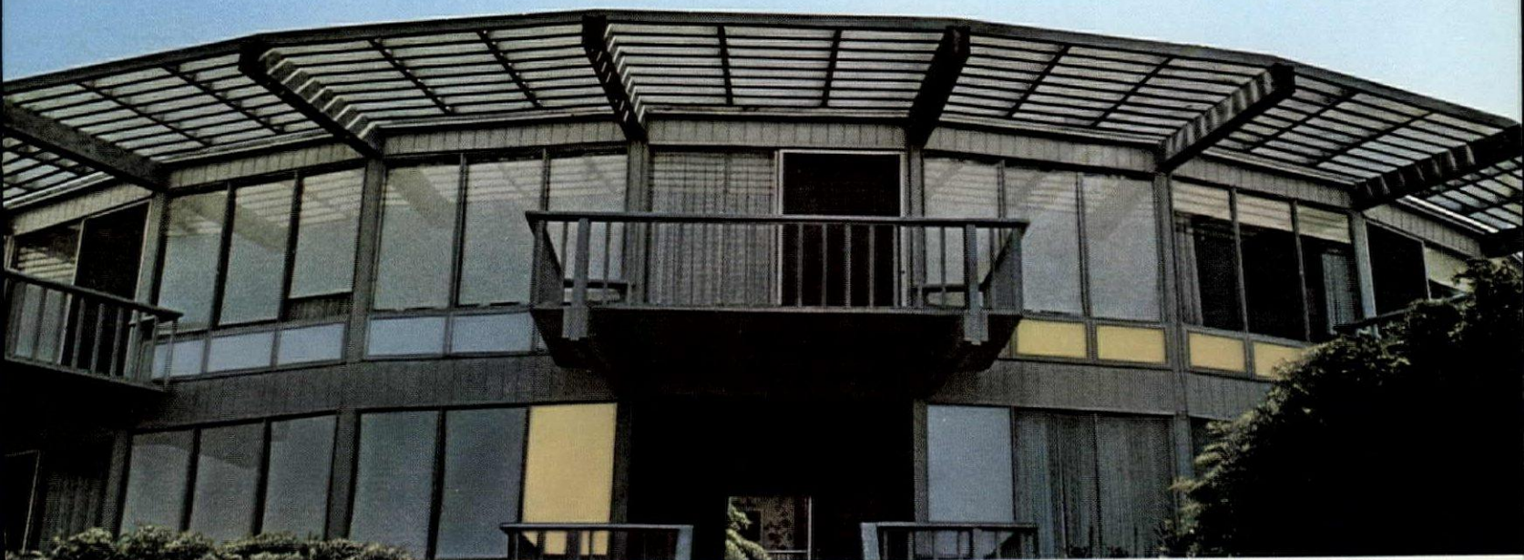
GLASWELD INSTALLED APRIL 1960, PHOTO TAKEN JUNE 1968.
