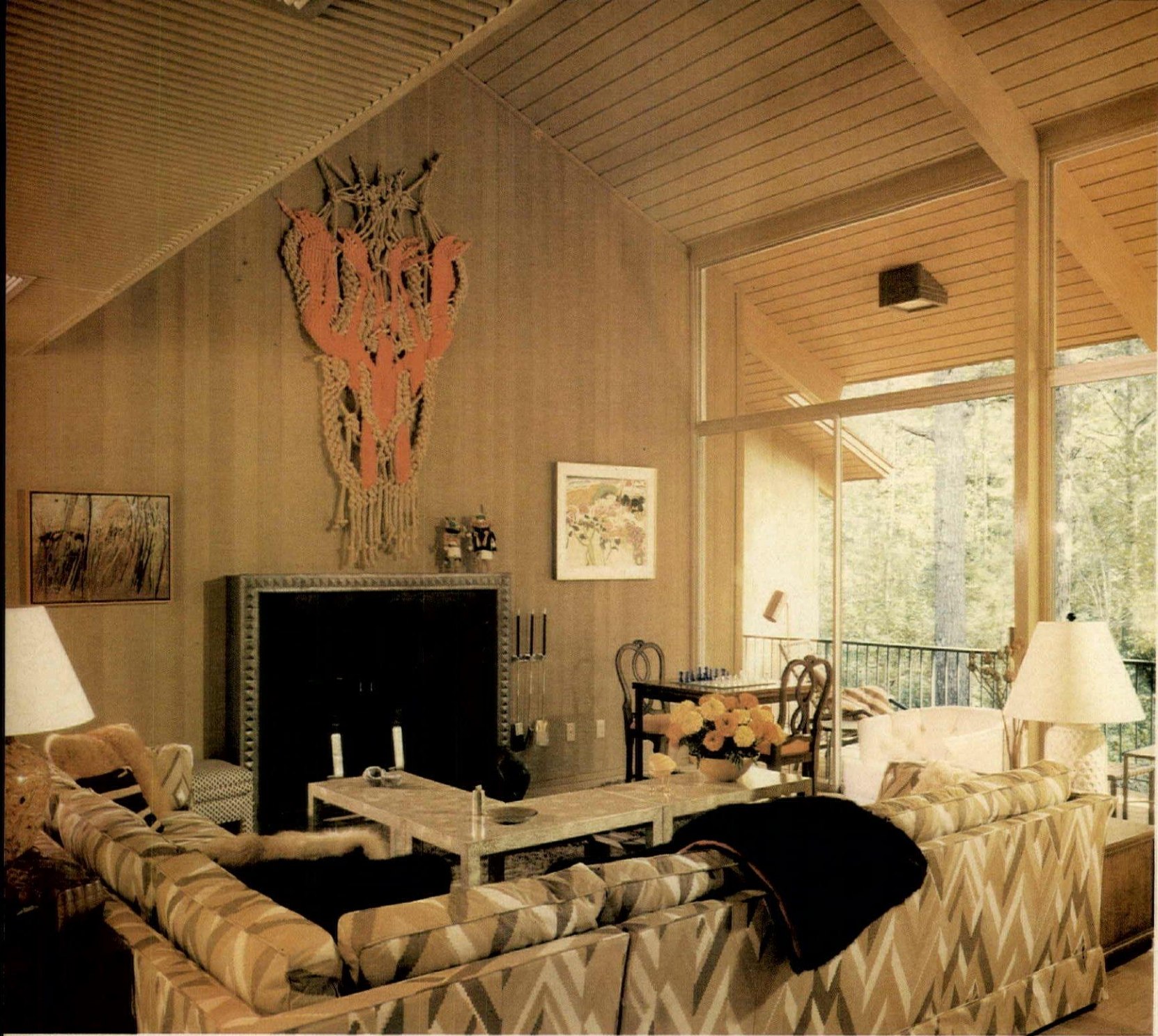
LIVING ROOM (view 1 in plan on facing page) is topped with vaulted plank-and-beam ceiling — 3x6 T&G planking over rafters 9' o.c. Rafters are in turn supported by posts which rest on under-floor girders 9' o.c. (see photo on p. 79). Dropped ceiling section with ribbed surface at upper left is the underside of the second floor.
