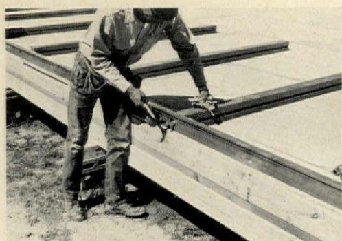
1. PREDRILLED BOTTOM PLATE is fastened to predrilled studs with lag screws. Workman sets screw with a hammer, tightens it up with a socket wrench. Plate sections are linked by shiplap joints.
