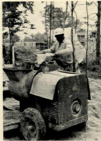
8 Built-on bag opener cuts out a work step. Mortar bags used to be opened by hand—one motion per bag—until a triangular cutter
