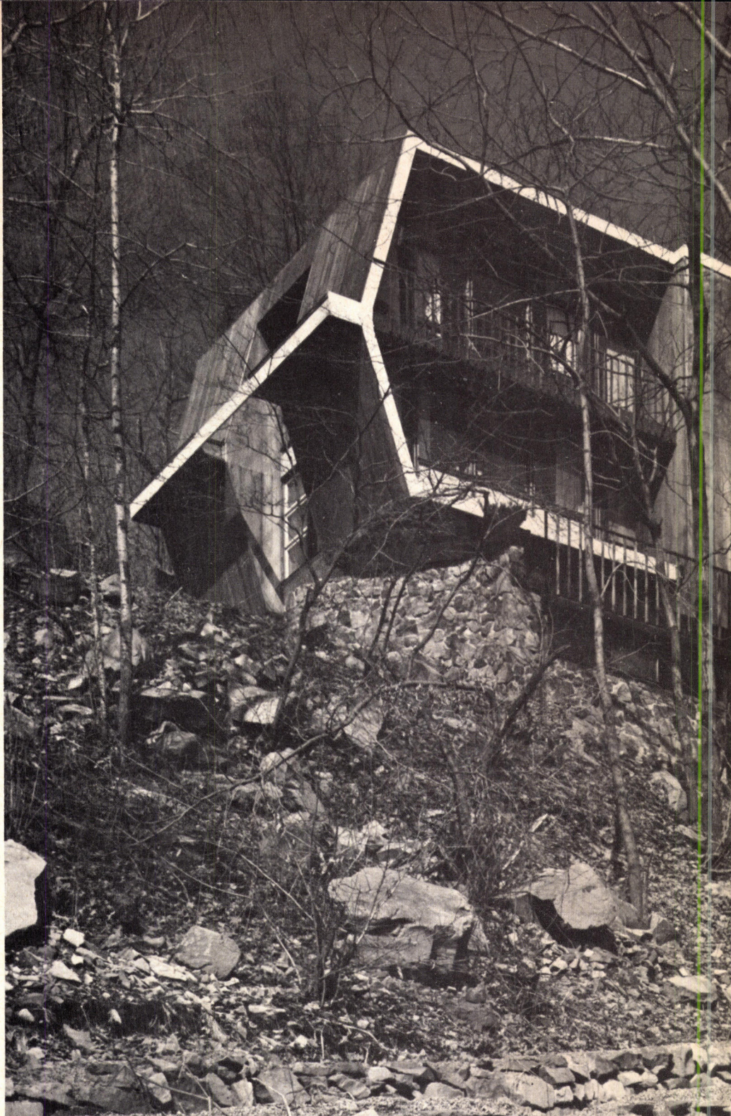
FRONT ELEVATION shows steepness of site. Garage is behind stone wall at bottom level.
