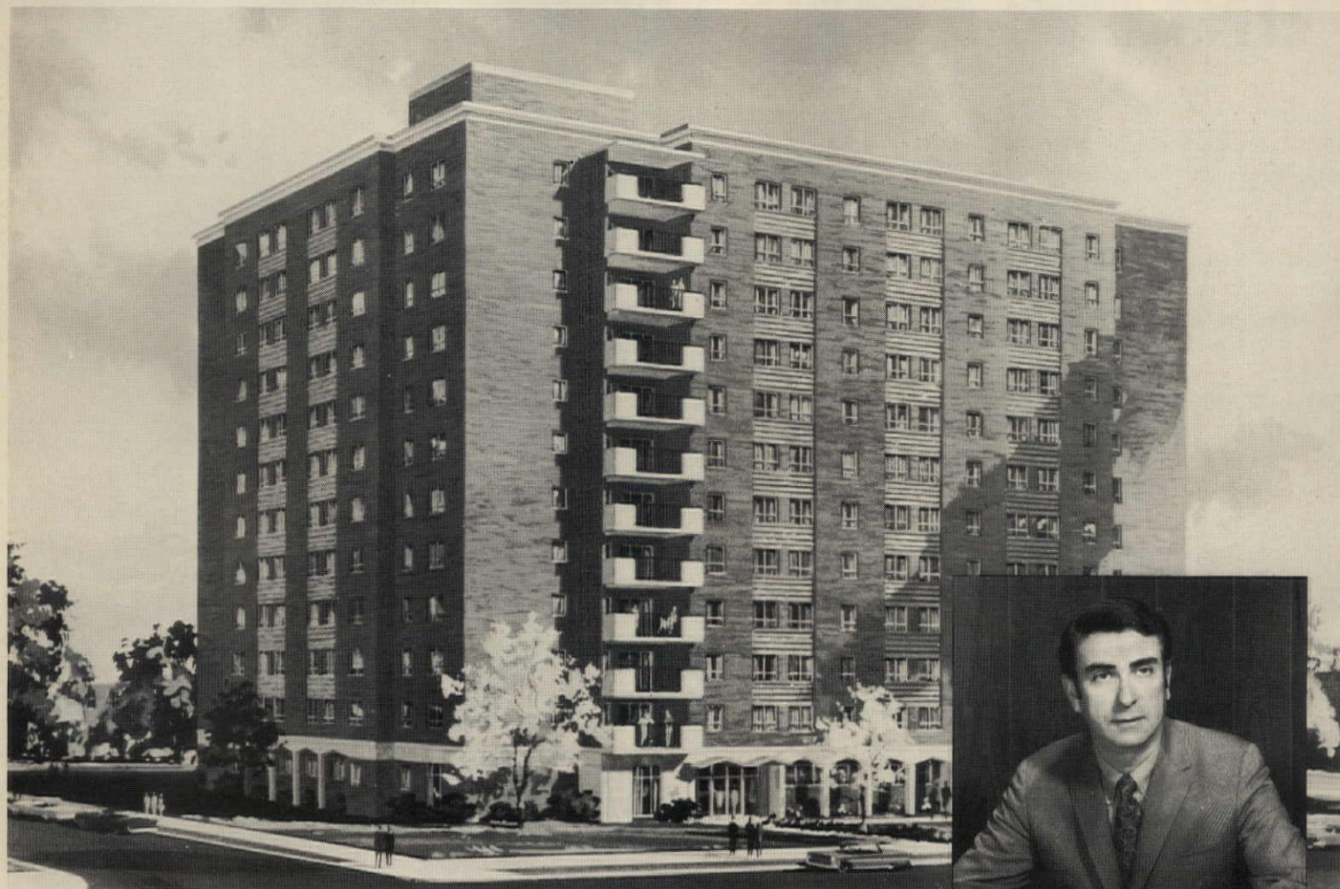
Paul E. Belcher Apartments, 400 Locust St., Akron, Ohio
