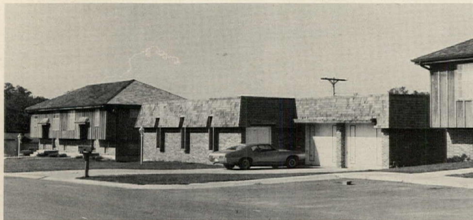
MANSARD-ROOFED SEWAGE PLANT looks like house, even has gas lamp and mail box in front.
