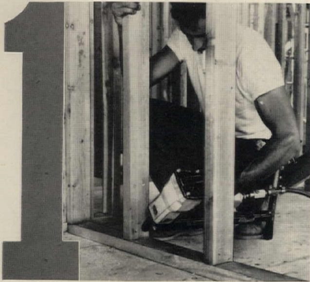
Fast, strong nailing . . . even in close quarters, is easy with a Duo-Fast CN-137 Nailer. The nailer handles coated regular, ring and screw shanks from 6d commons to 16d sinkers. Cohered nail strips are completely interchangeable without changing the nailer.
