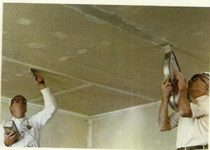
Panelectric panels are factory-wired single-layer 5/8" Fire-Shield Gypsum Wallboard, and can be applied, papered, painted or textured like any other gypsum board ceiling.
