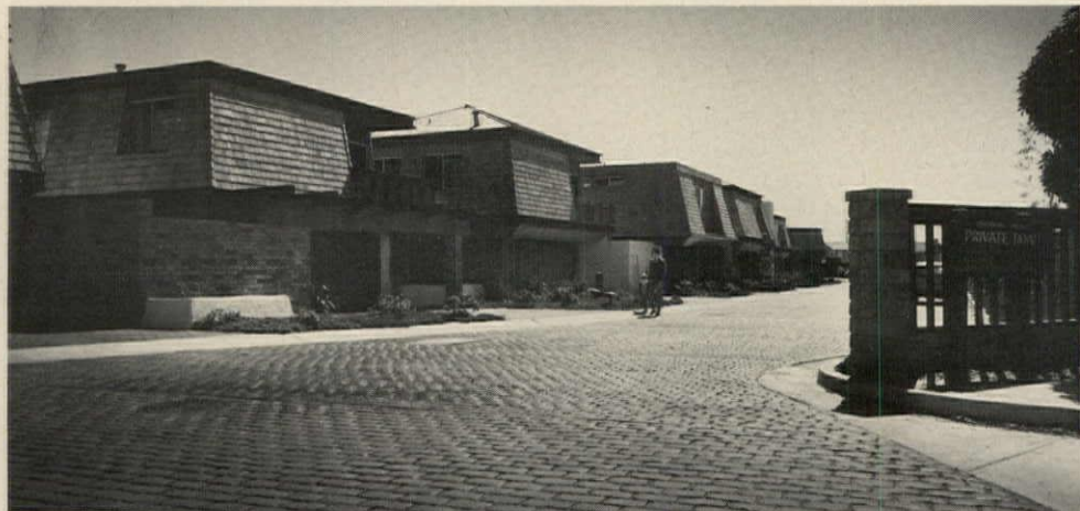
ENTRANCE VIEW shows unity of design in project; units all have same basic shape and wood-shingle finish. Cobblestones were used to pave all walkways and driveways.
