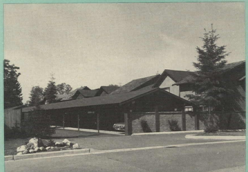
DETACHED CARPORTS behind houses are entered from driveways at perimeter of site. One of two side fences is at left; front wall is at right.
