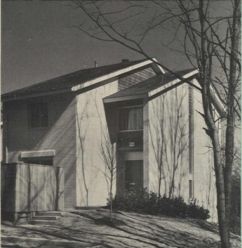
FRONT ENTRY is at middle level of three-bedroom unit (plan, upper right). Fence encloses dining-room patio. High, narrow window in end wall brings daylight into stairwell.
