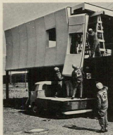
THREE-COMPONENT SYSTEM has wall panels with and without windows (left) and roof panel (right).
