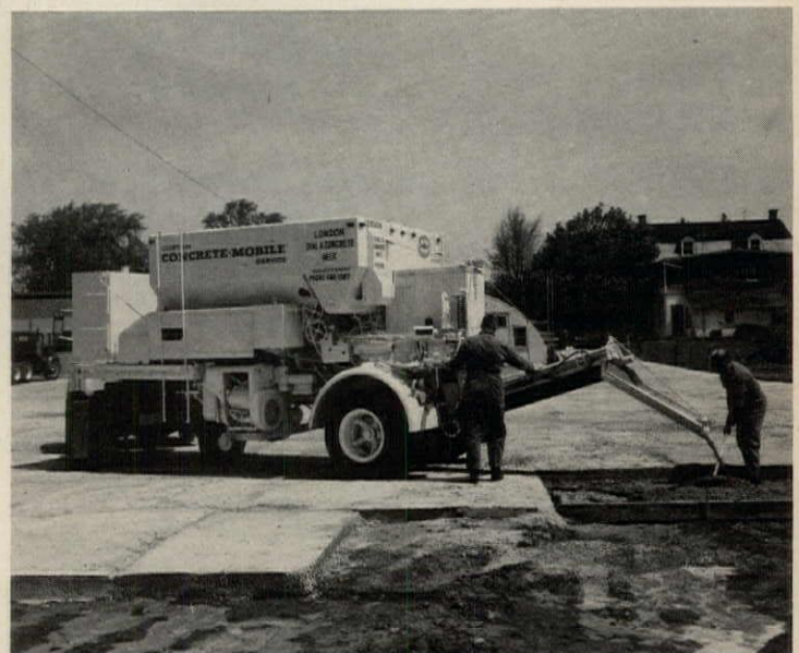
Mobile concrete plant for small jobs produces one cu. yd. in 2 1/2 to 4 min. Operator sets controls so that machine is ready to deliver specified mix on arrival at job site. National Concrete Machinery, Lancaster, Pa. Circle 274 on Reader Service card
