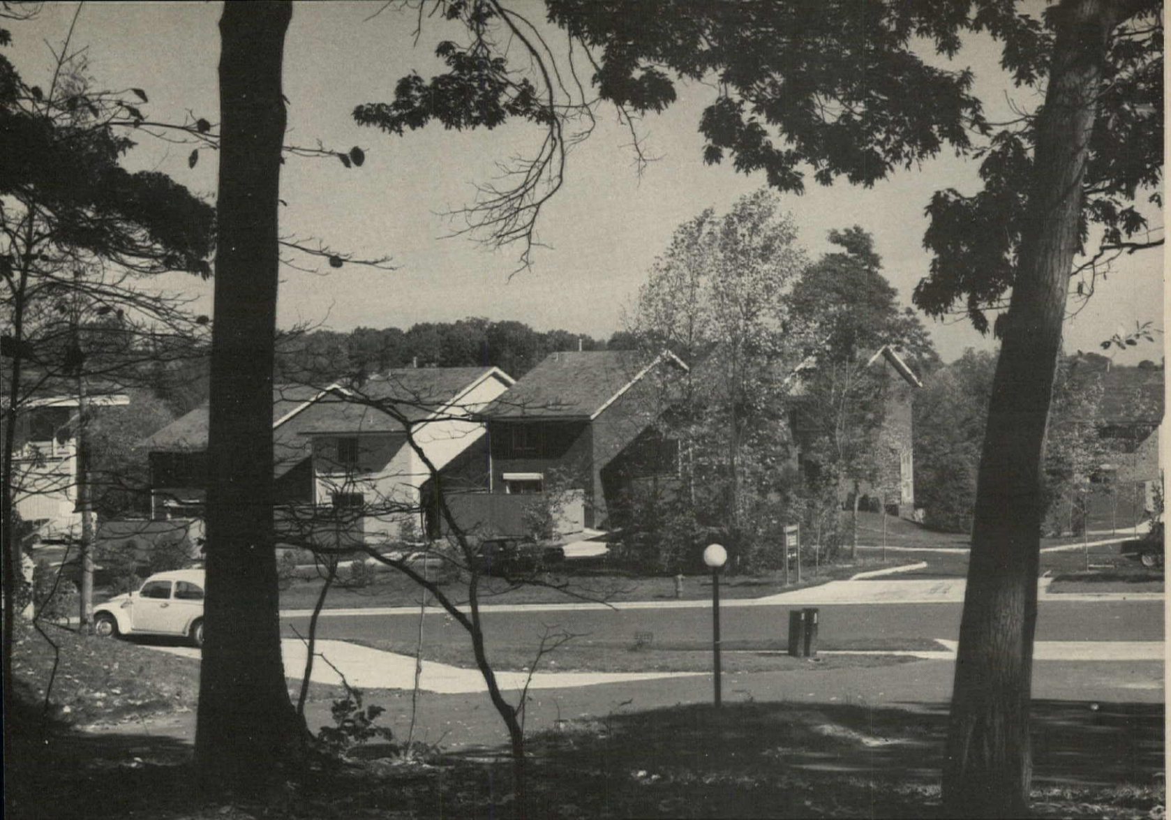
TYPICAL STREETScape at Newmark Commons shows how clustering of houses around courtyards leaves plenty of open space and staggering of setbacks eliminates visual monotony.
