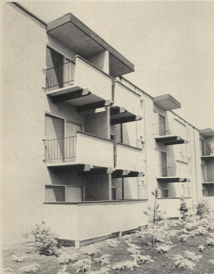
Precast balconies bolt onto extended beams through holes in floor. One-ton units are 7'8" x 4'6". Wood cap on 42"-high railing and wrought-iron side were added by builder. Available in Northwest only. Christy, Fremont, Calif. Circle 256 on Reader Service card
