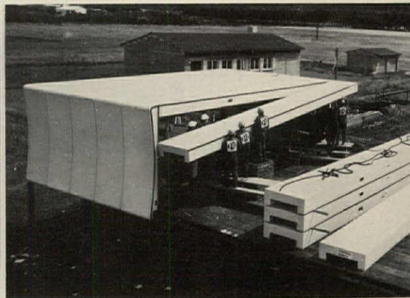
THREE-COMPONENT SYSTEM has wall panels with and without windows (left) and roof panel (right).
