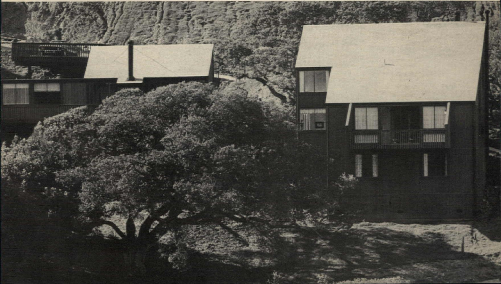
Three-level plan ( left ) puts children's bedrooms and baths on lowest level, main living areas in the middle, master bedroom and study above.
