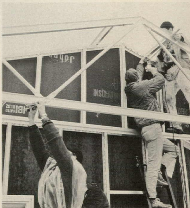
Trusses are tightened with wrench and temporarily braced.
