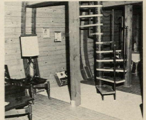
Spiral staircase is easily constructed out of wood. Steel rod in center of wood pole sections acts as support. Exposed t&g planks and double laminated ribs make up interior walls.
