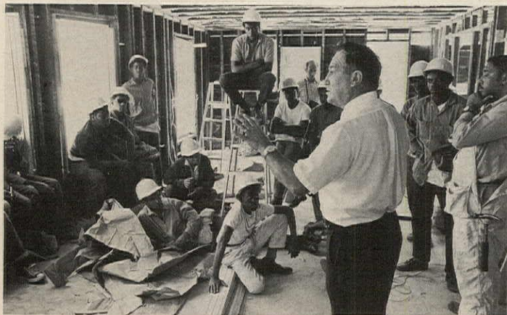
Building Inspector S. G. DeBonis talks to students after approving work.
