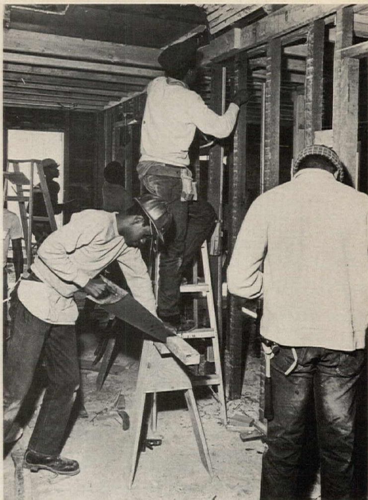
Student carpenters construct partition; they gutted and rebuilt interior.
