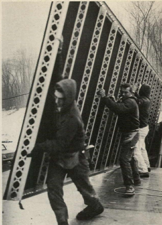
Wall section, easily handled by small crew, is 26' long.
