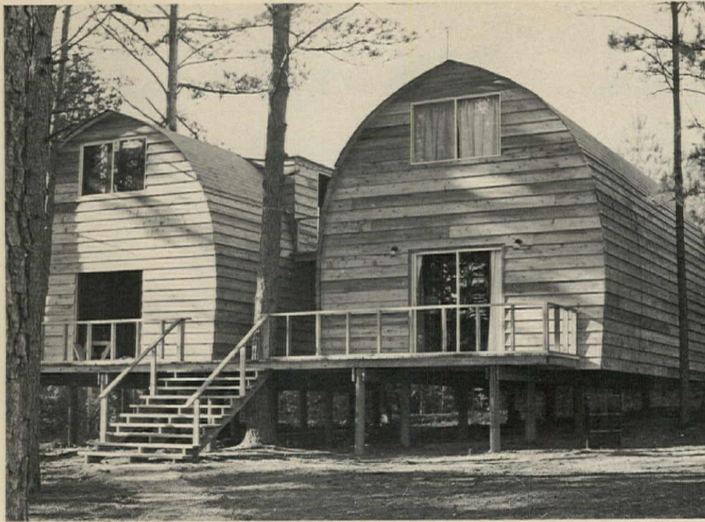
Duplex was built by Charles Doster, Winterville, Ga. Clapboards are nailed to shop-built arches 24" o.c. Alternate exterior has asphalt shingles nailed to plywood. Wallboard covers interior.
