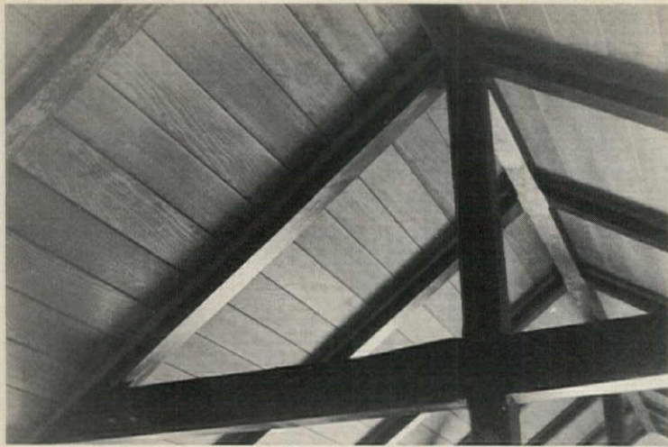
Beamed ceilings retained their original appearance (left), even though a second ceiling (drawing above) was installed in houses soundproofed in Stages 2 and 3.
