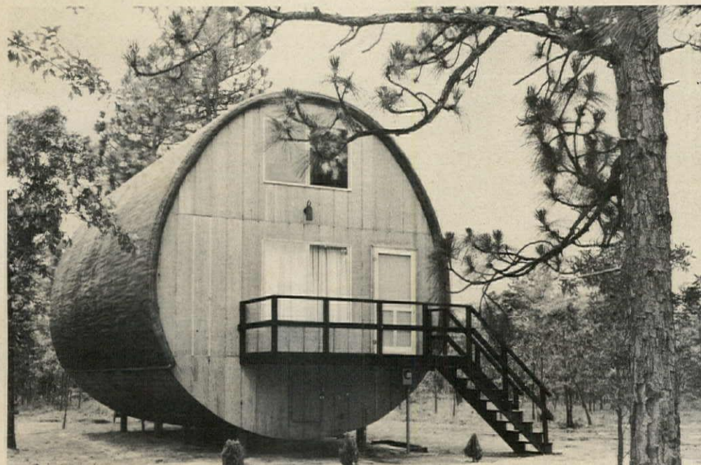
Tubular house was built by Pioneer Homes, Hope Mills, N.C. Built-up roofing and batt insulation were eliminated when foamed-in-place urethane was sprayed over 2x6 t&g planks and then painted.
