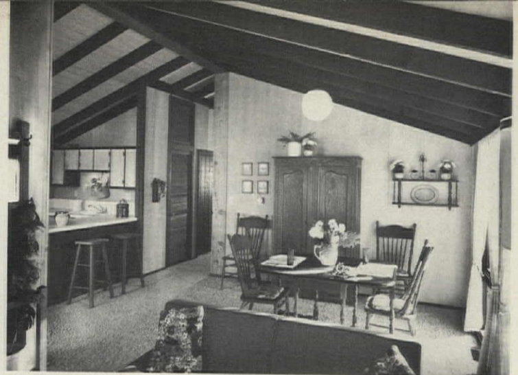
Cathedral ceiling (above) is formed when two shed roof modules are joined at the roof peak. Shown here are the dining area and kitchen of a two-bedroom unit (second from left in plans) with floor-to-ceiling windows in the wall at far right. Walls are prestained fir plywood.
