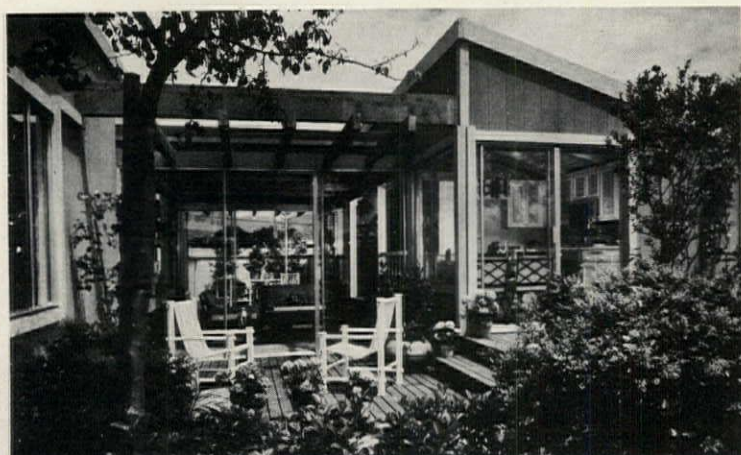
Mobile modulars, joined together by a bridge, form basic Levitt house.
