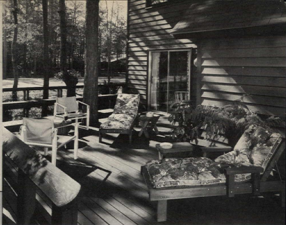
Rear deck (above) opens to living and dining areas (below). Horizontal siding is redwood, treated with preservative; roofing is asphalt.
