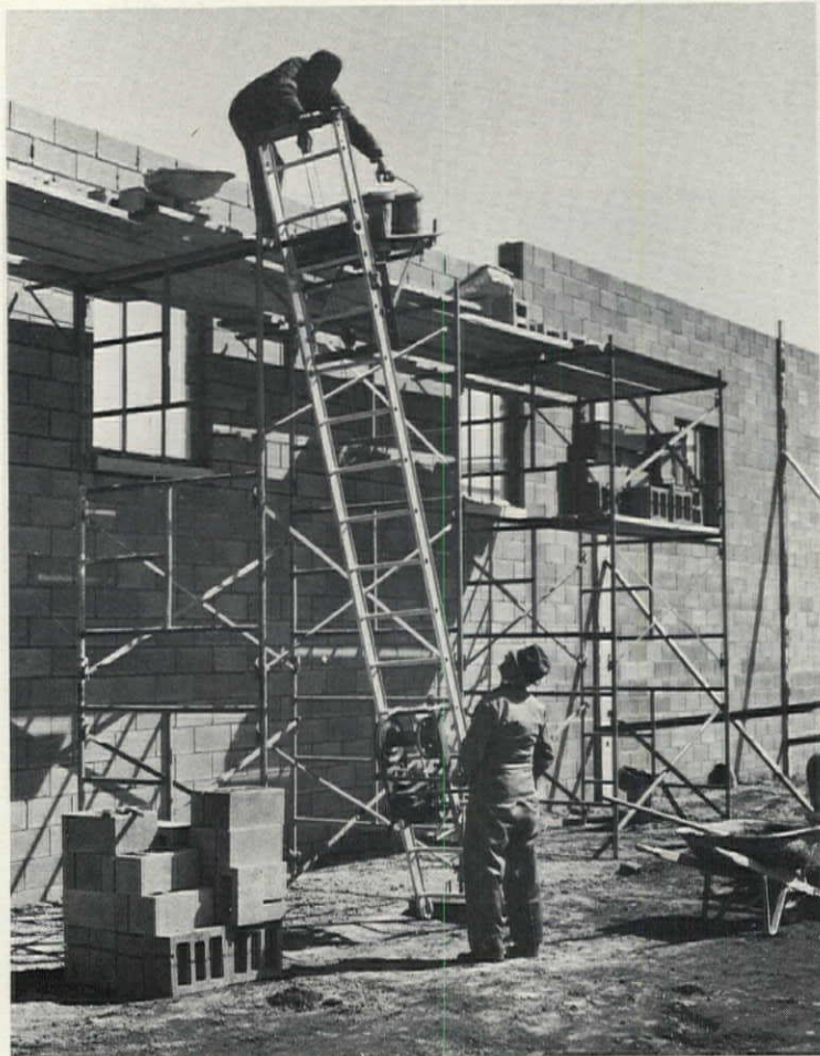
Ladder platform hoist moves construction materials, masonry, panel board, roofing, or appliances up to 44' high. Either gas or electric powered motor. Two sizes—with capacities of 200 or 400 lbs.—are
