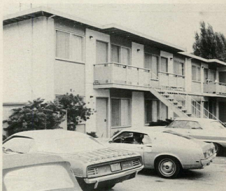
Parking area was the only "scenery" before remodeling, so tenants kept their curtains closed, completely isolating themselves from the outdoors.
