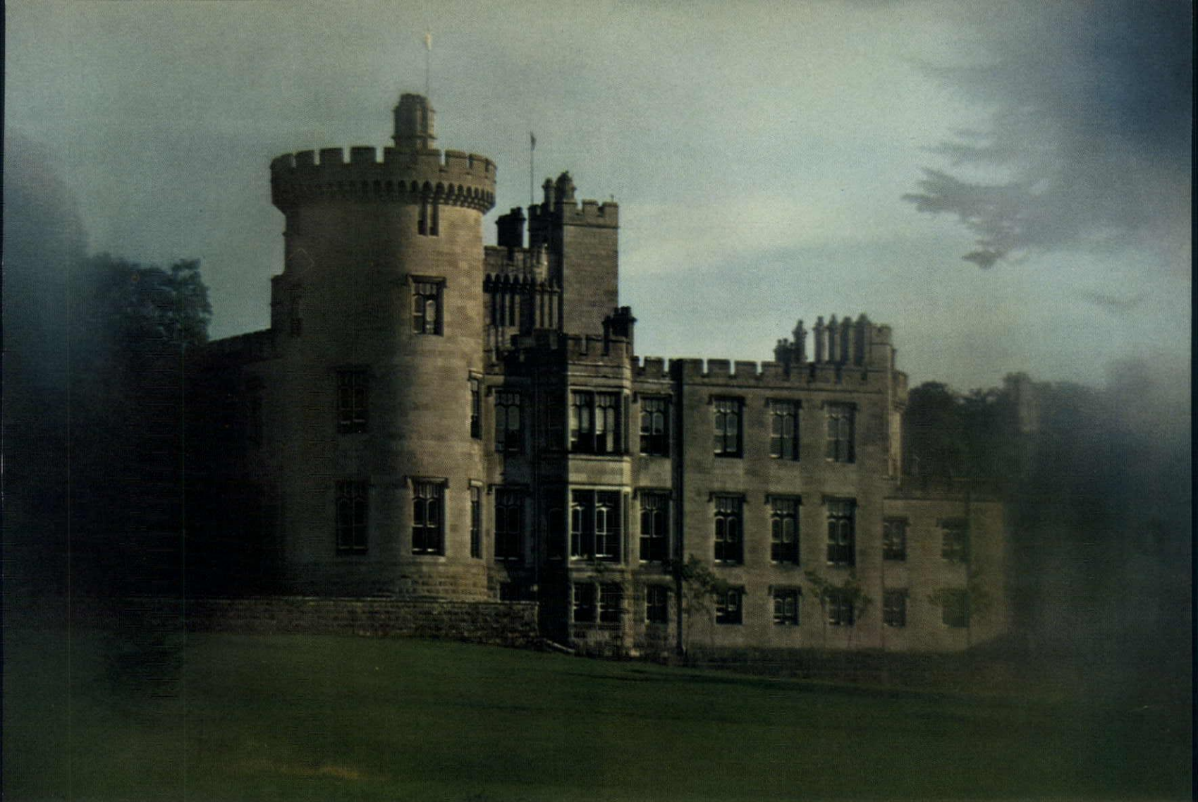
Dromoland Castle, County Clare, Ireland. Built between 1700 and 1800. Remodeled in 1962 by Milosevich and Trautwein, A.I.A.
