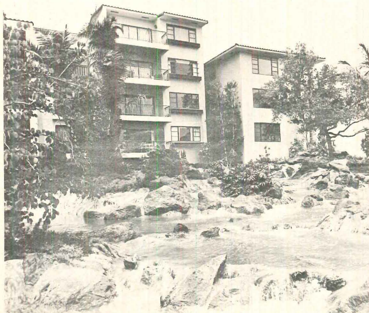
Garden apartments, Falls of Inverrary (Haft-Gaines)
