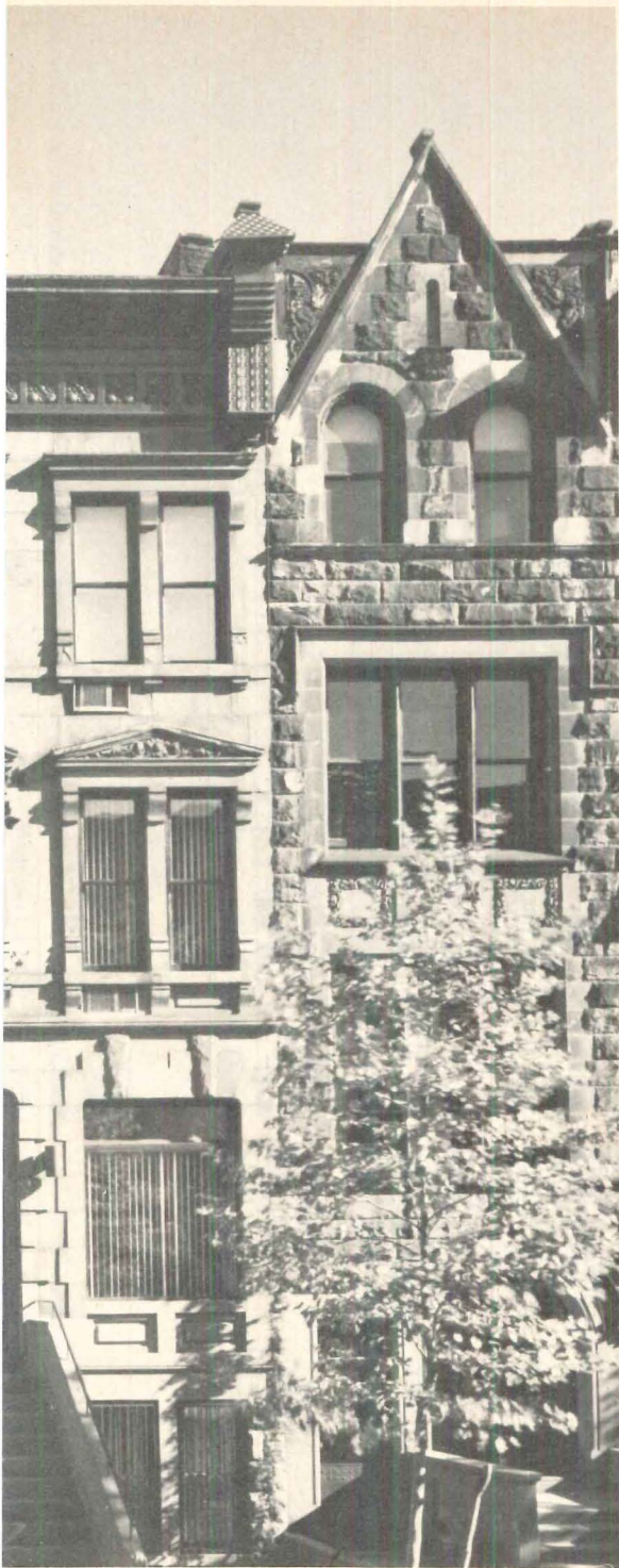
Renovated townhouse (fourth from left in photo above) needed little work on the facade. Major change was the substitution of a large fixed-glass window for two smaller windows similar to those in the adjoining twin houses. Rear elevation (right) was extensively altered. An original extension, which was half the width of the house, was demolished, and the house was squared off with large glass areas and a skylight that illuminates the interior with reflected northern light.
