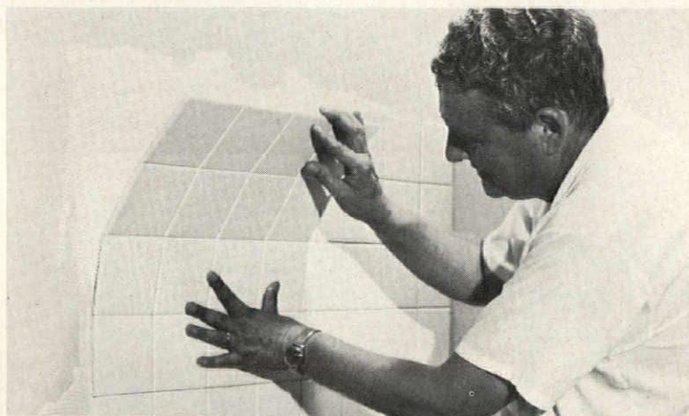
Pre-mounted tile sheets designed for fast, easy installation contain sixteen 4 3/8" square tiles. Up to 2 sq. ft. of tile can be set at once. Sheets with perfectly aligned tiles and joints can be cut to fit. "Set-N-Go" is applied
