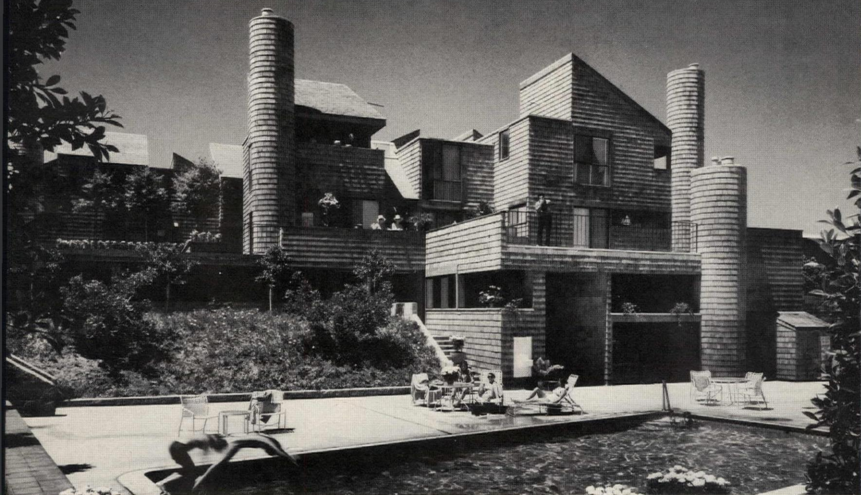
Seascape I, Solana Beach, California. Roots: Certigrade shingles No. 1 Grade, 24" Royals. Walls: Certigrade shingles No. 1 Grade, 16" Fivex. Architects: Oxley & Landau. Builder: Westward Construction Corp.
