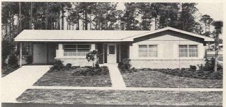
Generation III: Concrete floors allow modular home to be built at grade.
