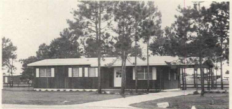
Generation II: Wood floors required air space between ground and floor.
