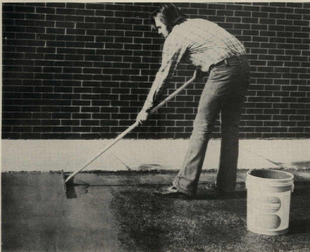
"Sandstrom TUF-TRAC" adds color while protecting asphalt surfaces. Offered in seven colors, sealer is non-fading, non-chalking and non-staining. Substance, with a slight texture for safe traction, fills hairline cracks and other small voids in pavement. Premixed sealer is quick-drying and thermal-resistant. Glenrock, Northlake, Ill. CIRCLE 247 ON READER SERVICE CARD
