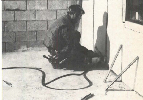
Interior wall insulation system, Zonolite® Thermo-Stud® (above), is used on masonry walls. The system is a rigid styrene foam insulation board in which a U-shaped metal furring channel is imbedded (see insert). Power-driven fasteners secure system. Grace, Cambridge, MA. Circle 252 on reader service card
