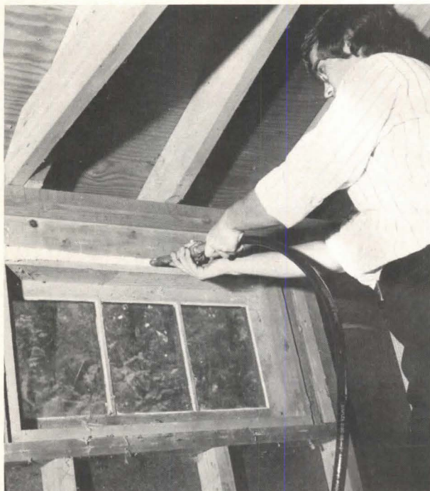
One-component urethane foam (above) serves as an insulating filler between a window and framing. Self-curing material expands to two to three times its original volume, filling nearby space as it sets to a flexible or semi-rigid form. Rubicon, Geismar, LA. Circle 249 on reader service card
