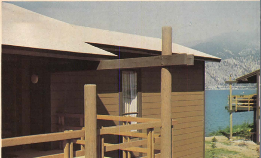
Washington Condominiums, Howard S. Wright Construction Co.
