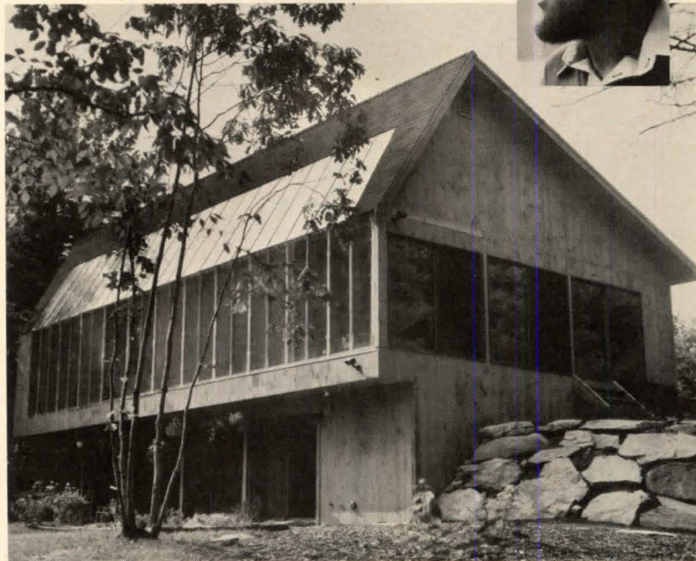
Solar house designed by Robert Parkin (inset) assures free flow of heat by reducing first-level partitions (plan left) and opening space to second level. Collectors span pitched portion of roof (above), and the vertical panels immediately below.
