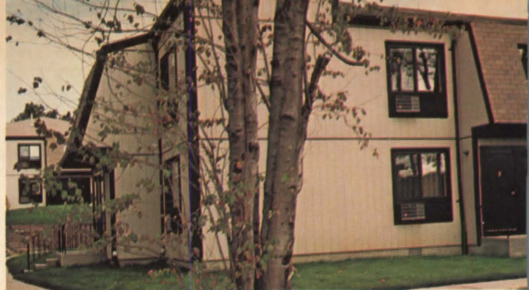
New York Apartments, Mar-Jef Construction Co.
