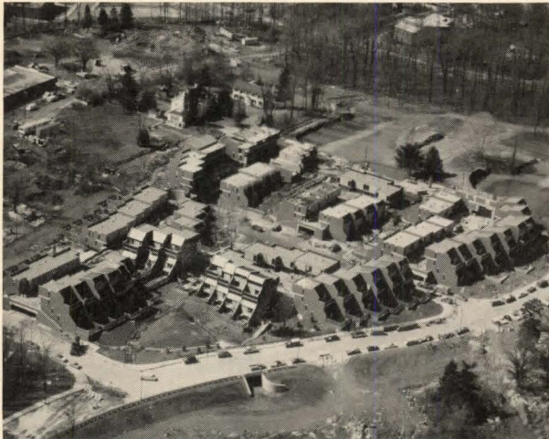
First phase of Baltimore's in-city housing project is cluster of 124 townhouses. Modernistic condo units (shown at right are front and rear views) use conventional building features such as masonry-bearing walls, precast concrete floor system and all-wood roofs to hold down construction costs.
