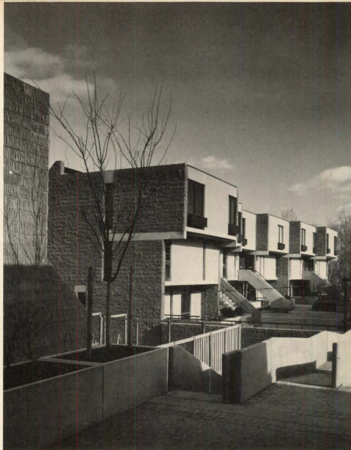
First phase of Baltimore's in-city housing project is cluster of 124 townhouses. Modernistic condo units (shown at right are front and rear views) use conventional building features such as masonry-bearing walls, precast concrete floor system and all-wood roofs to hold down construction costs.
