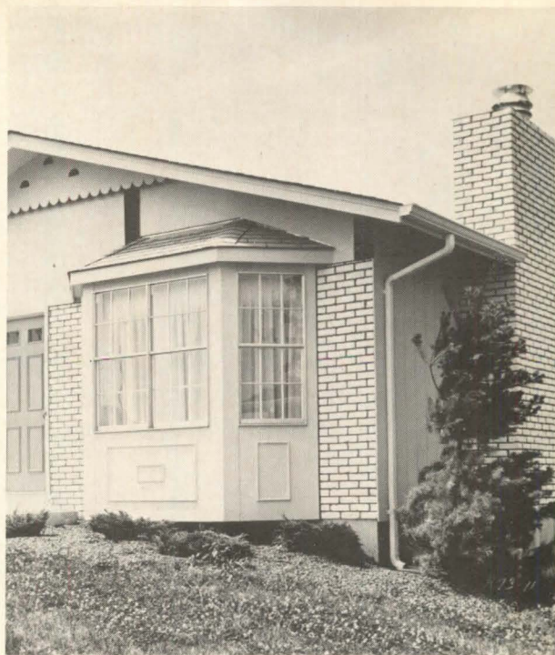
Premortared panels (above) are made from crushed stone reinforced with fiber glass. Interlocking brick-simulated panels are available in four tones. Marlite, Dover, OH. Circle 202 on reader service card
