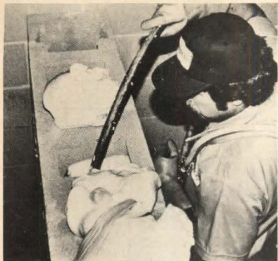
Insulspray® (left) is a urea-formaldehyde-based foam insulation. Foam may be pumped into concrete or cinder block cavities (shown), or into sidewall cavities in existing homes. Borden, Columbus, OH. Circle 224 on reader service card
