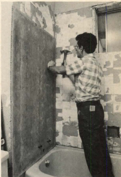
Backer-board (above) is used for ceramic tile and floor installation. The 1/2"-thick board, made of concrete reinforced with fiber glass, comes in sizes of 36" x 48", 36" x 60", 36" x 64" and 36" x 72". American Olean, Lansdale, PA. Circle 230 on reader service card
