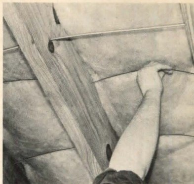
Insulspray® (left) is a urea-formaldehyde-based foam insulation. Foam may be pumped into concrete or cinder block cavities (shown), or into sidewall cavities in existing homes. Borden, Columbus, OH. Circle 224 on reader service card
