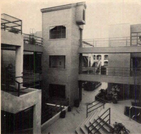
10. Glendale, Calif.; Architect: Collins & Wraight Developer & Builder: Richelieu Development; G.M. Tobian Construction Co.
