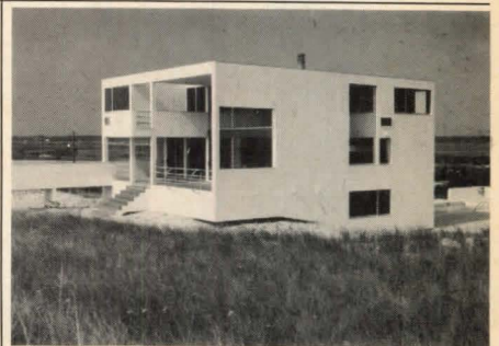
19. Quogue, N.Y. Architect: Gwathmey Siegel Architects Builder: Harold Reeve & Sons Inc.
