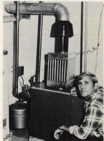
"Flue radiator" replaces section of boiler flue pipe, as shown above. According to the manufacturer, the unit recovers approximately 40% of the heat normally lost up a chimney. Stoneberg. Circle 241 on reader service card
