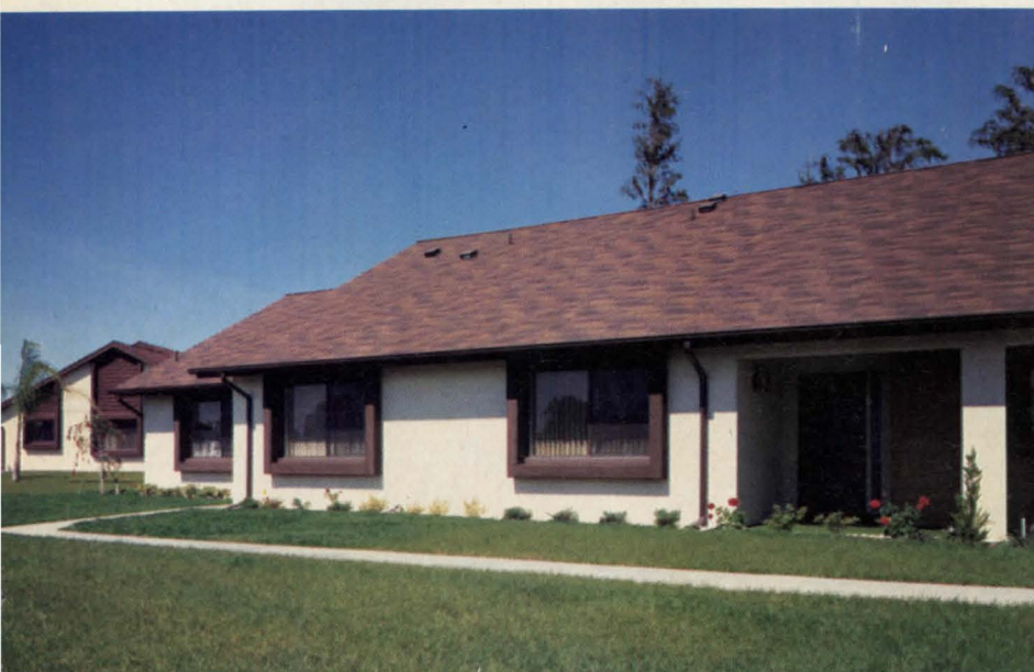
Village on the Green, Clearwater, Florida. Frank Macagnone, Division President. U.S. Home Corporation
