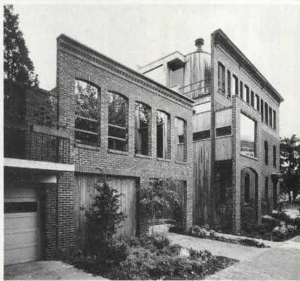
10. Washington, D.C. Architect: Kerns Group Architects, P.C. Builder: The Lenkin Co.
