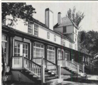
17. Glenbrook, Nev. Architect: Backen Arrigoni & Ross Inc. Builder: Squaw/Wynn Construction Co.
