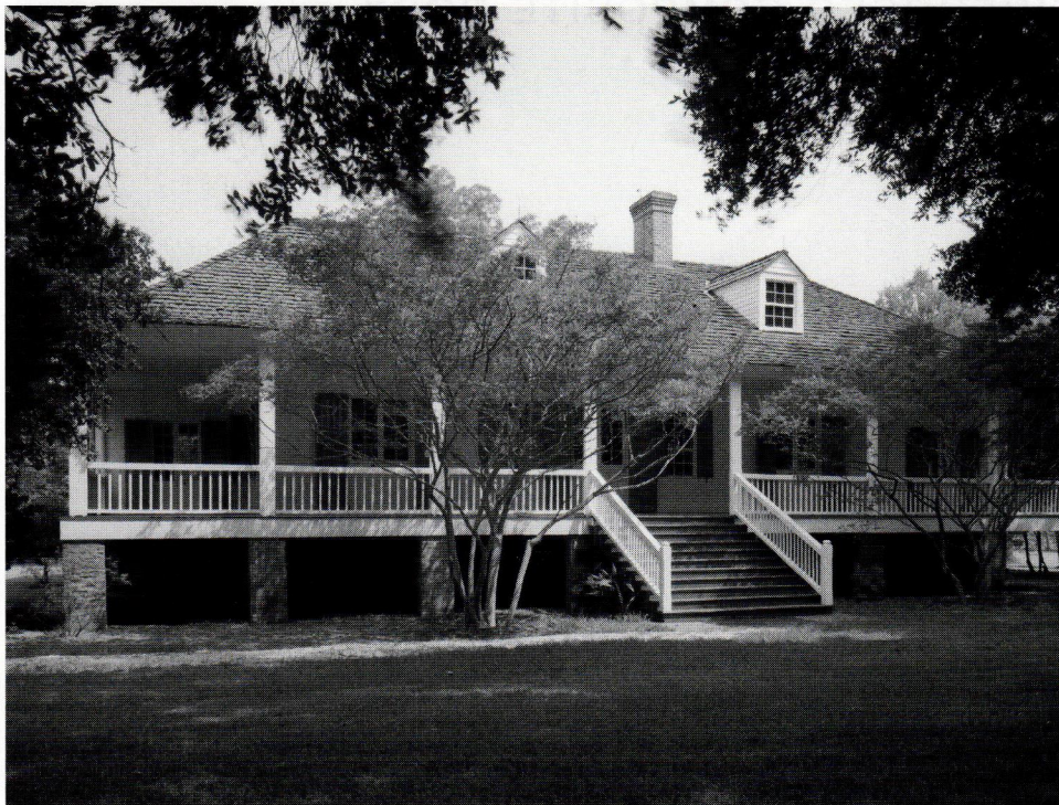
Magnolia Mound in Baton Rouge, Louisiana, built in the 1790s, offers a deep front porch and several doors and windows for cross ventilation during the region's hot summers.
