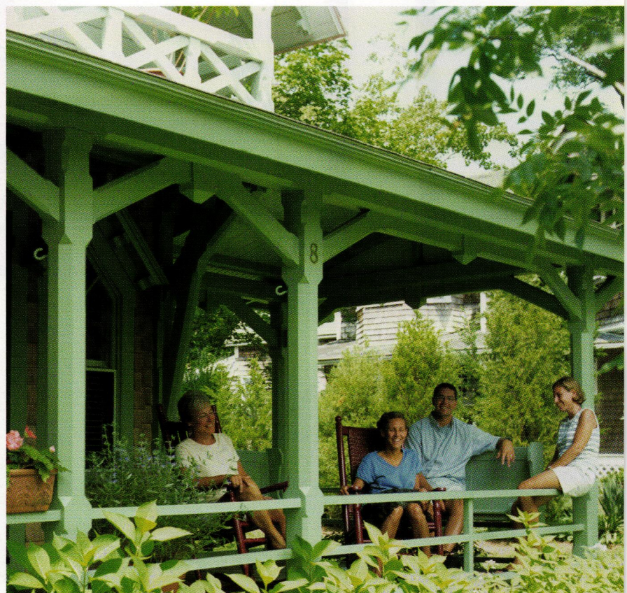
These romantic modified Gothic Revival cottages in Oak Bluffs on Martha's Vineyard have been jointly renovated for use by a growing family and creatively united by a common courtyard. A front view of the exterior restoration highlights their harmonious profiles while celebrating the architectural differences found in the gable, truss, porch post, bracket, and railing details. The Blue cottage on the left is limited to summer use, while the Green cottage on the right is winterized. Above right White cedar shingles appear in contrasting random and diamond-shaped patterns. A decorative window hood deflects rain away from the Gothic-arched window. Below right Homeowner Sharon Robinson, daughter Bre, son-in-law Janszen, and daughter Erin relax on the front porch of the Green cottage.
