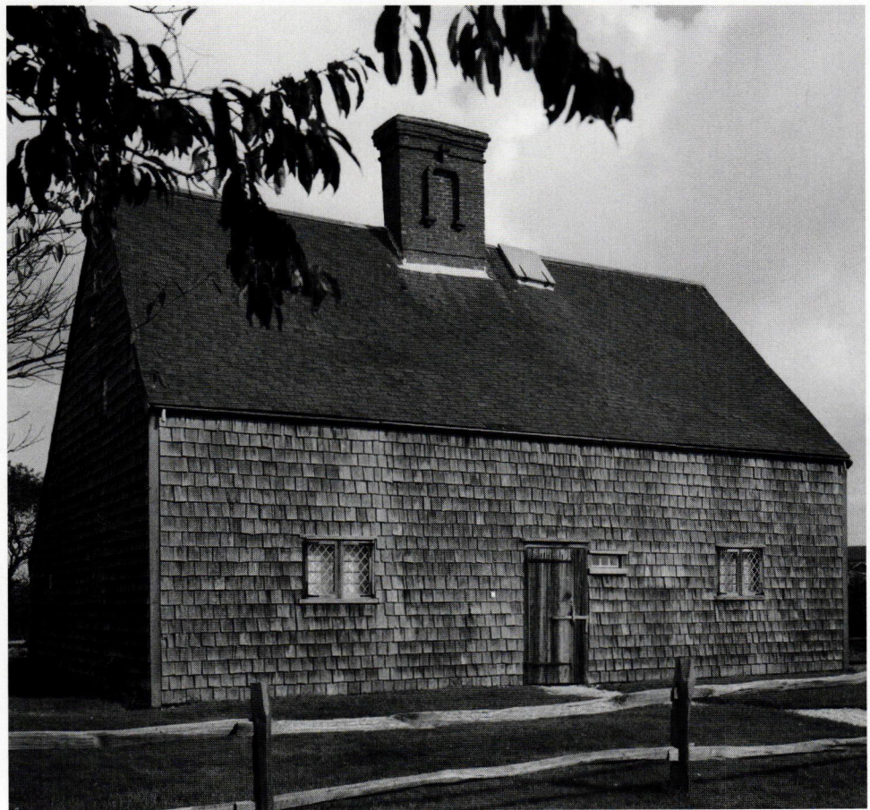
HISTORIC AMERICAN BUILDINGS SURVEY JACK E. BOUCHER, PHOTOGRAPHER
