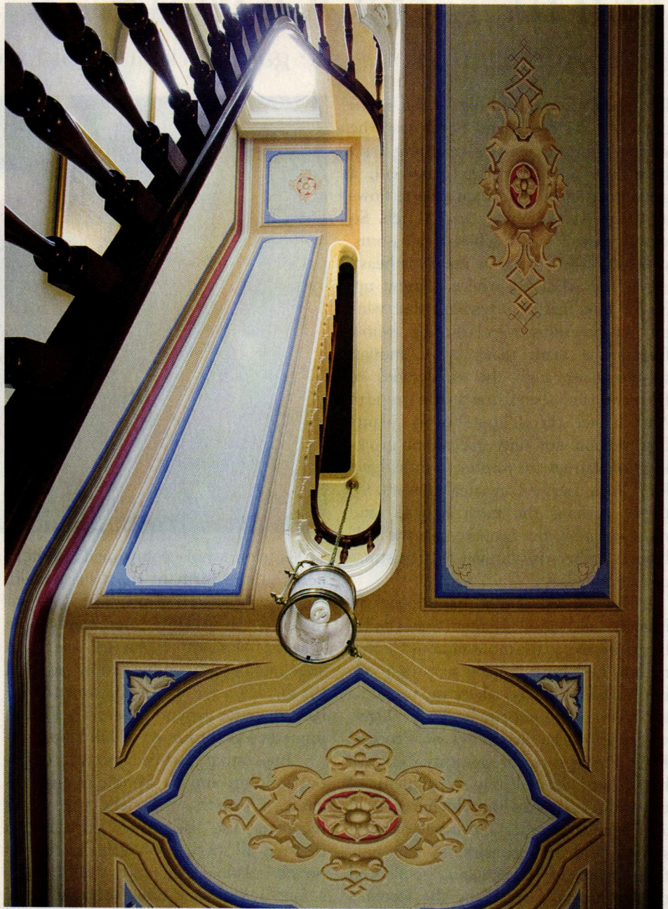
Castro often works with stencilling to recreate designs that have been lost.
