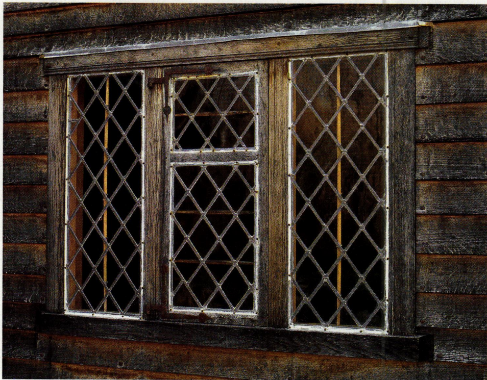
Maurer and Shepherd Joyners makes historically accurate windows, such as this seventeenth-century lattice window with diamond panes.
