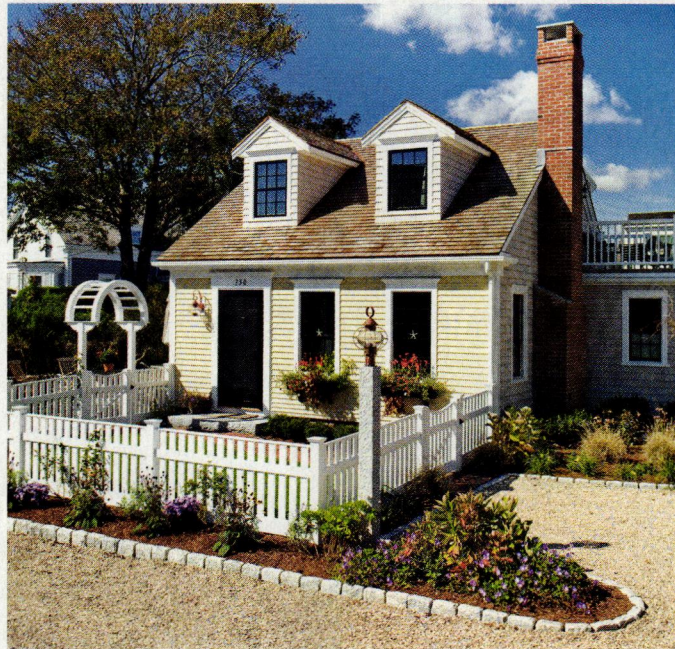
Rick Roy Construction built this 900-square-foot house on Cape Cod using the basic principles of building lean.
