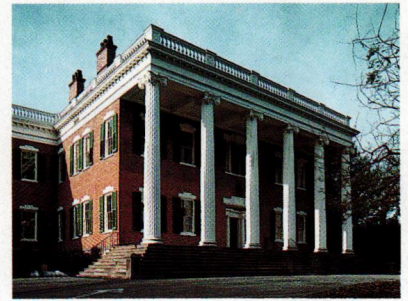
Drew University's Mead Hall suffered disastrous fire damage. Massey-Maxwell Associates provided the historical basis for its rehabilitation and restoration.
